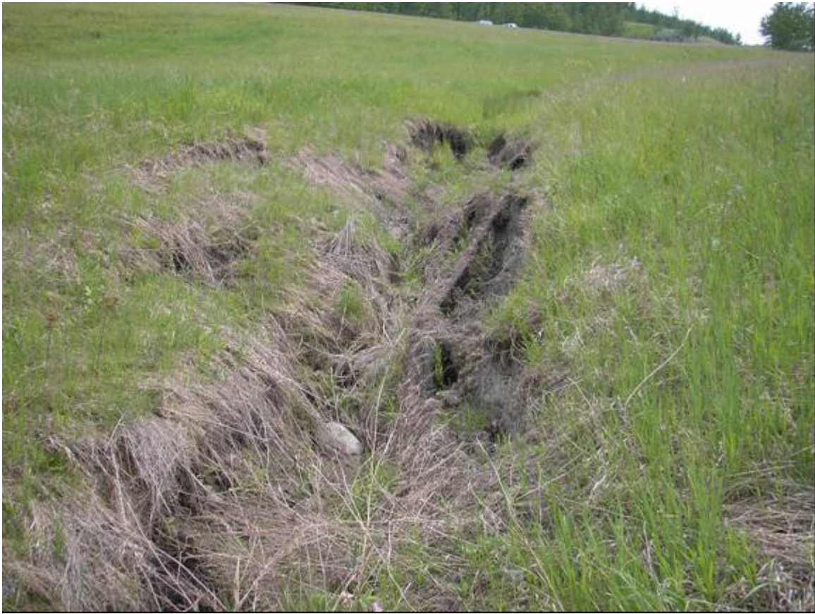
Photo 2 - Looking southwest at erosion gully.
