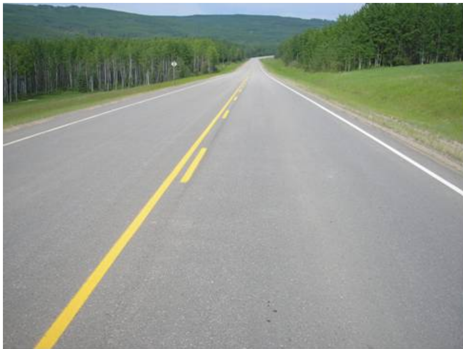
Photo 5 - Northeast view along highway at Site # 2.
