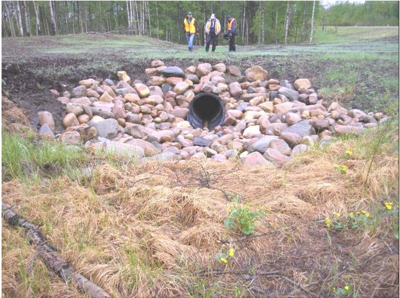
Photo 2 - Looking north at culvert inlet, May 24, 2006.
