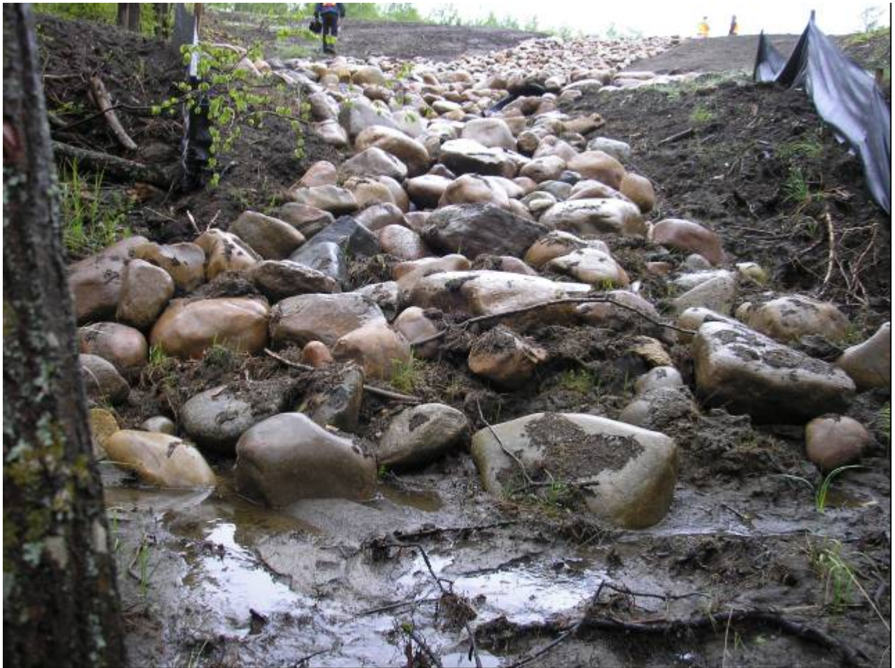
Photo 3 - Looking south at culvert outlet, May 24, 2006.
