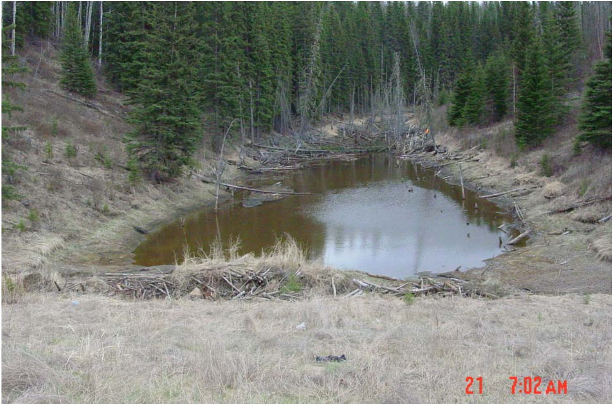
Photo 1: View of south sideslope, beaver dam remains with ponded water south of culvert inlet.
