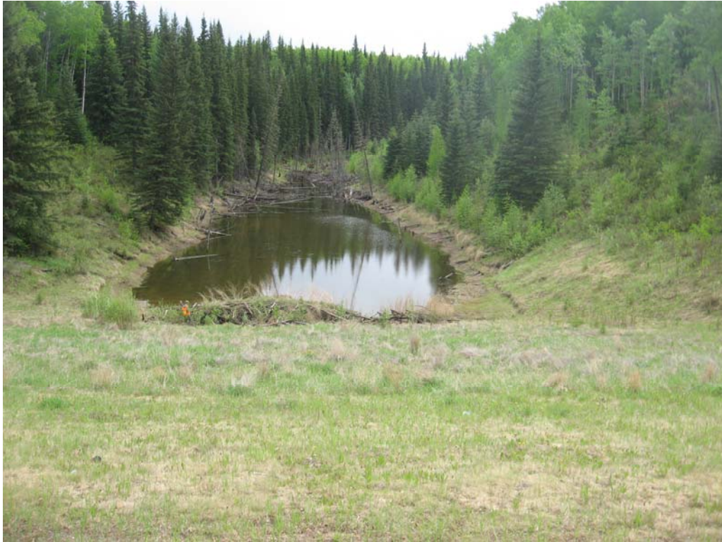
Photo 1: View of south sideslope, beaver dam remains and ponded water, south of culvert inlet.
