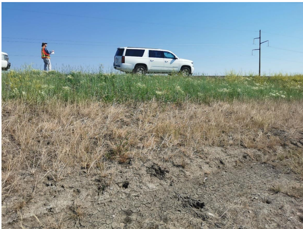
Photo 2 – Looking northeast at south slope of highway embankment from south ditch.
