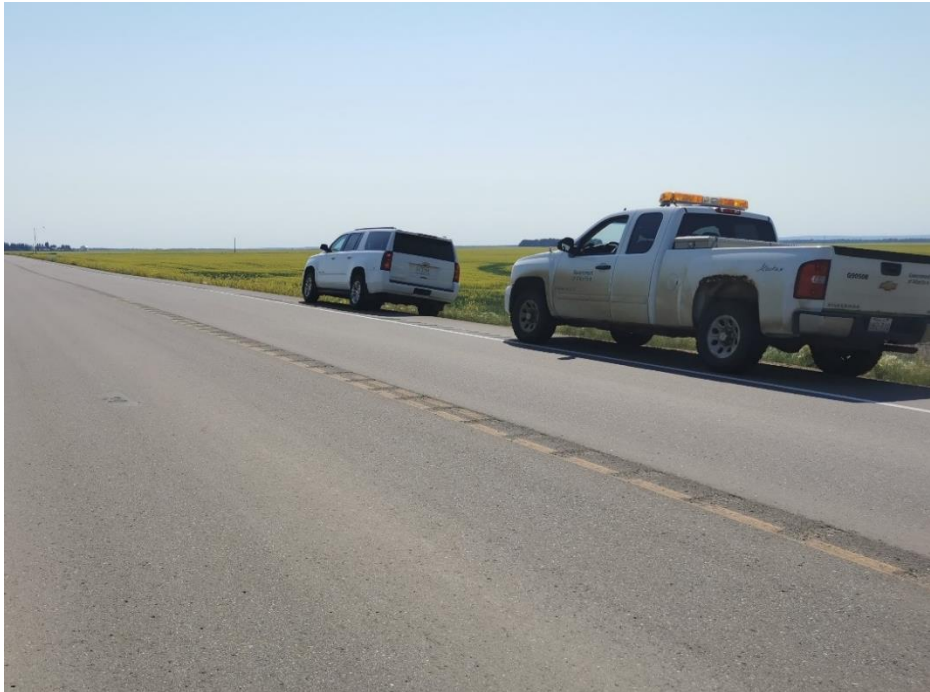
Photo 1 – Looking east from west end of newly-reconstructed portion of EBL.
