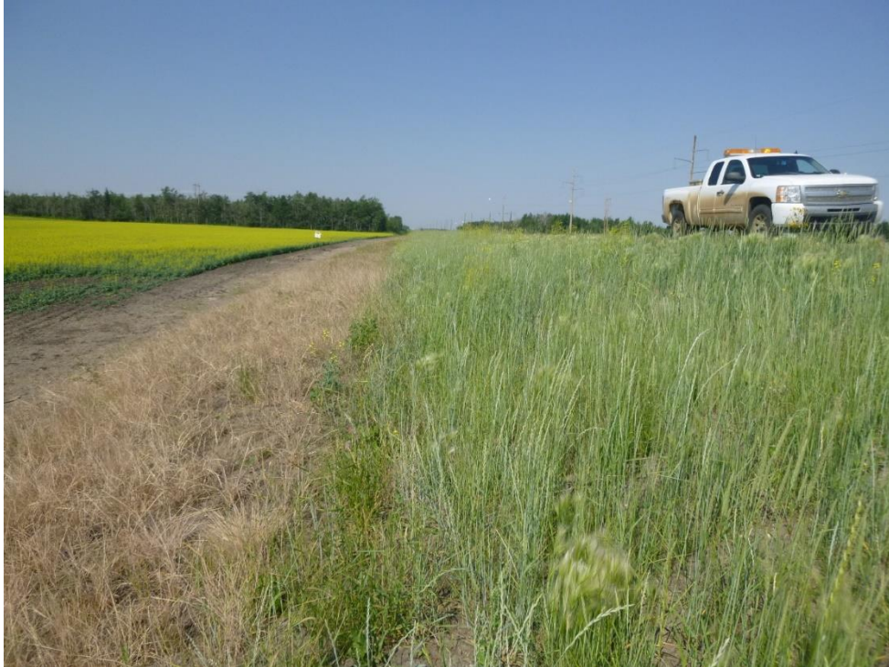
Photo 3 – Looking west along south side slope of highway embankment.
