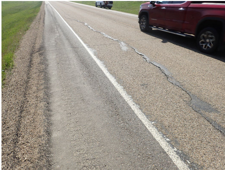
Photo 2 – Looking east along the WBL at longitudinal cracks that extends west from the main landslide crack.
