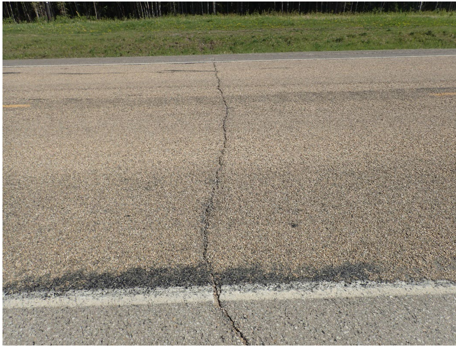
Photo 1 – Looking north at transverse crack that crosses the main landslide’s head scarp crack and highway dip.
