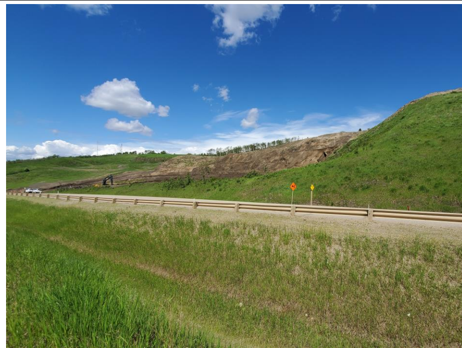
Photo 59-02. Looking northwest towards the slope above the highway that was excavated for borrow fill for other highway work (35+000).
