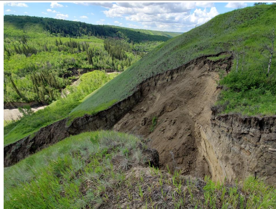
Photo 59-05. Looking downslope at head of the widest segment of an erosion gully approximately 125 m downslope (south) from the highway (35+450).
