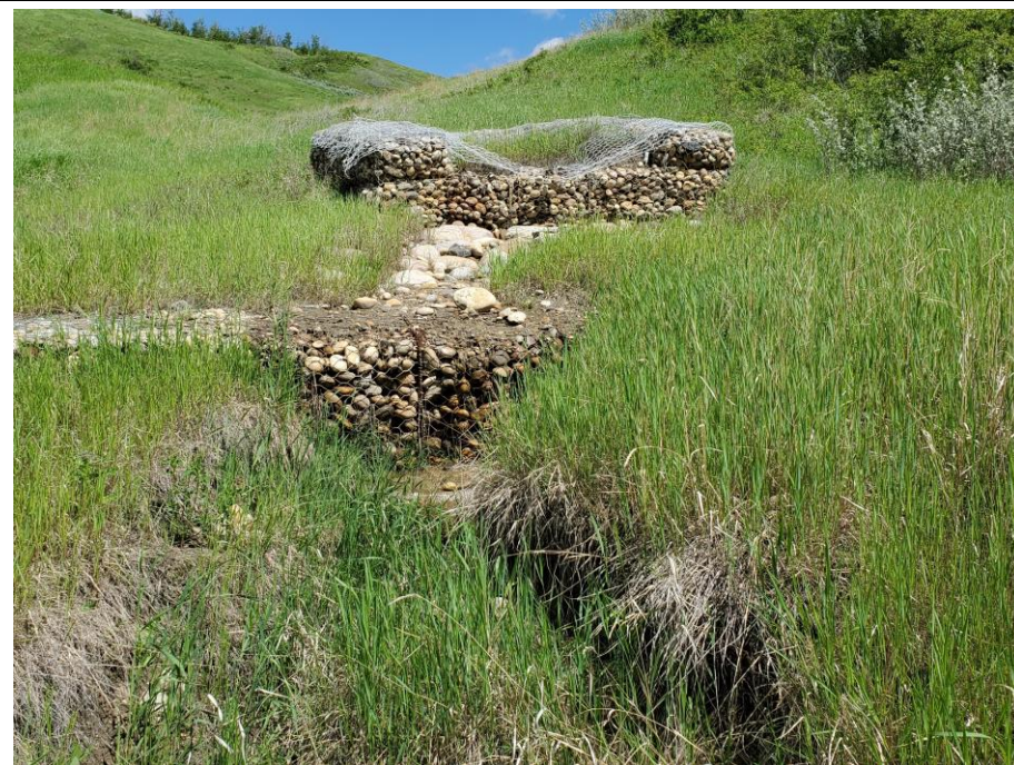
Photo 59-07. Gabion culvert outlet structure (35+500) appears in similar condition to previous inspections.
