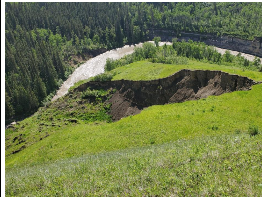
Photo 60-04. View overlooking the main scarp of a major slide/earth flow event that occurred in 2016. Minor retrogression since that time. Slide area is offset approximately 180 m from the highway (35+950).
