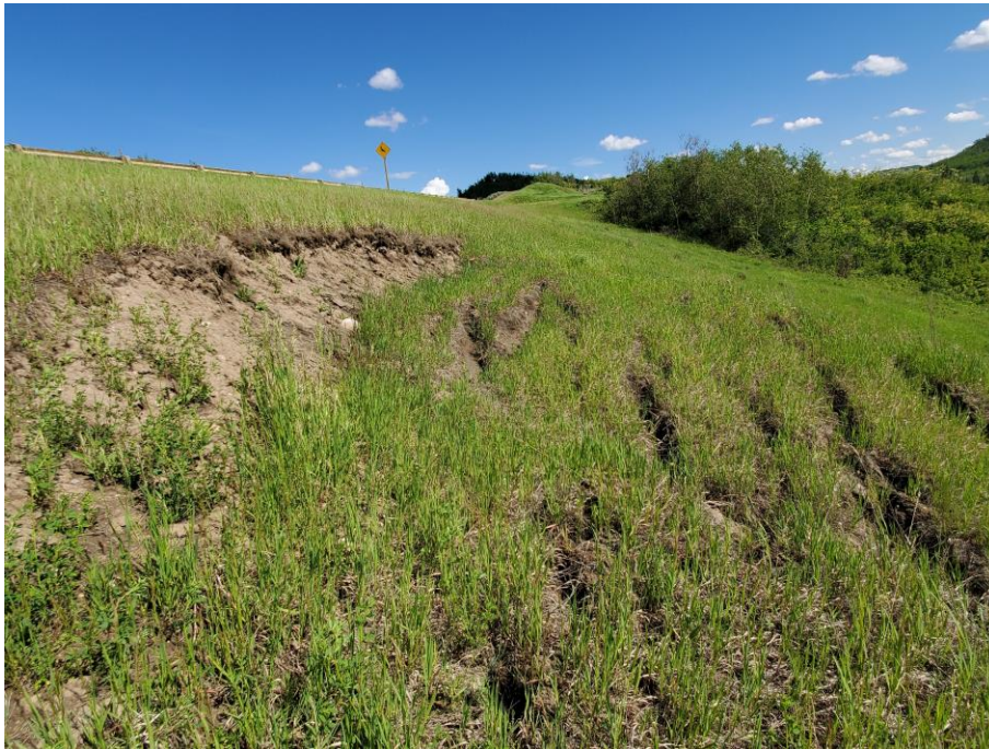
Photo 61-01. Looking east towards the shallow slide scarp approximately 10 m below the highway (36+350). No major change since 2019.
