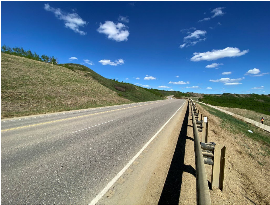
Photo 70-07. View along highway looking east above pile wall. No pavement disturbance was visible since the Fall 2022 repaving.
