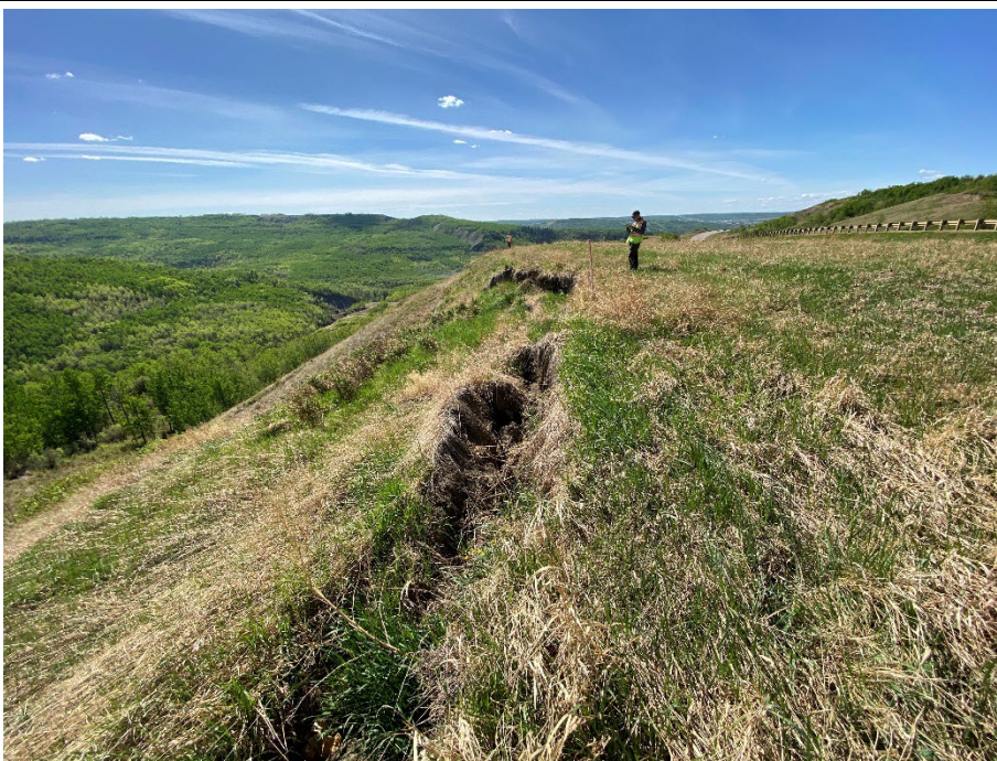
Photo 70-09. Looking west from the east end of the active landslide scarp developing west of the pile wall (34+050). There was a more visible scarp with increased dropdown (up to 1.6 m in height) and the tension cracks have extended and opened up further relative to the 2024 condition.
