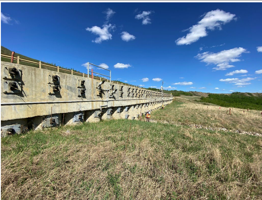
Photo 70-03. Looking east near the centre of the retaining wall with Class 1 riprap swale located near 33+950. East flank of the 2016 slide is visible in the background. SI13-3 is visible on the right side of the photo. No major changes were visible on the bench below the wall since 2024.
