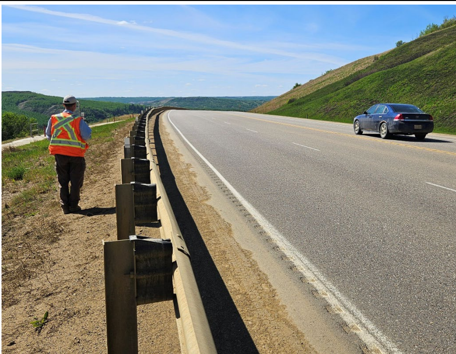
Photo 70-08. Looking west along highway above pile wall. Visible dip in guardrail (near 33+900) suspected from install and likely not related to slide related settlement that occurred prior to the pile wall. No cracking or other slide related distress was visible in pavement along previous damage extents since the highway was repaved in 2022.
