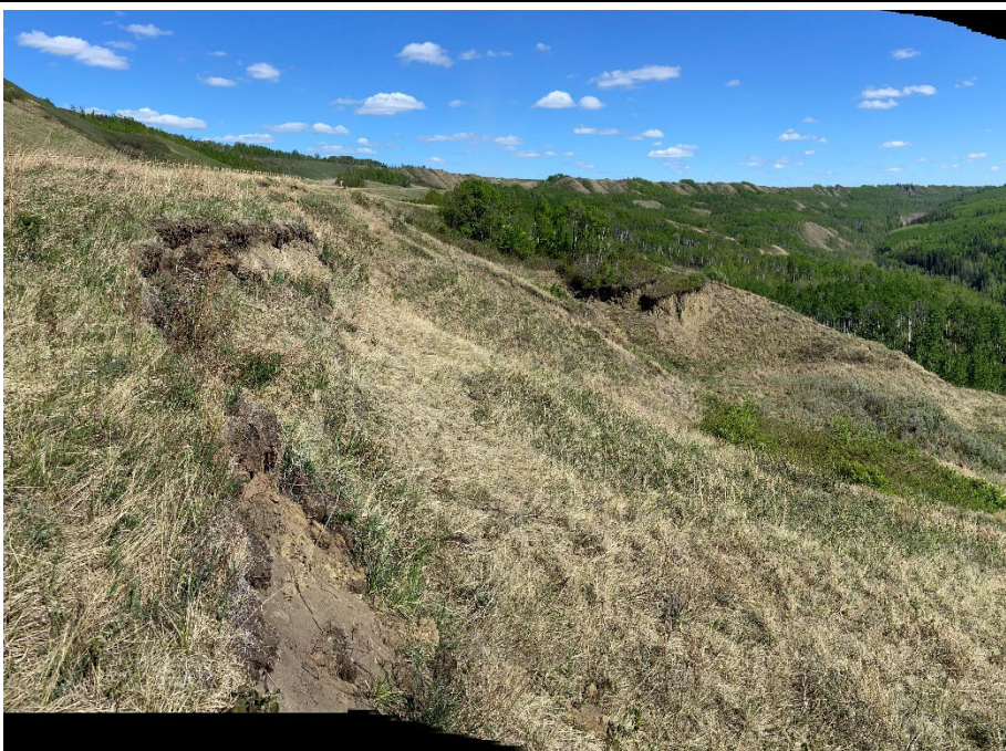
Photo 70-10. Looking east at main scarp expansion west of the pile wall near 34+100 with increased movement since 2024. Dropdown of the scarp in this area was up to 1.5 m in height. Increased dropdown and lateral expansion along previously observed tension cracks. Minor retrogression towards the highway was measured at the survey stakes. Lower slide terrain has ongoing movement but no major visible changes.
