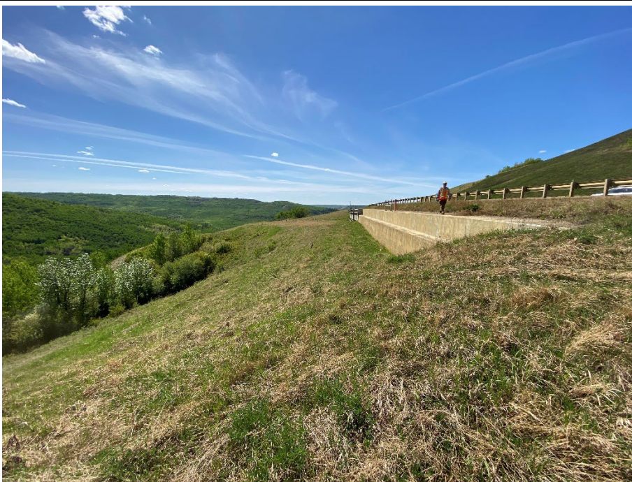
Photo 70-01. Looking west at concrete pile retaining wall at 33+850. No major visible changes downslope from the wall since 2024.
