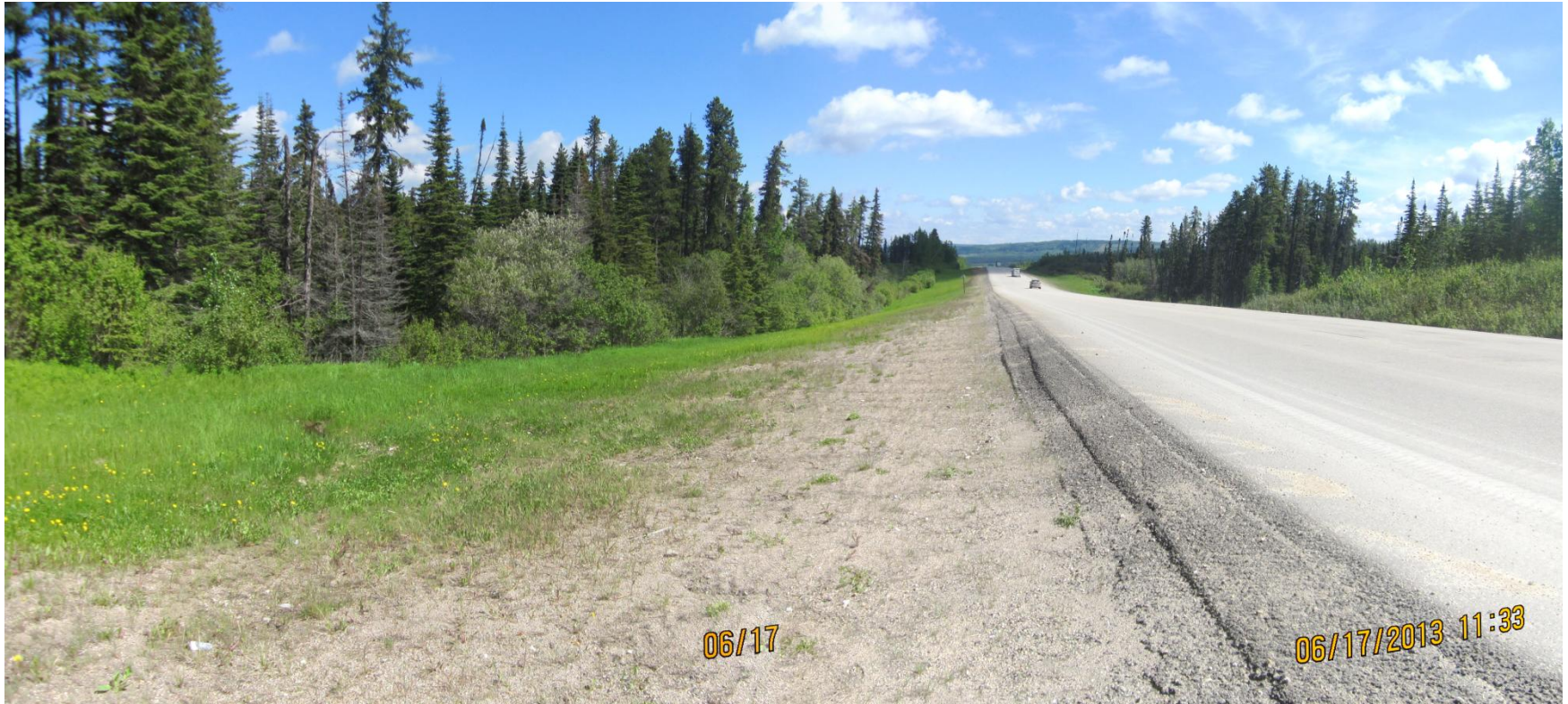
Photo 2: Looking north east along downslope side of highway embankment.
