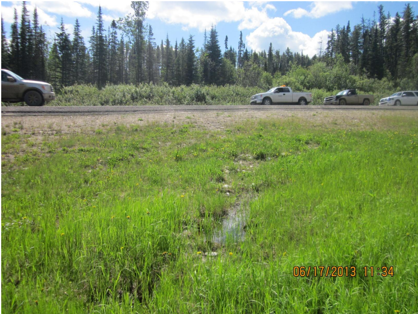
Photo 3: Looking south. Wet area of downslope ditch
