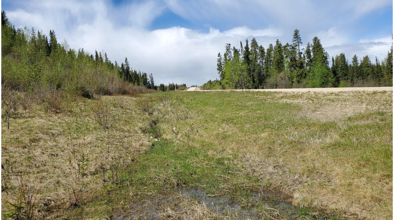
Photo 5 – Looking south at erosion in east ditch.
