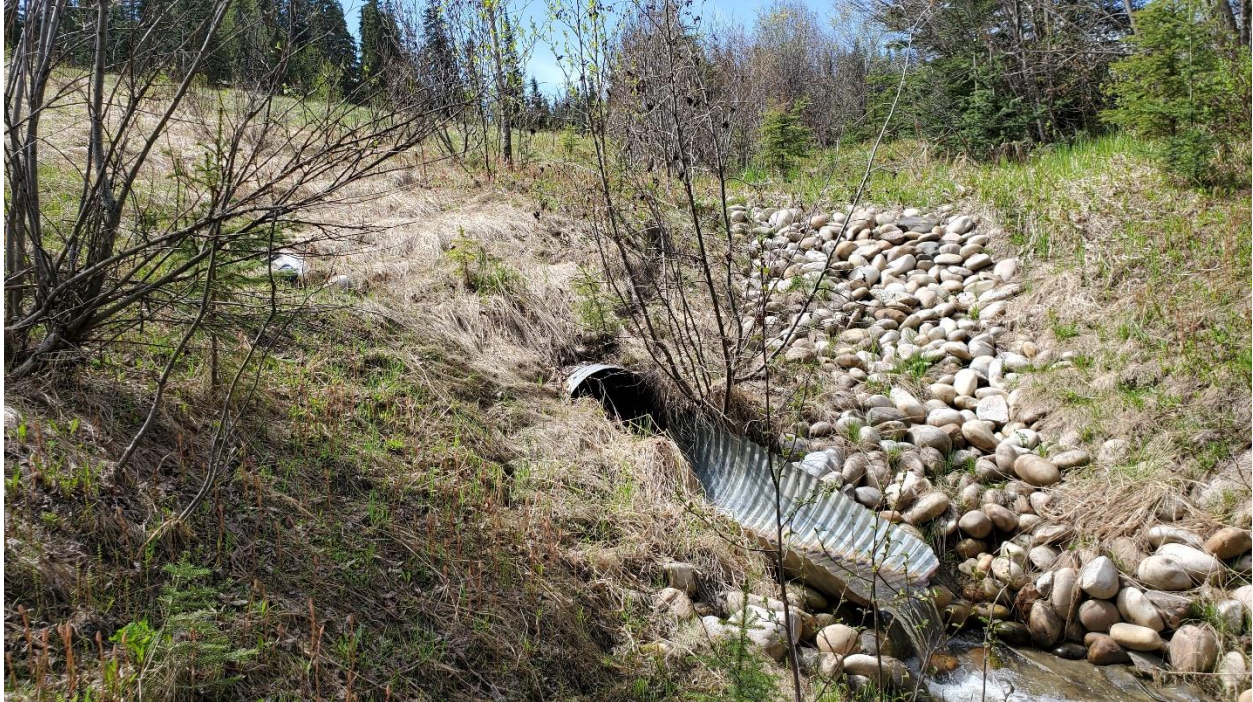
Photo 11 – 920 mm dia. centreline culvert outlet.
