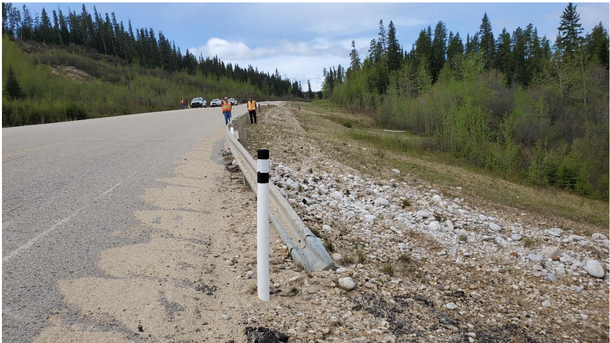
Photo 6 – Looking south at cobbles placed in gully at north end of guardrail.
