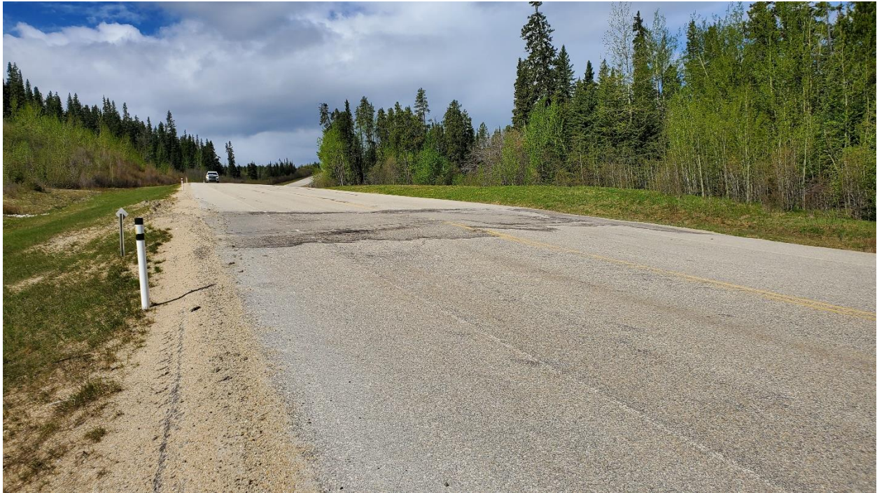
Photo 1 – Looking southwest at patch over cracks forming at the southwest end of the wall.
