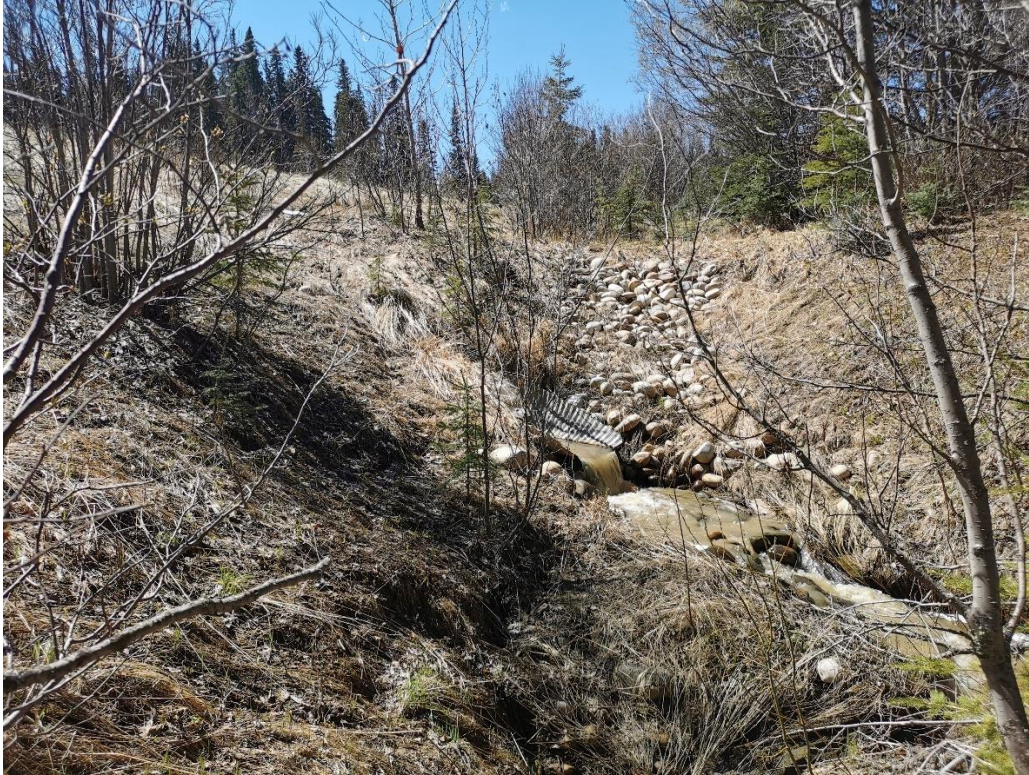
Photo 11, SH001-1 – 920 mm dia. centreline culvert outlet.
