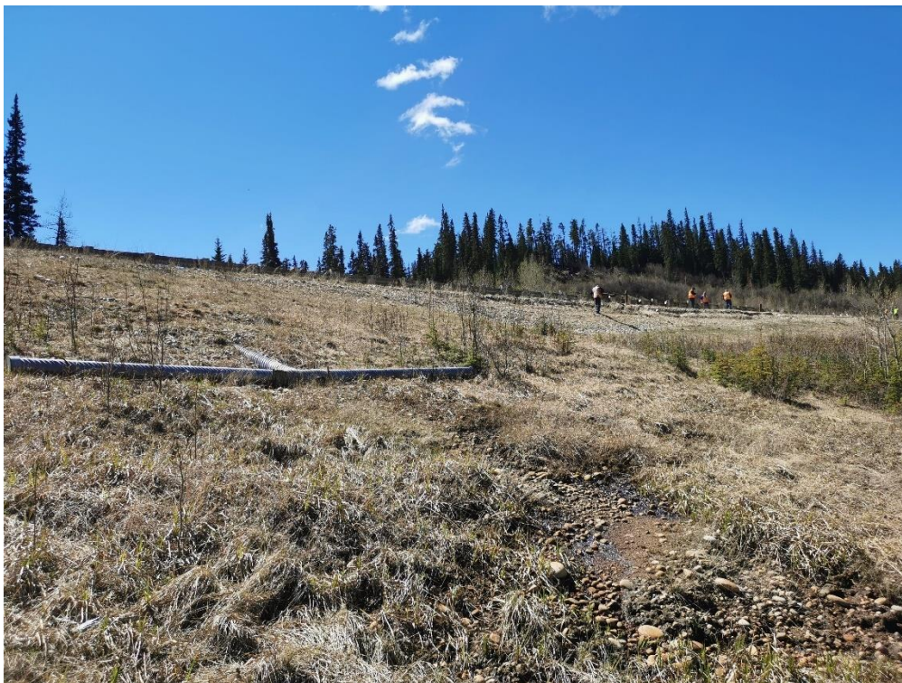
Photo 8, SH001-1 – Seepage out of slope below north-most T-drain.
