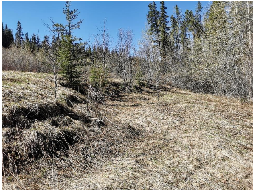
Photo 3, SH001-1 – Looking southwest at scarp on slope below highway between SI20 and SI21.
