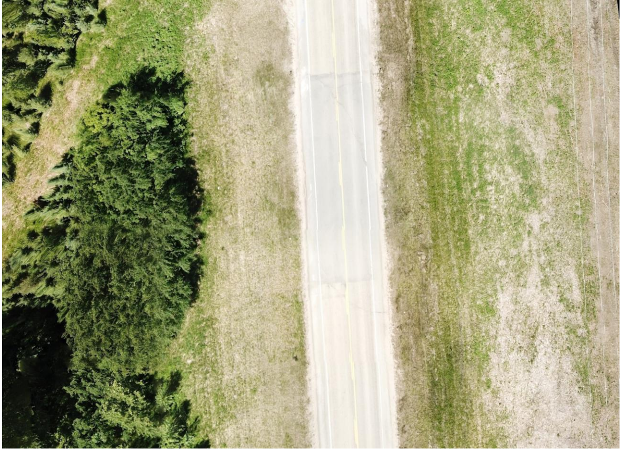
2018 UAV Image of patch section at north end of slide with drill access road to the west and new powerline on the east.
