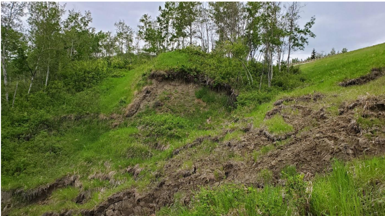
Photo 8 – Slide A: Downslope view, looking west. Over-steepened exposed slope face is more vegetated than in 2015. A former grass-covered access route is located on the left side of the small hill in the center of the photo.
