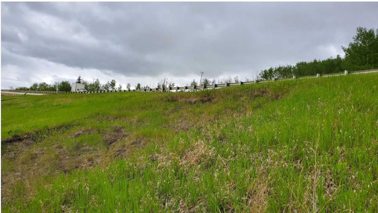
Photo 6 – Slide A: Embankment sideslope, looking northeast.
