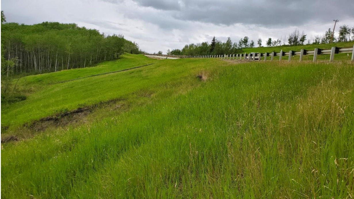
Photo 5 – Slide A: Increased retrogression movement, looking north.
