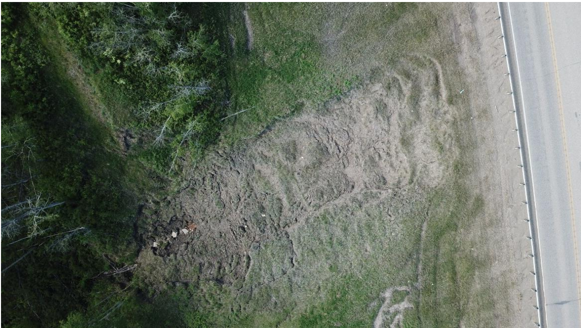
Slide A: 2020 UAV photo of landslide.
