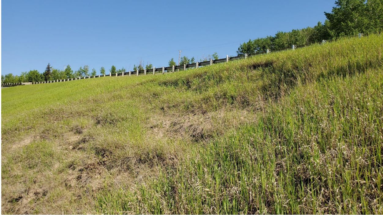
Photo 7 – Slide A: Embankment sideslope, looking northeast.
