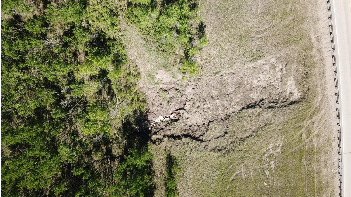
Slide A: 2022 UAV photo of landslide.
