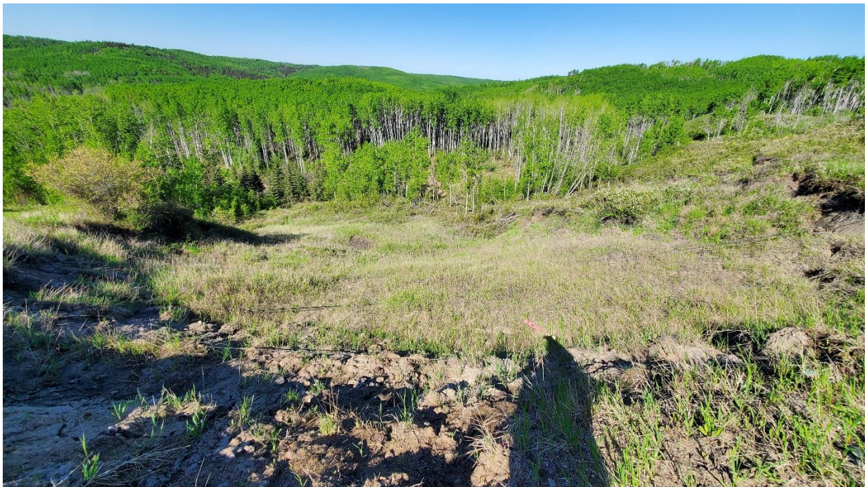
Photo 2 – Slide B: View of slope failure and landslide block, looking southwest.
