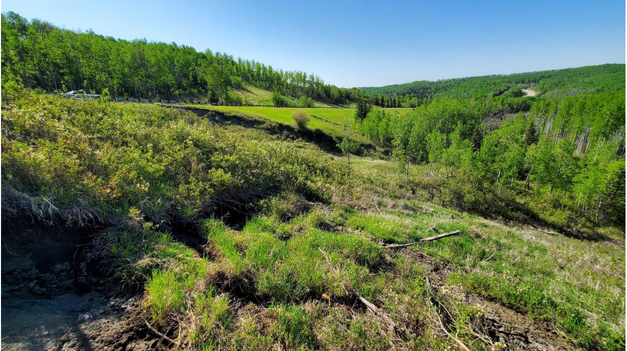
Photo 5 – Slide B: Looking south at the developing extension on the north side of the landslide.
