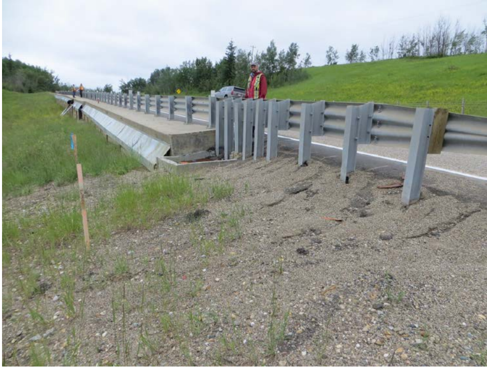
Photo 1 – Looking northwest at catch basin and pile wall.
