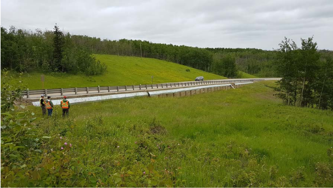
Photo 9 – From the north end looking east at pile wall with scarp in foreground.
