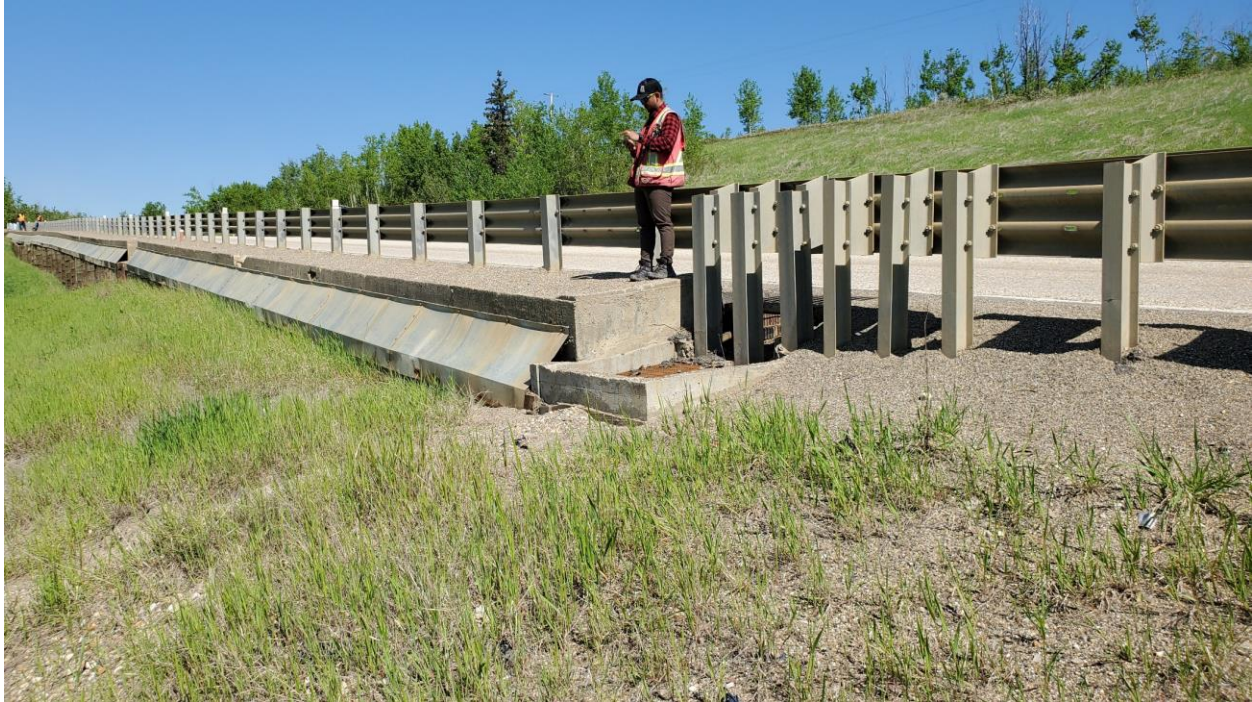
Photo 1 – Looking northwest at the catch basin and pile wall.
