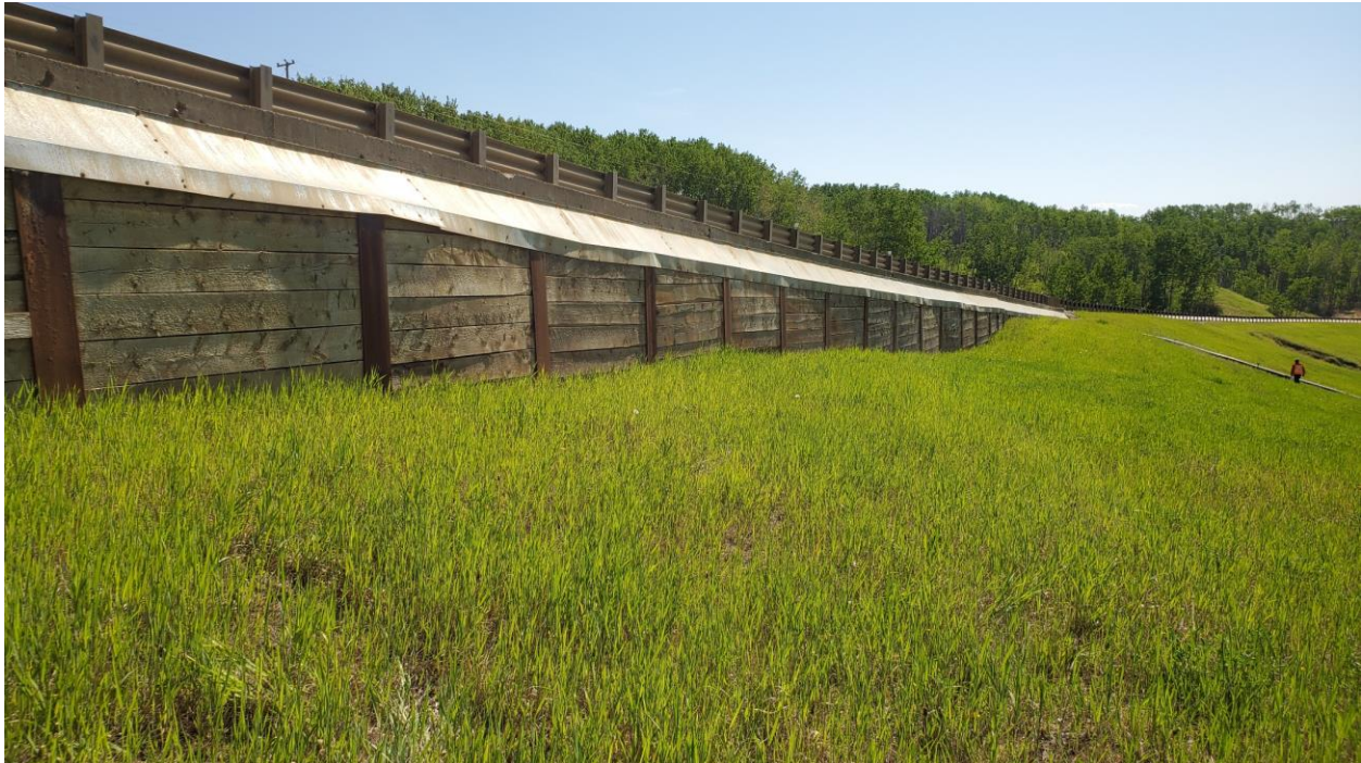
Photo 6 – Looking east at the end of the displaced section of lagging and beyond to (as yet) undisturbed lagging.
