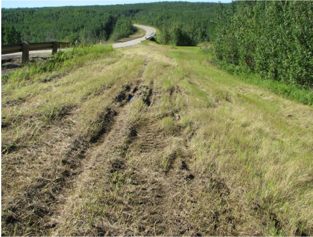
Photo 5 – Wet area at the back cut of access bench, looking southwest.
