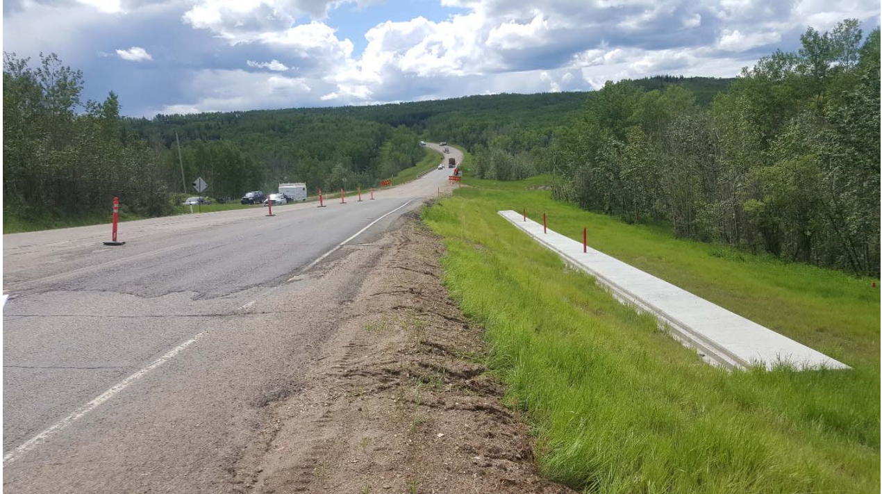
Photo 3 – Looking south along pile wall.
