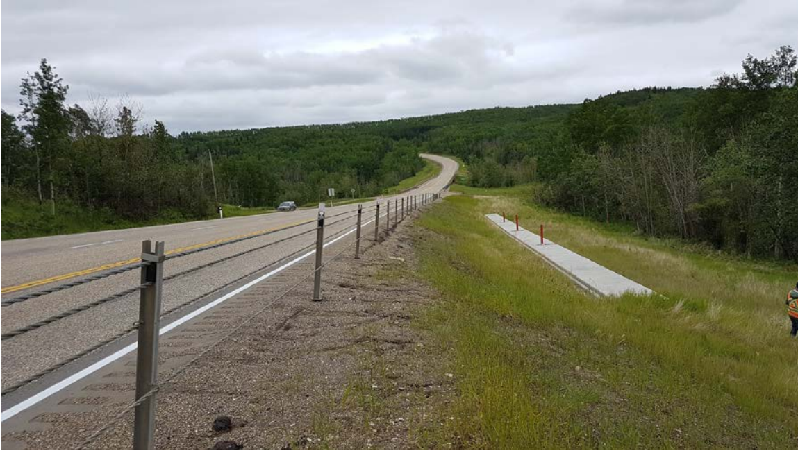
Photo 3 – Looking south along pile wall.
