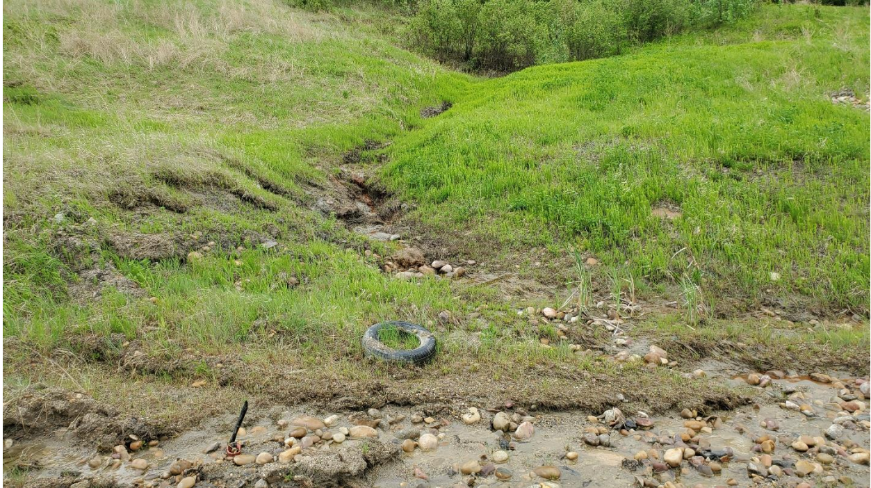
Photo 5: Recent grading (2019) of lower portion of the slope at toe of Slump B becoming vegetated.
