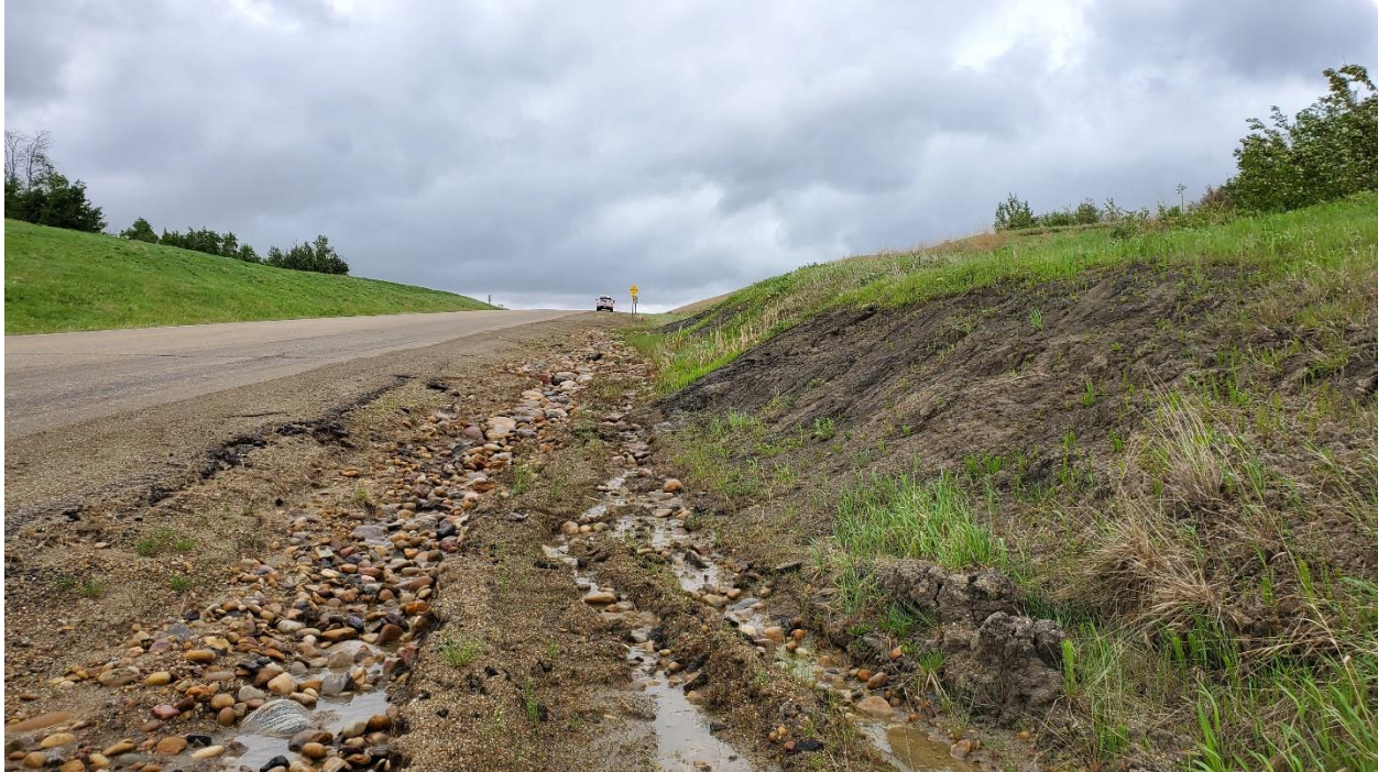
Photo 1 – Looking east at toes of Slumps B and A which were excavated in 2019 to improve ditch flow with the material placed back onto the slide masses.
