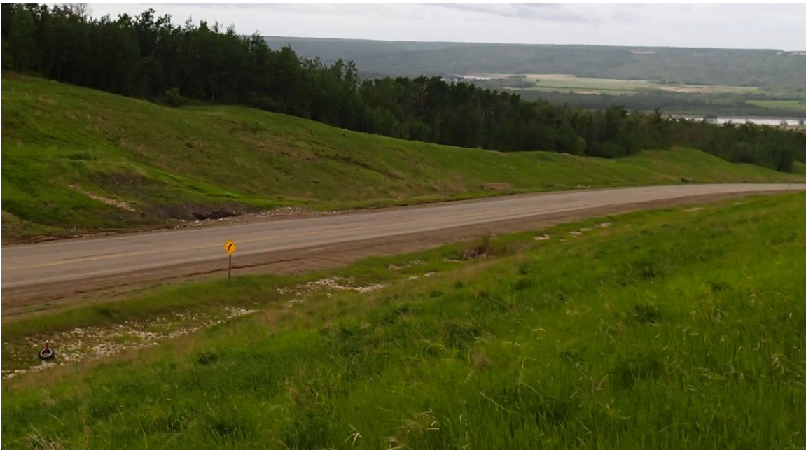
Photo 6: Looking southwest at Slump D (by R. Wang, TRANS).
