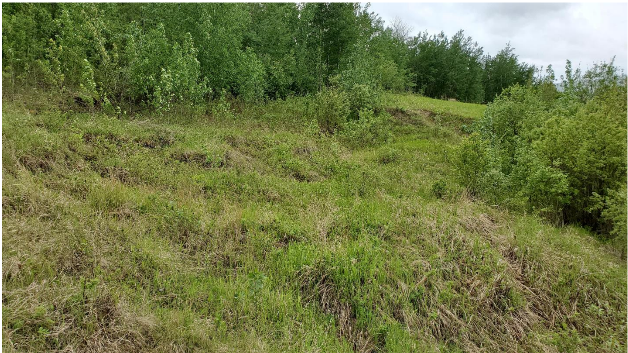
Photo 8: Looking west at top of Slump B.
