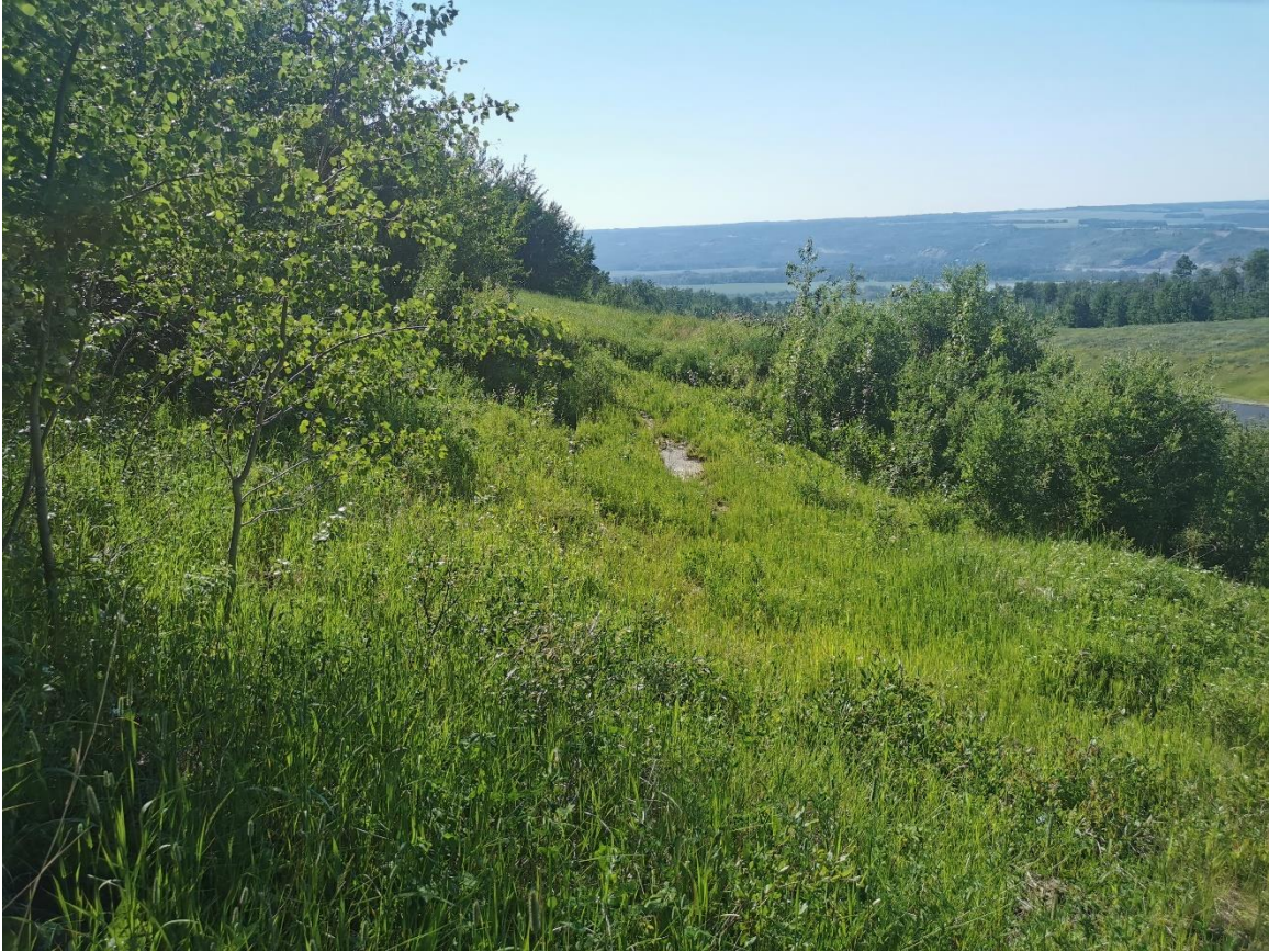
Photo 7: Looking west at top of Slump B.
