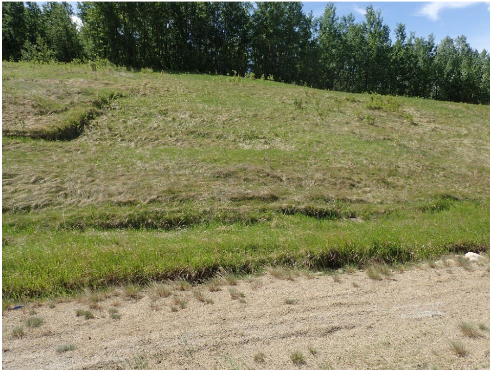
Photo 1 – Looking southwest at Slump D where extensions of scarps were observed due to continued creep movement.
