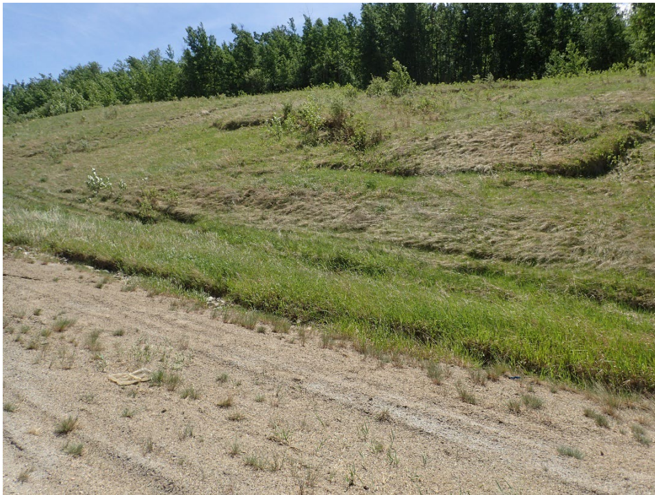
Photo 2 – Looking southeast toe bulges of Slumps D and E. No significant changes since 2023 inspection.
