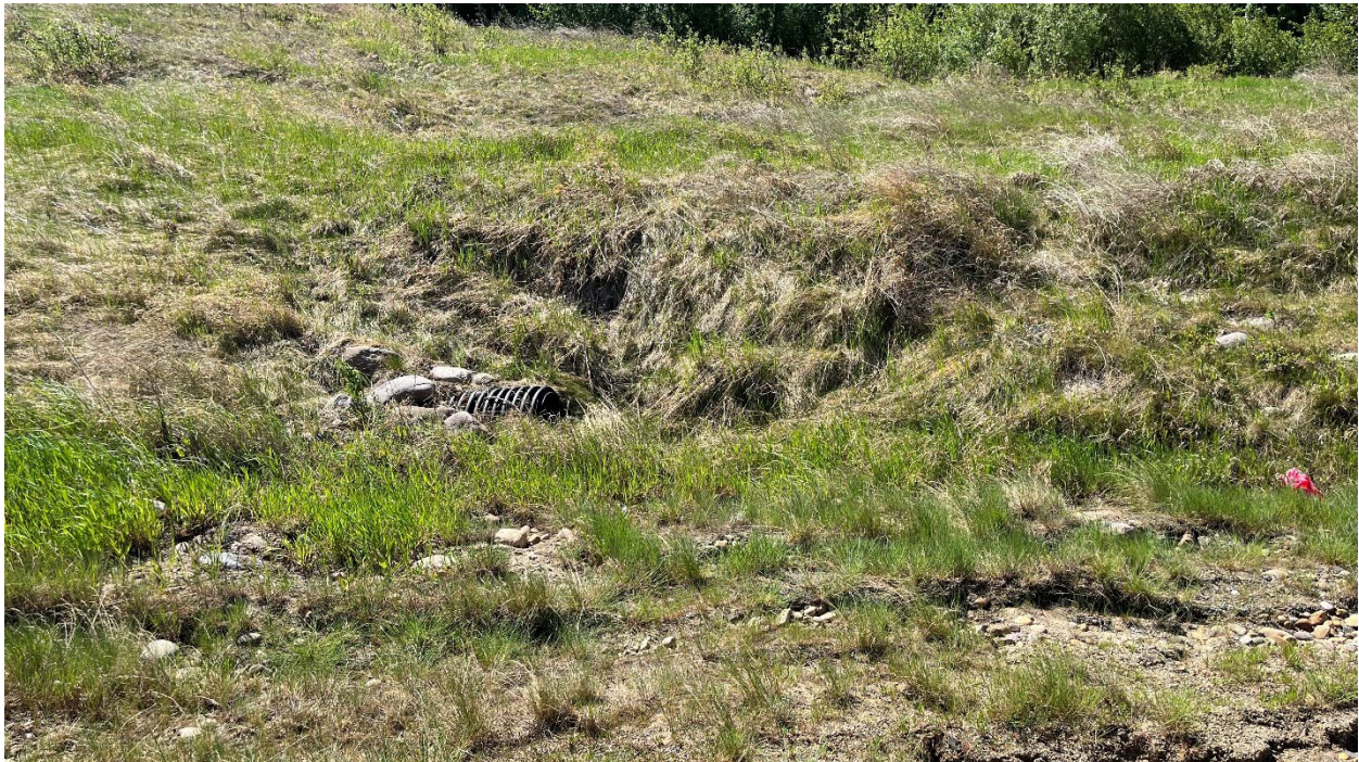
Photo 10: Lower south at culvert outlet with observed slumps upslope.
