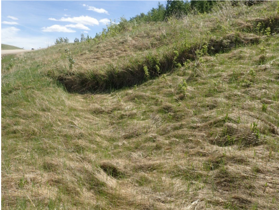
Photo 3 – Looking east at intermediate scarp within Slump D that has vegetation present.
