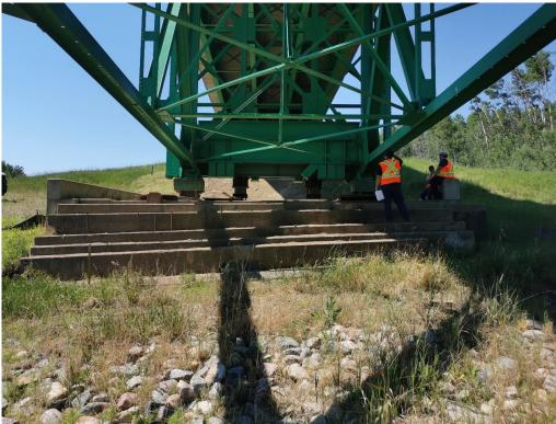
Photo 7 – Looking west at Pier 1 foundation which is tilted downward to the south.
