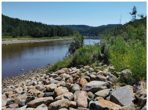
Photo 9 – Looking south at erosion along toe of riprap and riverbank.
