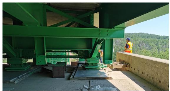
Photo 4: Sliding configuration at abutment.
