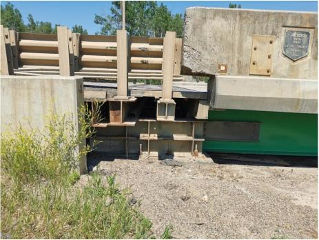
Photo 2 – Looking north at west bridge abutment. The two I-beams at the edge of the wingwall are the remainder of the 5 installed in 2000.
