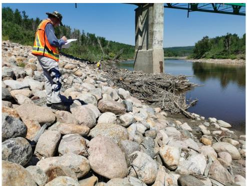
Photo 10: Oversteepening of riprap south of Pier 2.
