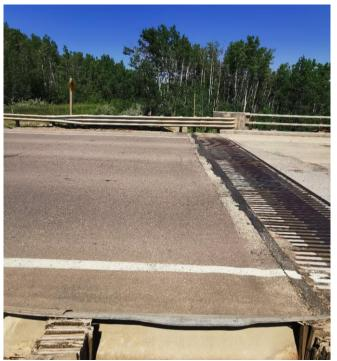
Photo 1 – Looking north at paved surface at the abutment expansion joint where cracks were previously observed
