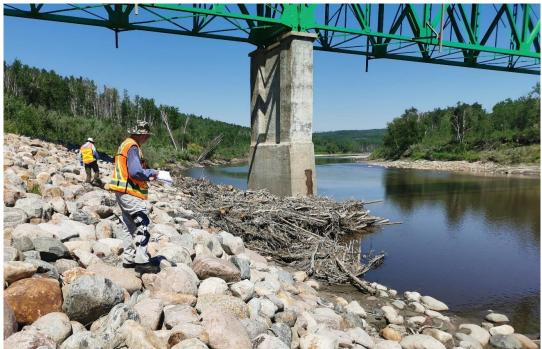
Photo 8 – Looking north at accumulated tree debris against Pier 2.
