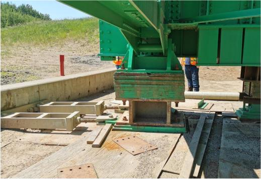
Photo 5 – Shims under rocker bearings at Pier 1.
