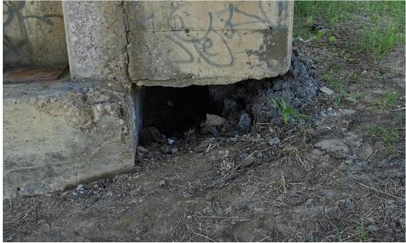
Photo 3 – Void on northeast corner of Abutment #1 exposing rusting H-pile.
