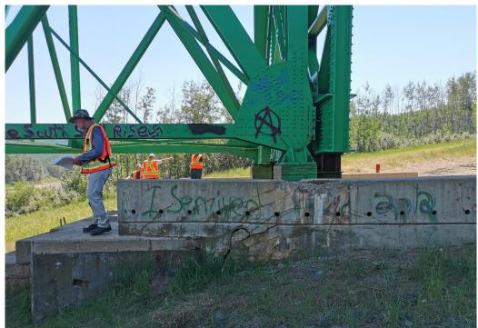
Photo 6 – Looking south at Pier 1 wingwall at arc-shaped crack pattern in foundation. Left-hand portion of foundation is pile supported; right-hand is on-grade.
