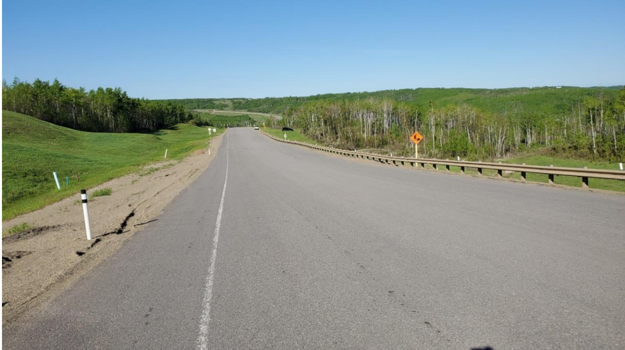
Photo 5 – Looking southwest an area of frequent patching in the main graben block movement between Sta. 0+600 and 0+800.
