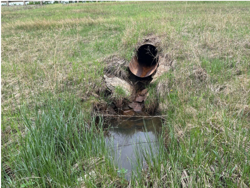
Photo 2 – Erosion bowl at outlet of the 750 mm diameter culvert at about Sta. 0+810.
