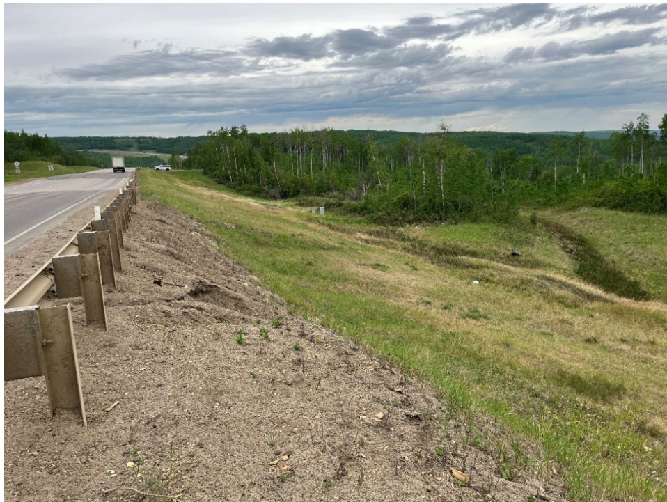
Photo 12 – Erosion rills by the guardrail and ravelling of the north side slope backscarp between Sta. 0+650 and 0+700.
