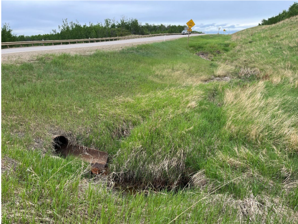
Photo 15 – Erosion at the culvert inlet (foreground). Scour bowl (background) at Sta. 0+430 is encroaching towards the highway.
