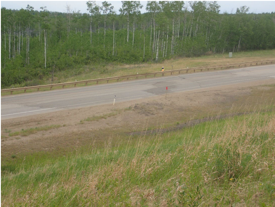
Photo 6 – Looking northeast at where main scarp crack crosses highway at Sta. 0+600.
