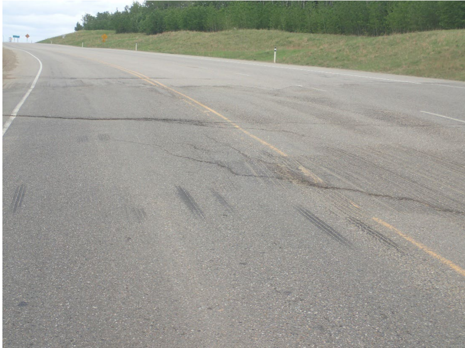
Photo 9 – Looking southeast at cracks that were milled at Sta. 0+600.
