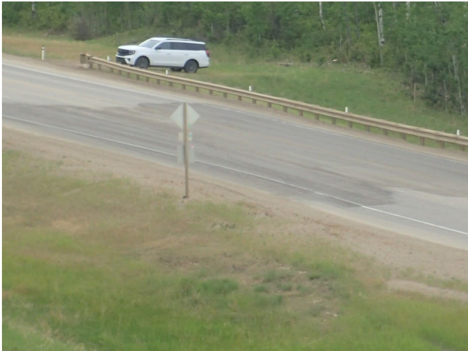
Photo 8 – Looking northwest at where main scarp crack crosses highway at Sta. 0+780.
