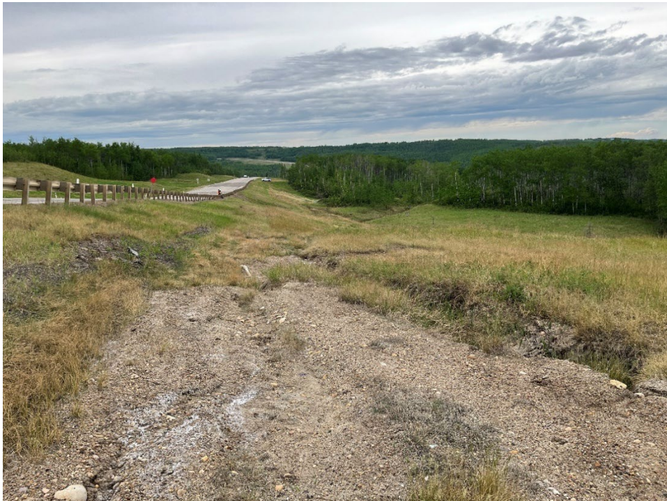
Photo 14 – Looking southwest along erosion gully near Sta. 0+550.
