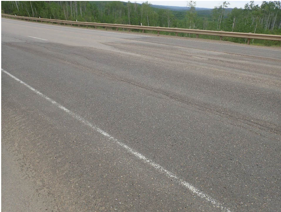
Photo 5 – Looking northwest at area of frequent patching at Sta. 0+700.
