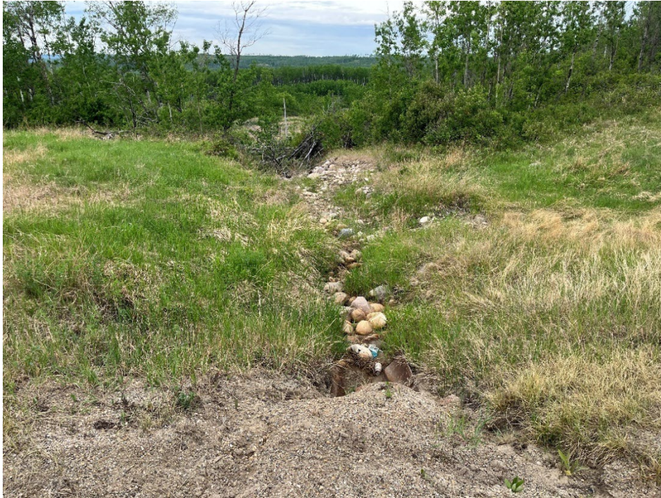
Photo 13 – Erosion gully at outlet of culvert at about Sta. 0+470.
