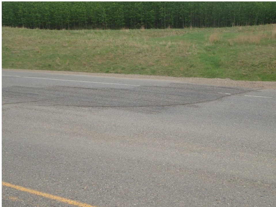
Photo 10 – Looking south at cracks that were milled at Sta. 0+600.
