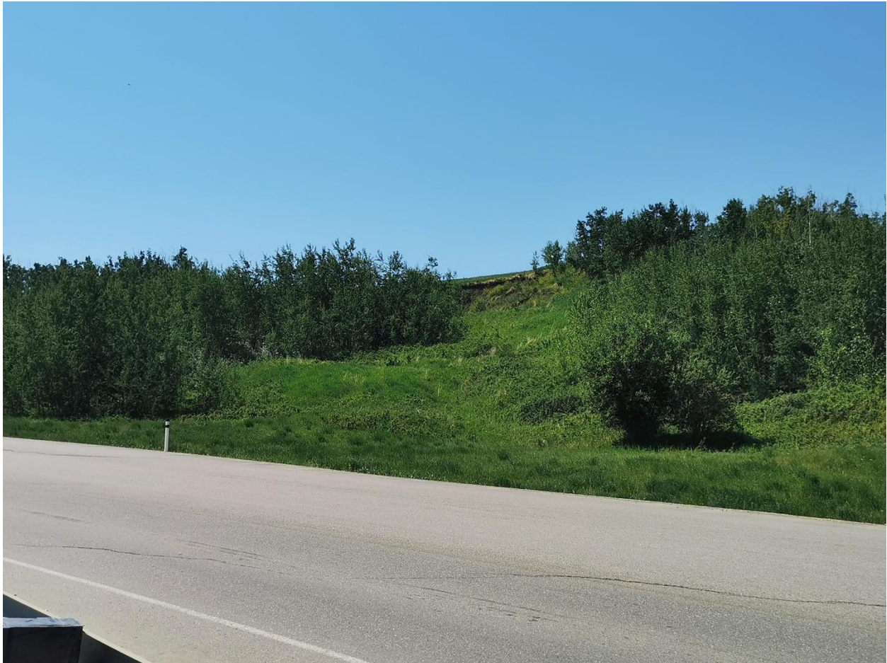
Photo 2 – Looking southwest at slide movement in the backslope above the highway.
