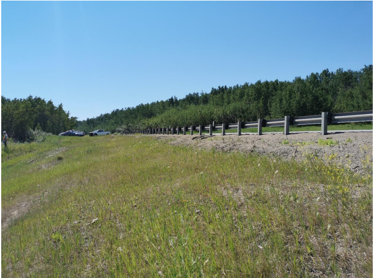
Photo 4 – Looking southwest at guardrail at south end of site.
