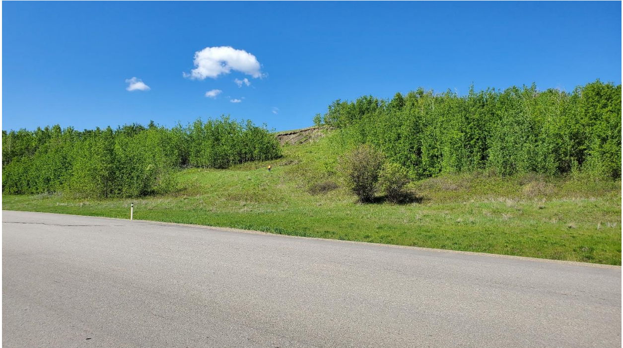
Photo 2 – Looking southwest slide movement in the backslope above the highway.
