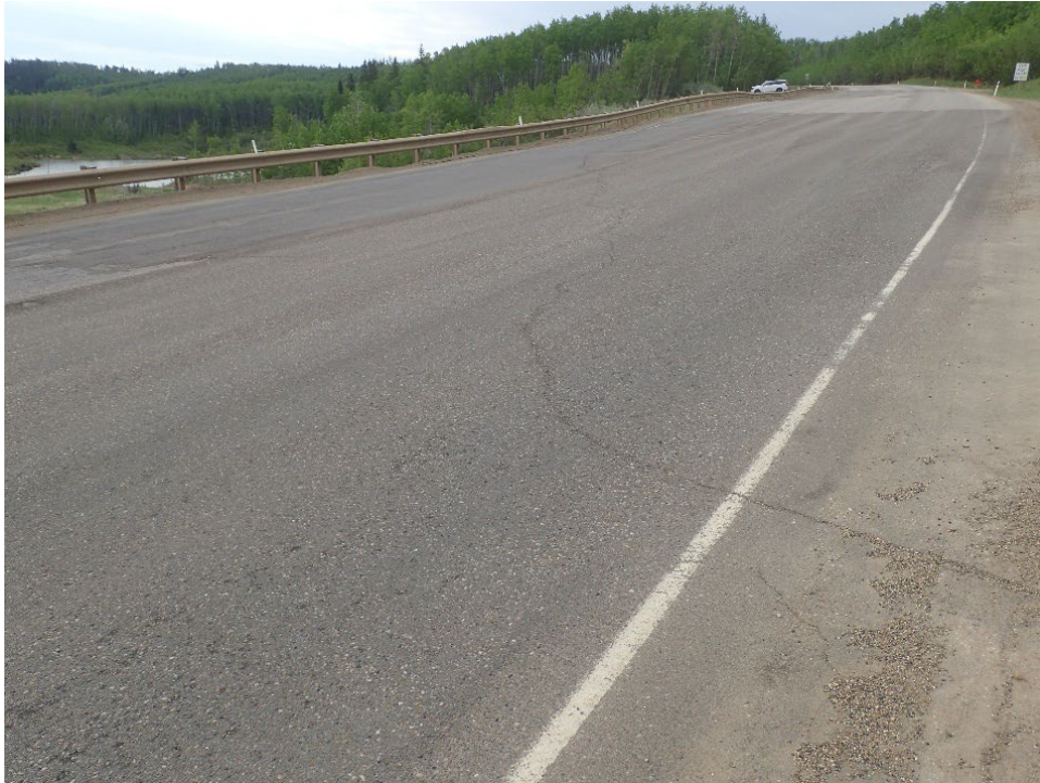
Photo 9 – Looking south at third set of scarp cracks from north end of east guardrail.
