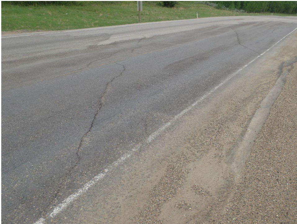
Photo 3 – Looking north at second set of scarp cracks just north of Photo 2.
