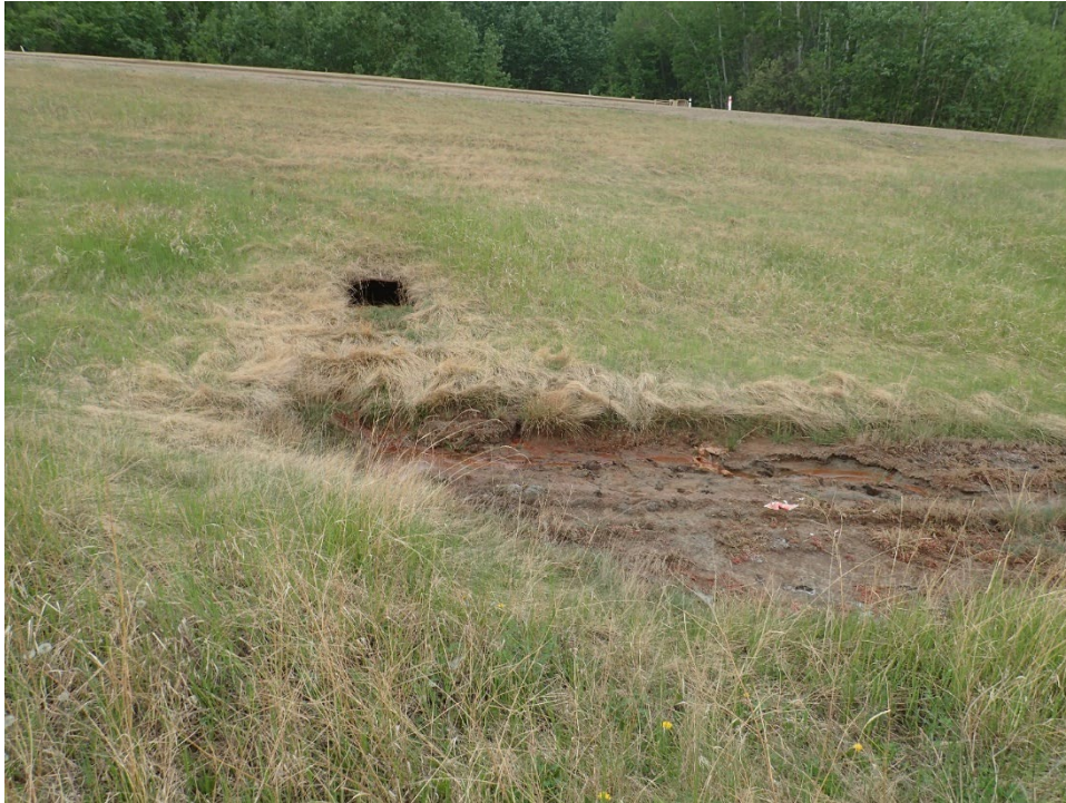
Photo 14 – Looking west at culvert outlet with observed rust-stained area and soft ground.
