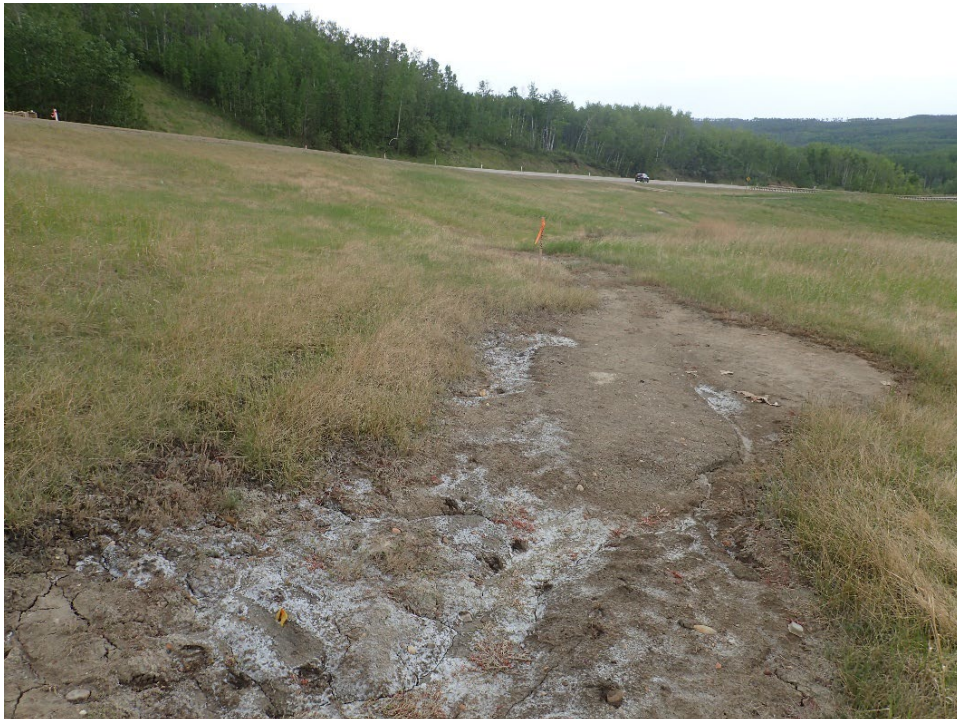
Photo 13 – Looking north at bare area on sideslope with previously observed seepage. Area was observed to be dry in 2025.
