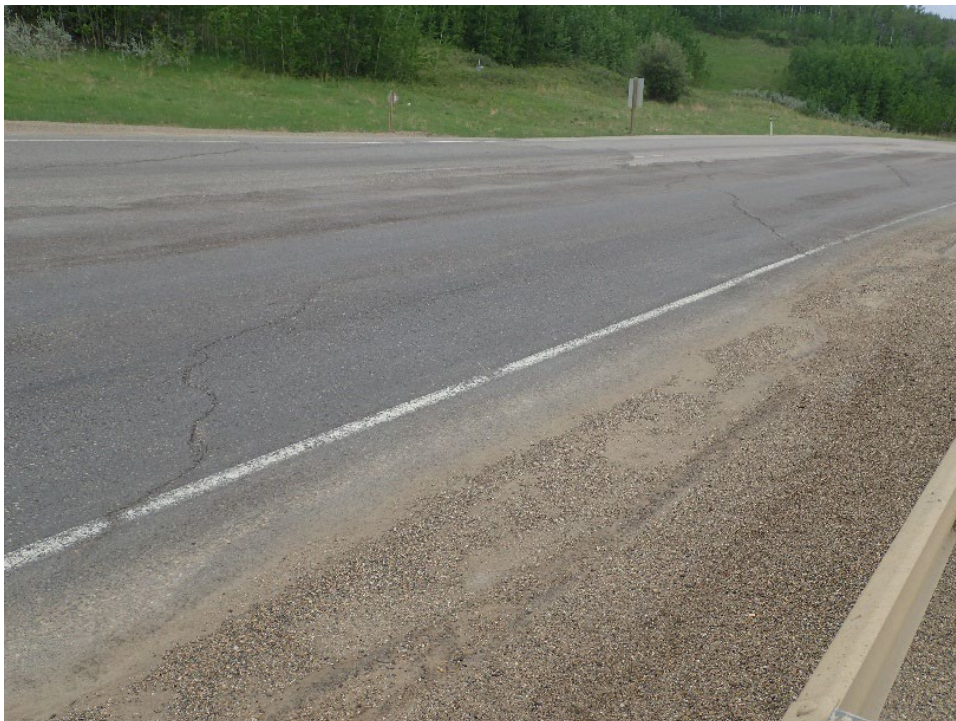
Photo 2 – Looking north at the first set of scarp cracks at south end of the site.
