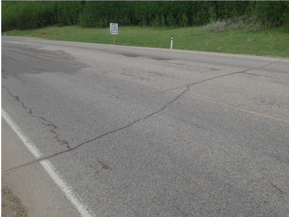
Photo 7 – Looking west at cracks present outside of patched areas.
