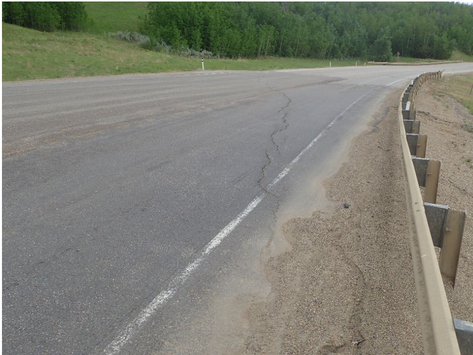
Photo 8 – Looking north at third set of scarp cracks near the north end of the east guardrail.
