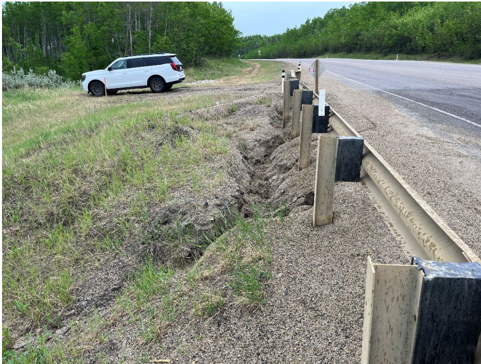
Photo 5 – Looking south at an erosion gully present at the south end of the guardrail.
