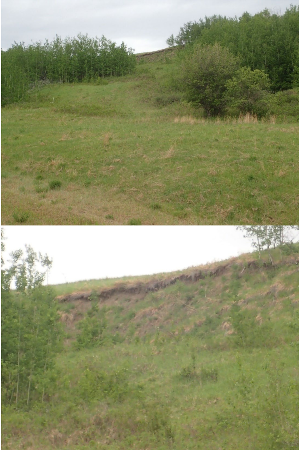
Photo 10, 11 – Looking at the southwest slide movement in the backslope above the highway.
