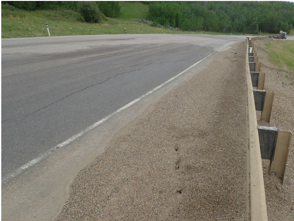
Photo 4 – Looking north at extensions of cracks just north of Photo 3. Note small voids present on shoulder adjacent to guardrail.
