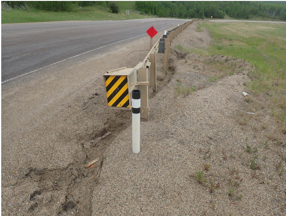
Photo 1 – Looking north at an erosion gully that extends past south end of the guardrail.
