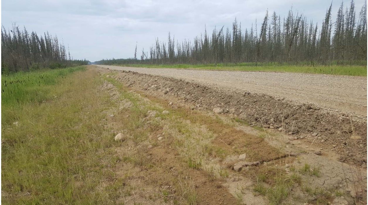
TEL Photo 1: Looking east toward start of distressed and note the thickness of pitrun placed in May 2016.
