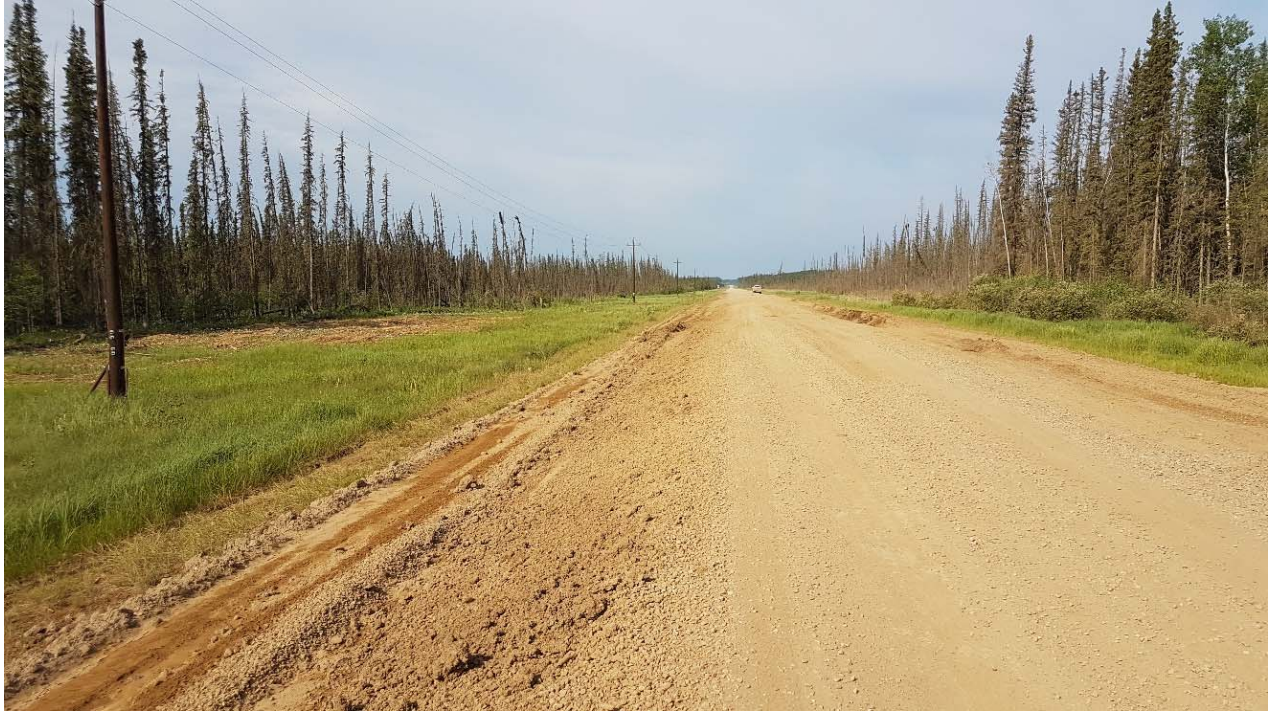
Photo 5 – Looking east at grading work. Note that shoulder (left side of photo) has been scraped back onto highway surface and rutting on the other shoulder (right side)
