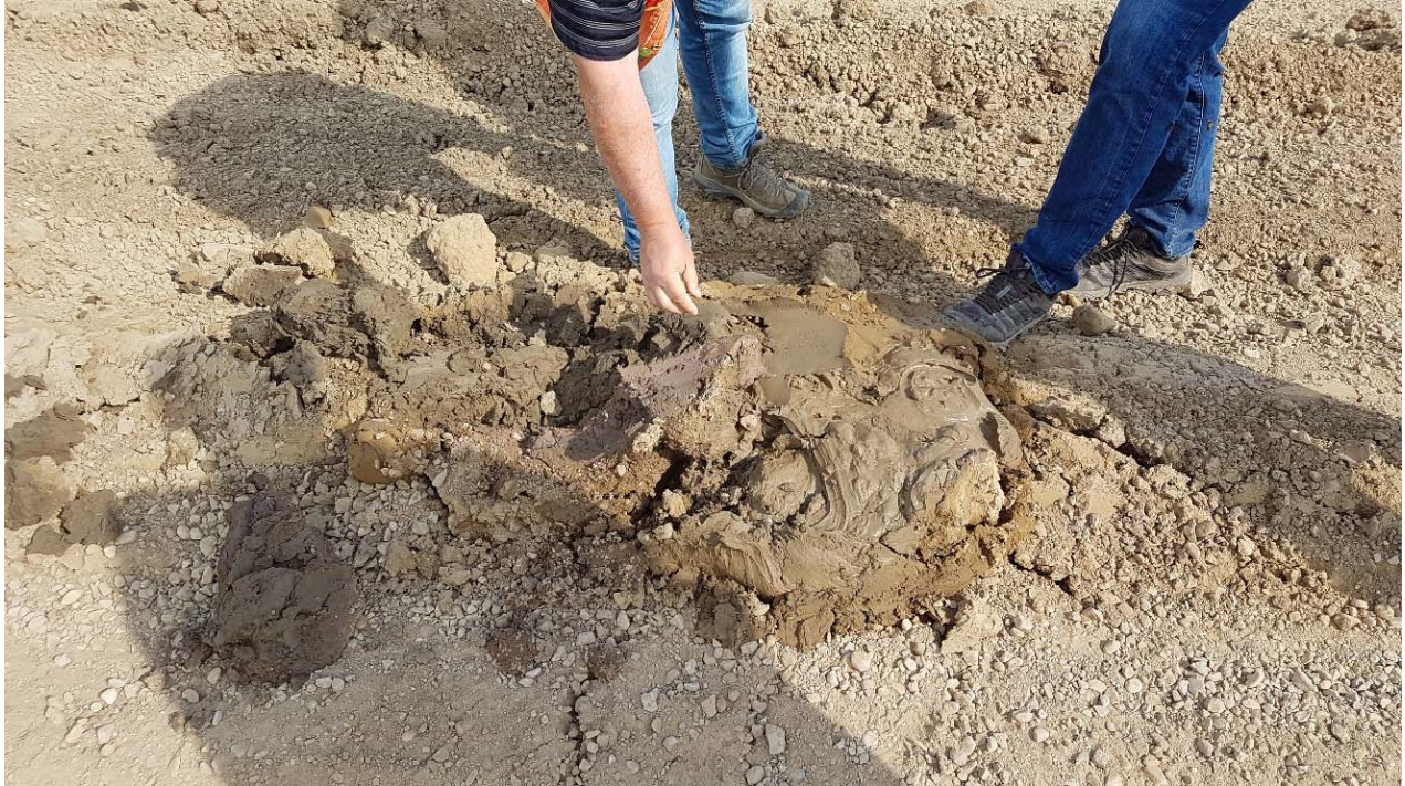
Photo 7 – Saturated silty material pushed up through rut by grader traffic.
