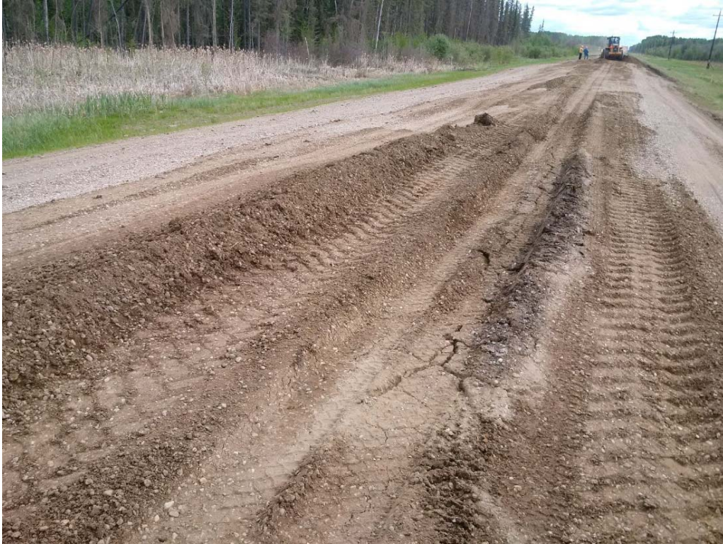
Photo 3 – Looking east at rutting during gravel placement on May 30, 2018 (AT photo).
