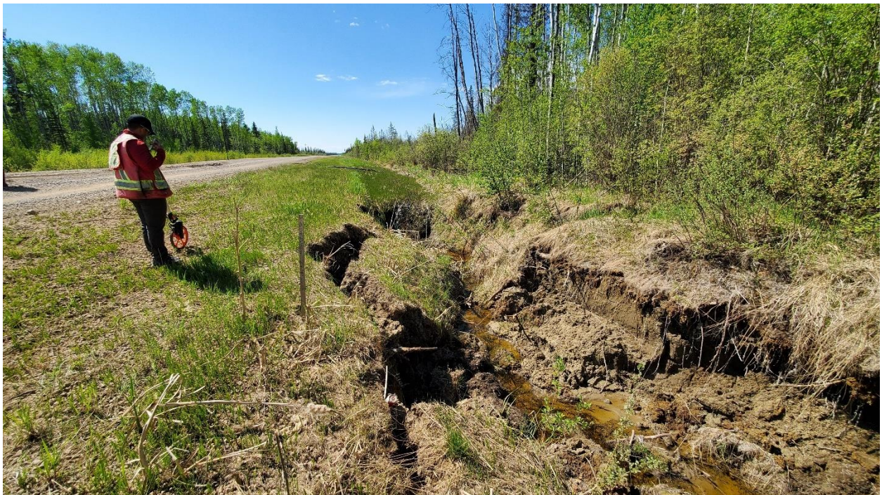
Photo 2 – Looking west at rutting during gravel placement on May 30, 2018 (AT photo)
