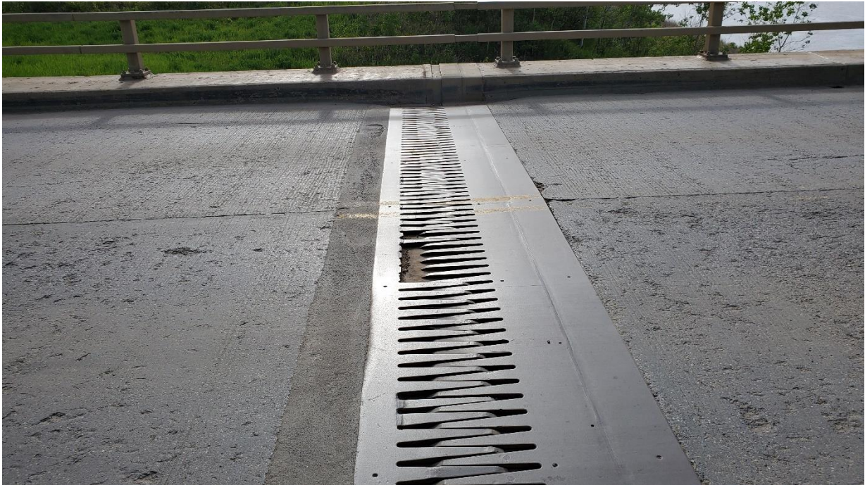
Photo 1, North – Looking east at north abutment finger joints.
