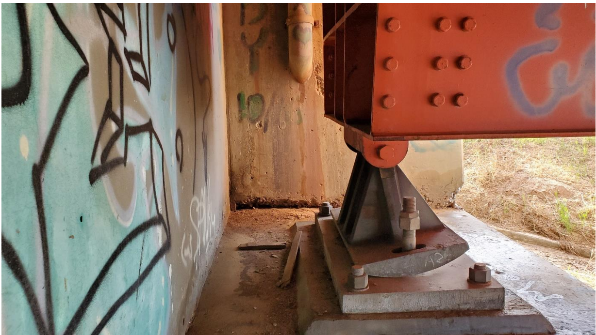
Photo 9, North – Looking east at north abutment east rocker bearing.
