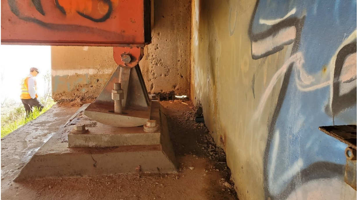
Photo 17, South – Looking east at south abutment east rocker bearing.
