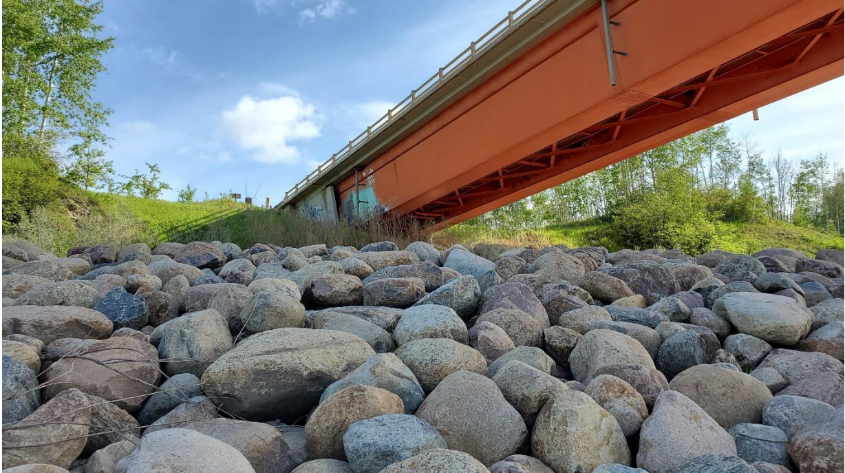
Photo 4, North – Looking north at west side of north abutment.
