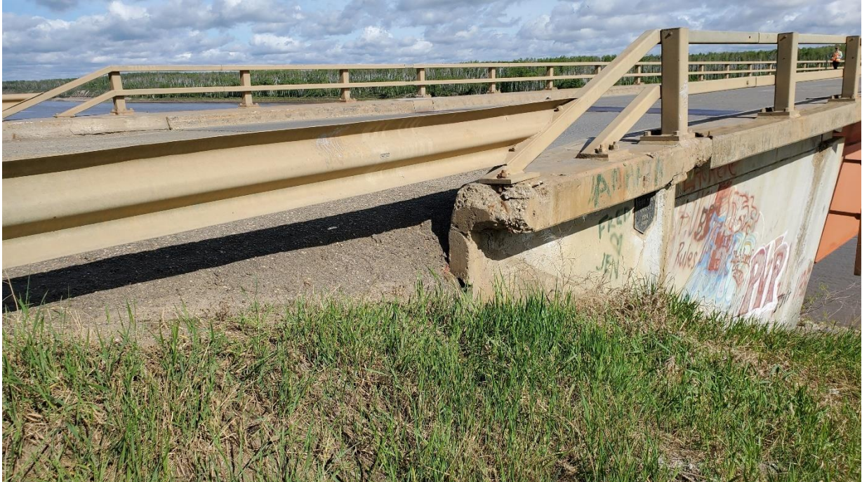
Photo 12, South – Looking northeast at top of east side wing wall.
