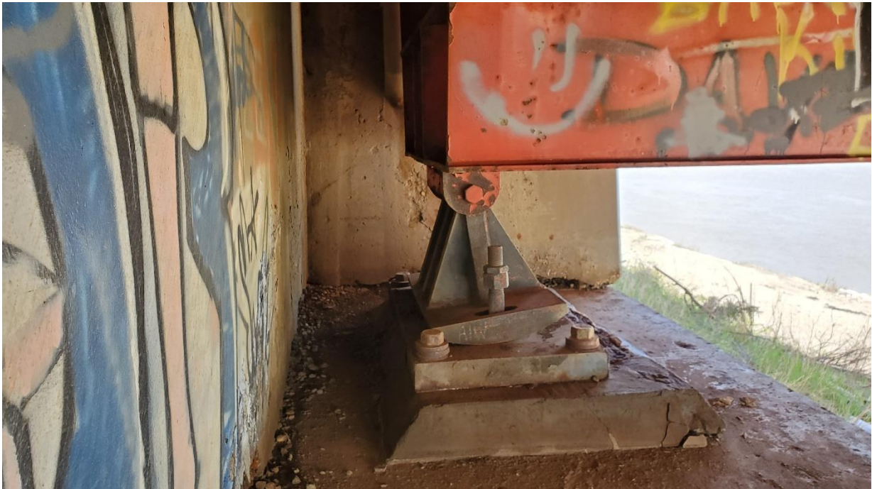
Photo 18, South – Looking west at south abutment west rocker bearing.
