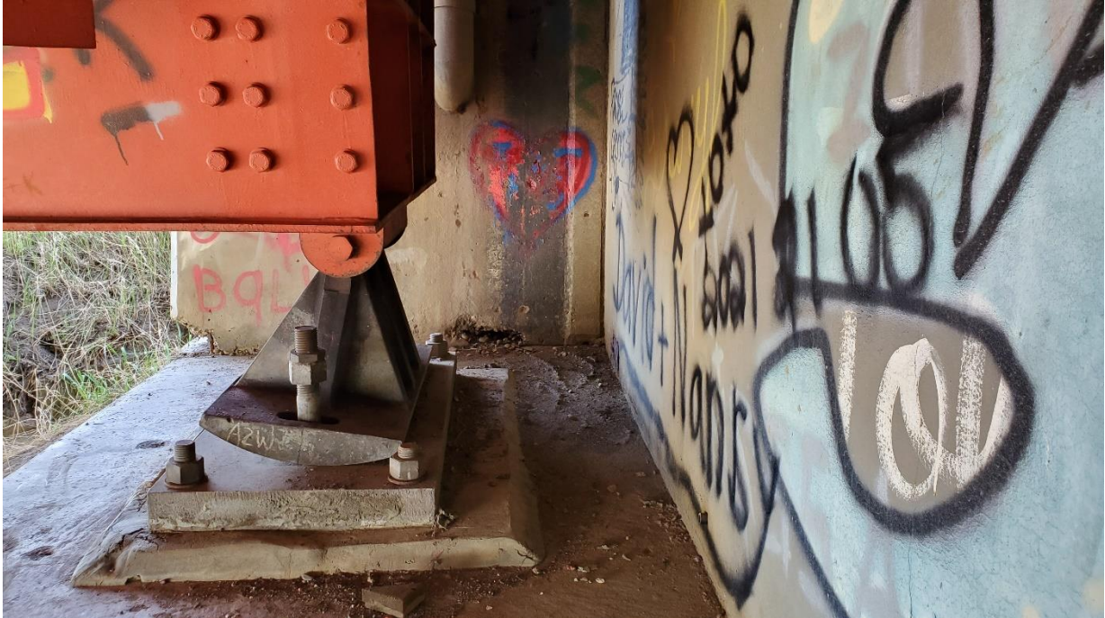
Photo 8, North – Looking west at north abutment west rocker bearing.
