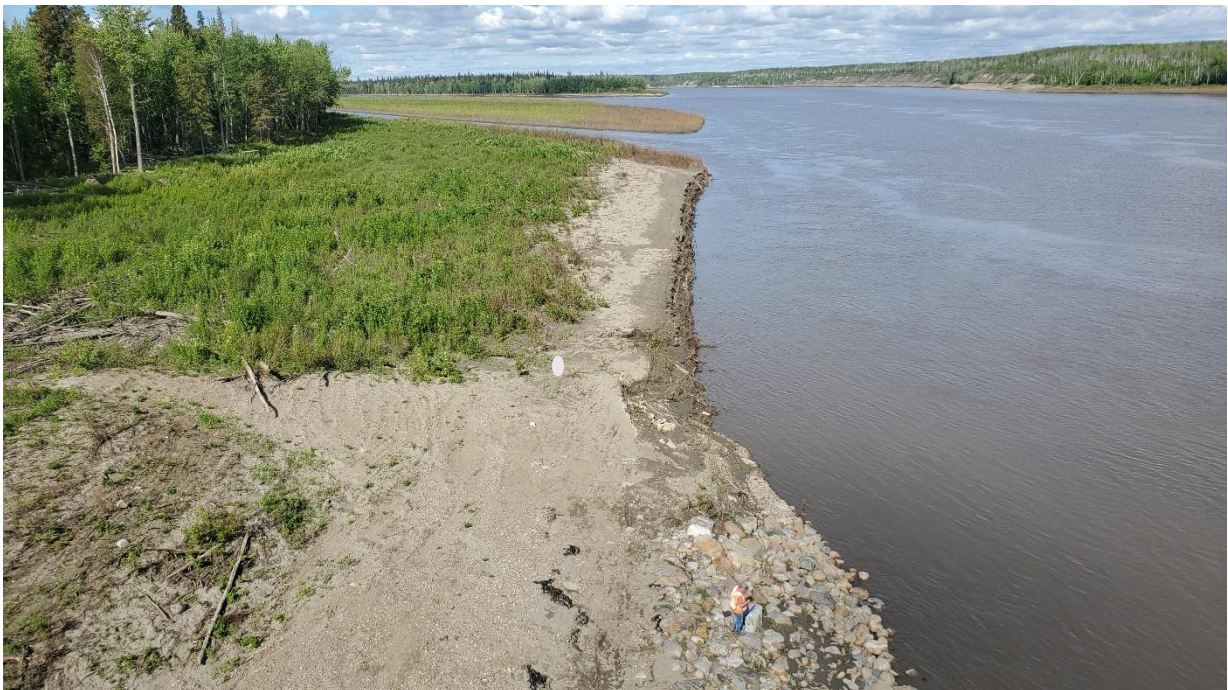
Photo 20, South – Looking south at west side of south abutment.
