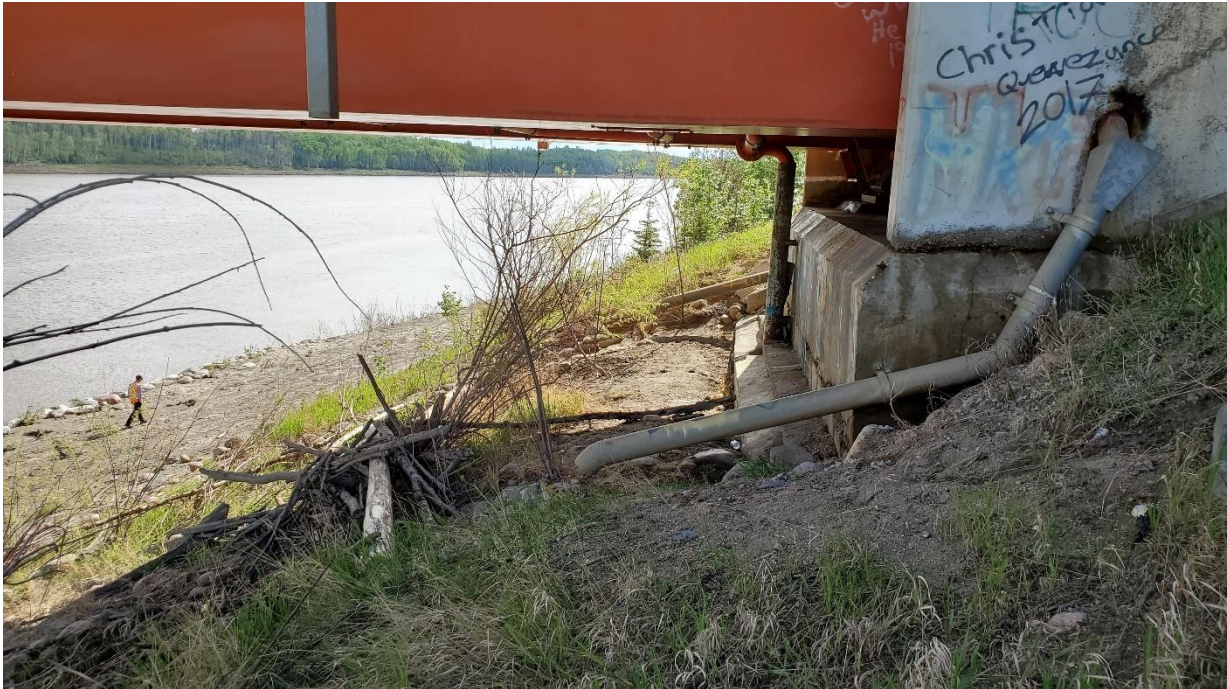
Photo 14, South – Looking east at south abutment concrete wall.
