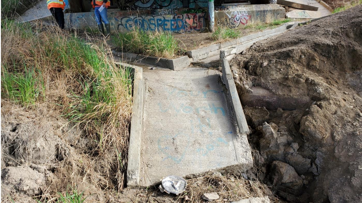
Photo 3A, North – Looking north at north abutment concrete gutter.
