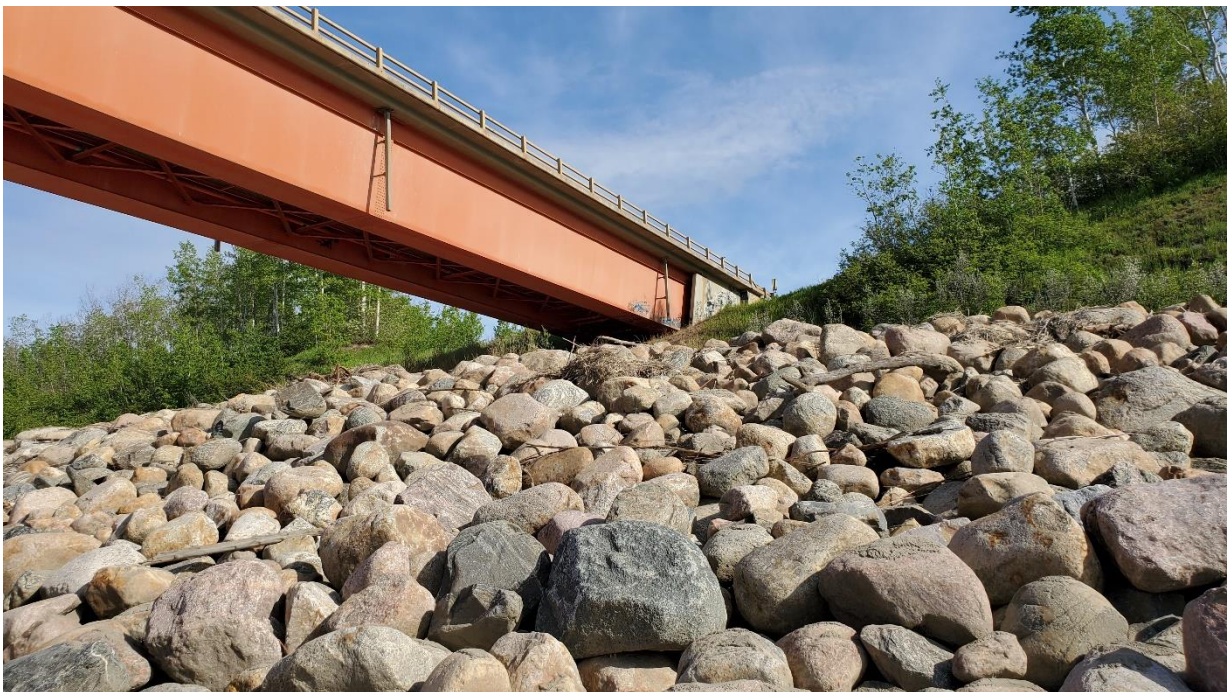
Photo 5, North – Looking north at east side of north abutment.
