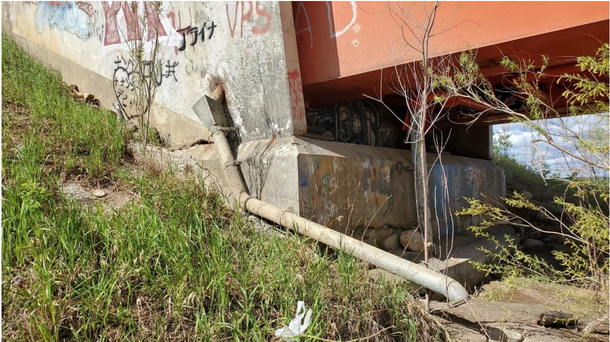
Photo 16A, South – Looking southwest at south abutment concrete wall.
