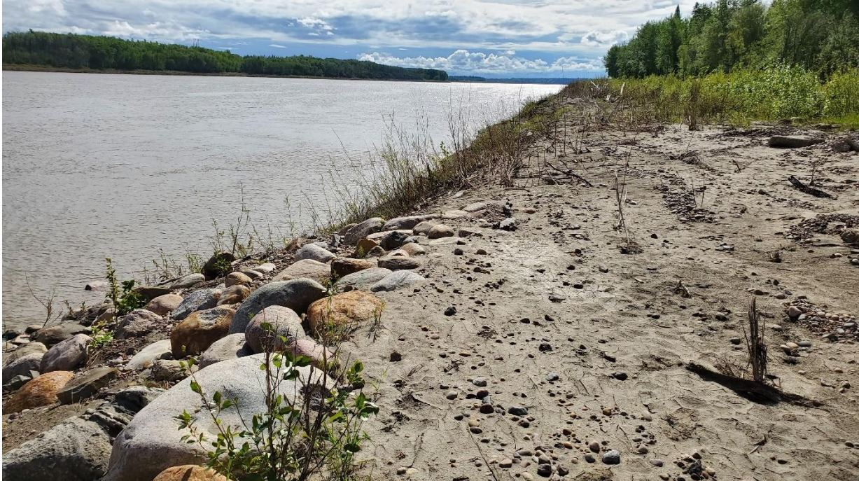
Photo 21, South – Looking east at new toe berm under south abutment.
