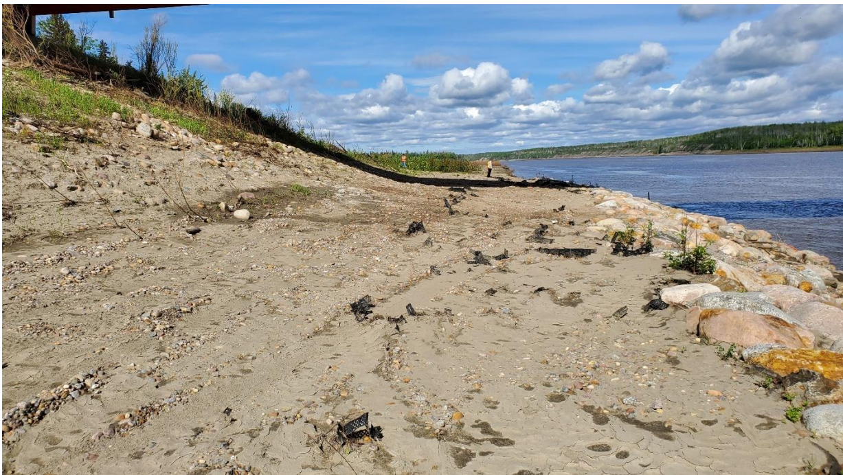
Photo 15, South – Looking west at new toe berm at south riverbank. Erosion of gravel at the top of toe berm occurred with high flood levels in Spring 2018 exposing GeoCell at several locations.
