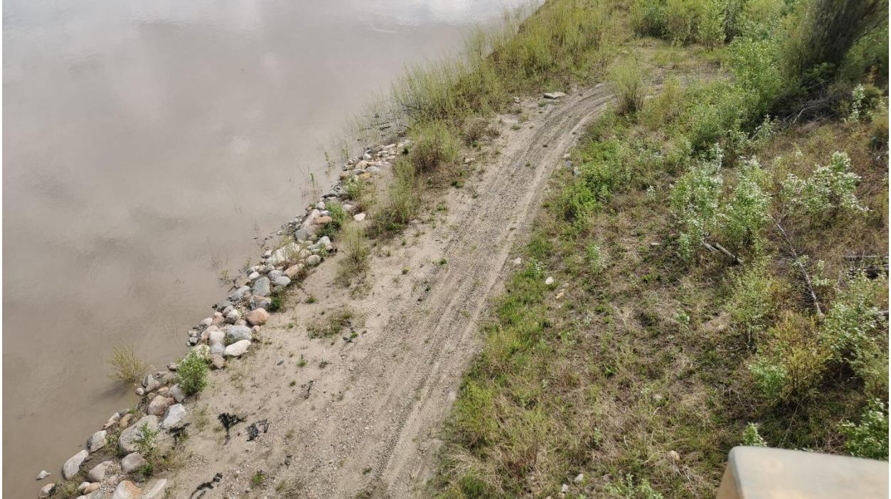
Photo 19, South – Looking at east side of south abutment with completed construction of toe berm.
