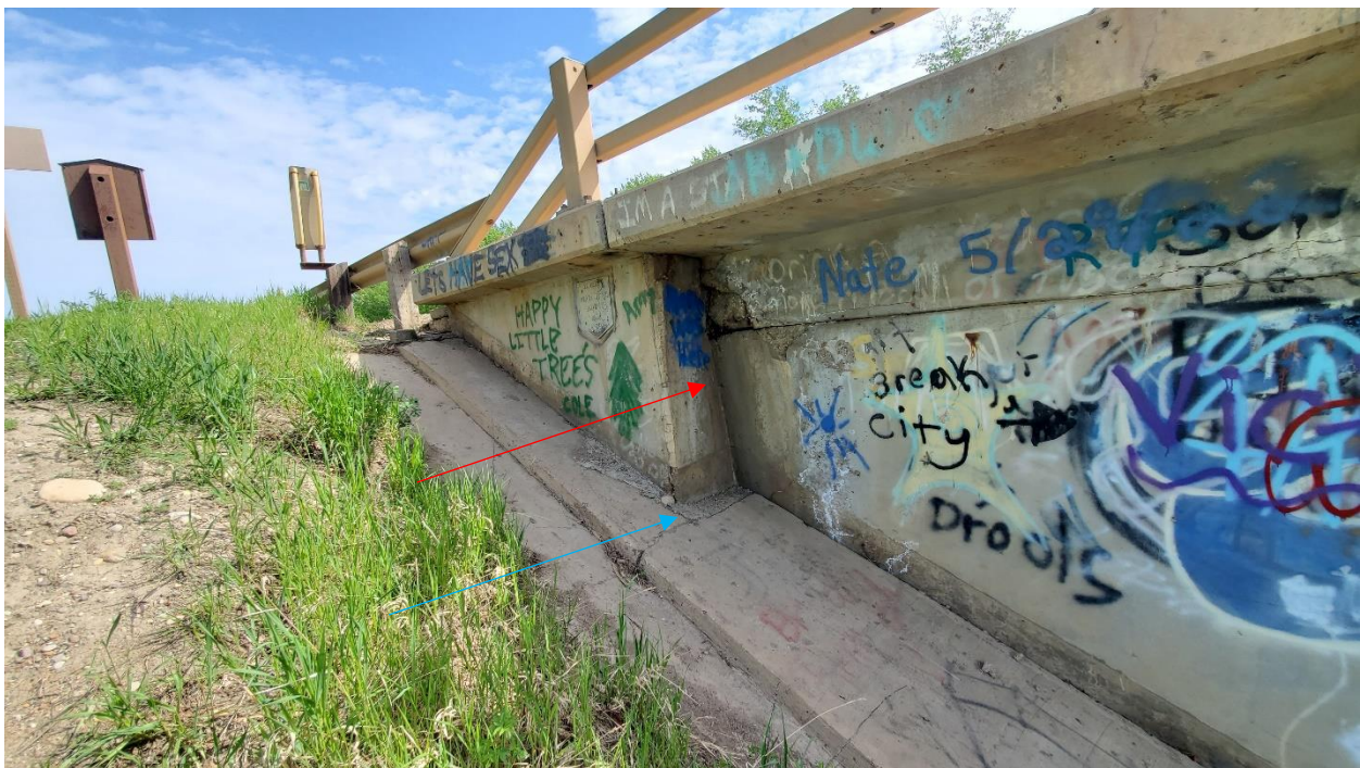
Photo 11A, North – Looking northeast at north abutment west side wing wall. Blue arrow shows recent grouting of voids. Cracking of beam denoted by red arrow shown in Photo 11B.
