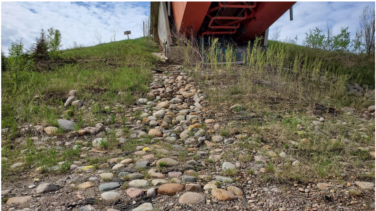
Photo 23B, South – Riprap placed in 2015 on south headslope below east deck drain.
