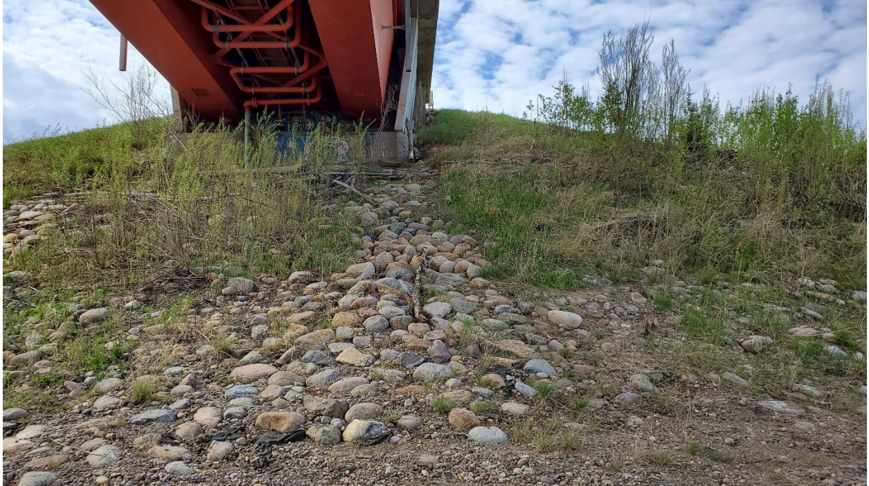
Photo 23A, South – Riprap placed in 2015 on south headslope below west deck drains.
