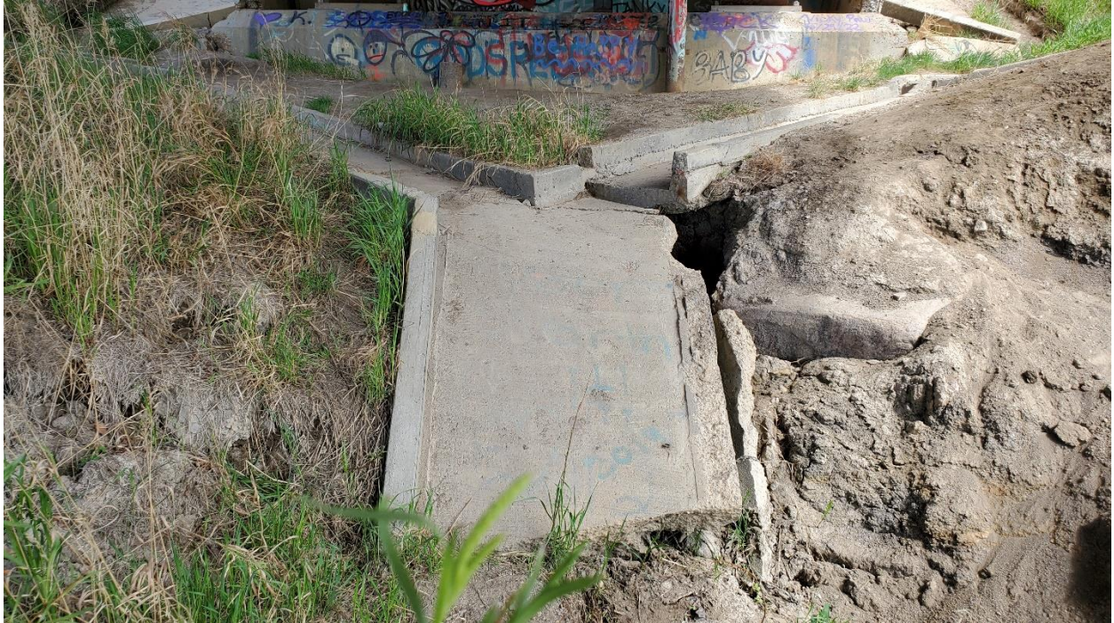
Photo 3A, North – Looking north at north abutment concrete gutter. Void below the gutter is up to 670 mm deep.
