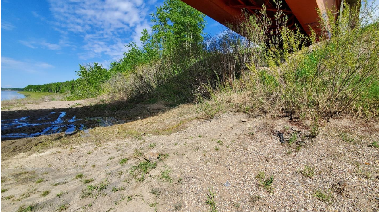
Photo 6, North – Seepage along toe of headslope face just above the top of the toe berm which is ponding on the surface of the berm.
