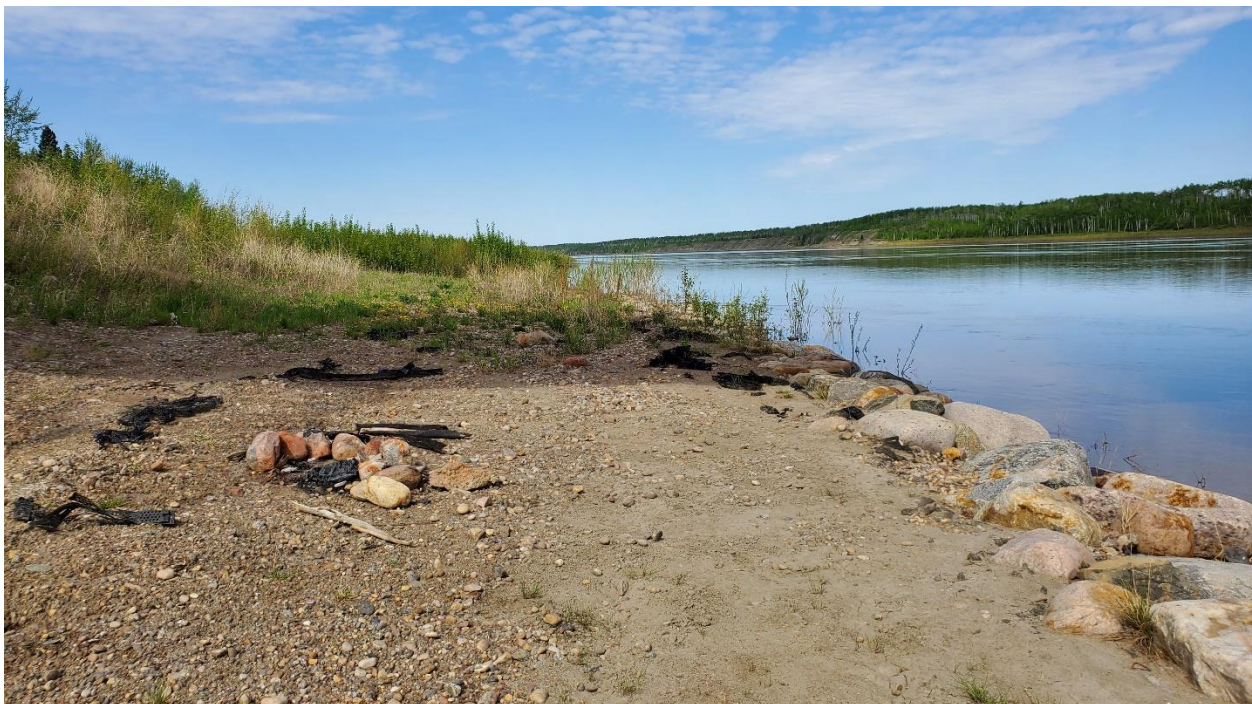
Photo 15, South – Looking west at new toe berm at south riverbank. Erosion of gravel at the top of toe berm occurred with high flood levels in Spring 2018 and 2022 exposing the GeoCell at several locations.
