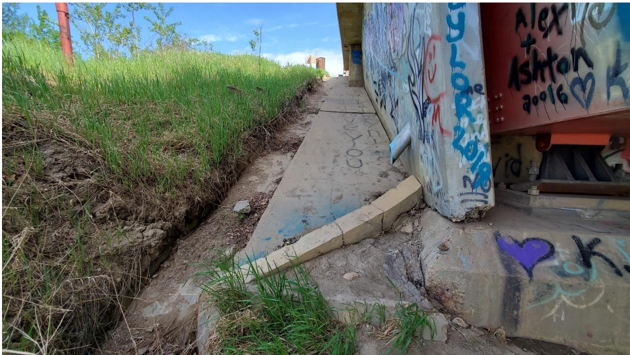
Photo 11C, North – Hump of material creeping into concrete drainage trough adjacent to west wingwall.
