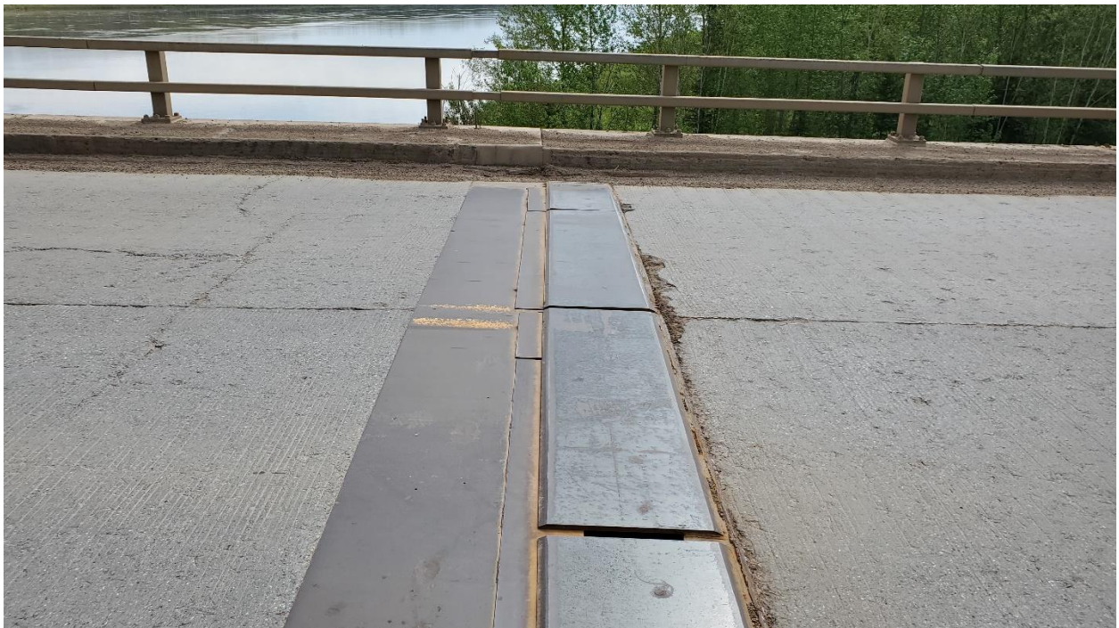
Photo 22, South – Looking east at south abutment finger joints which was covered with a plate between the 2017 and 2018 visits and repaired prior to the 2022 visit.
