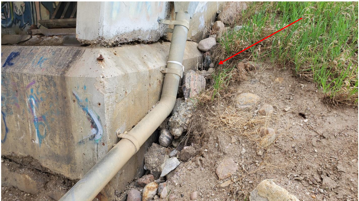
Photo 13, South – Looking southeast at south abutment west side wing wall. Erosion occurring at the base of the wall.
