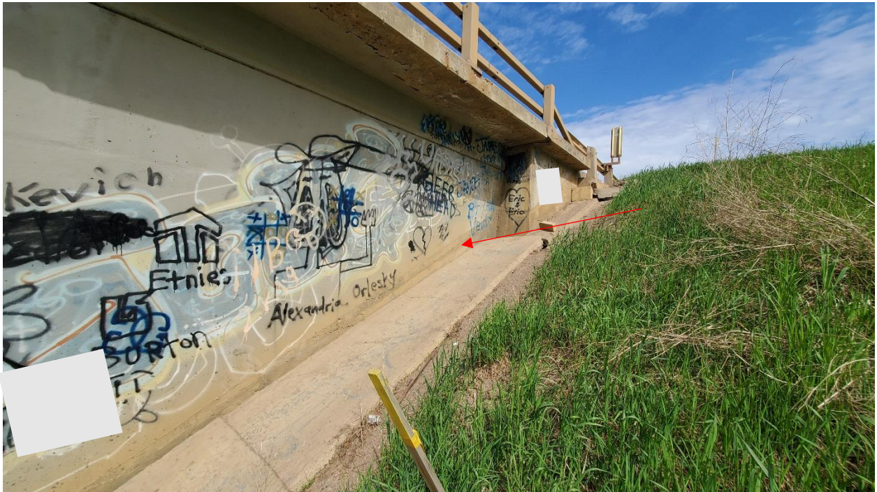
Photo 7, North – Looking northwest at gap between the concrete gutter and north abutment wing wall resulting from settlement of abutment fill.
