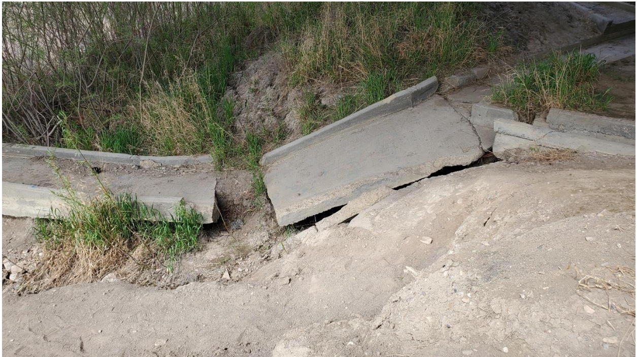
Photo 3B, North – Looking west at cracked and shifting north abutment concrete gutter. Void below the lower portion of the slab up to 300 mm (measured from top of concrete).
