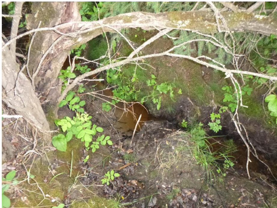
Photo 10 – Looking south at the stream below the west end of the slide. The streambed is in the order of 0.5 m wide here.
