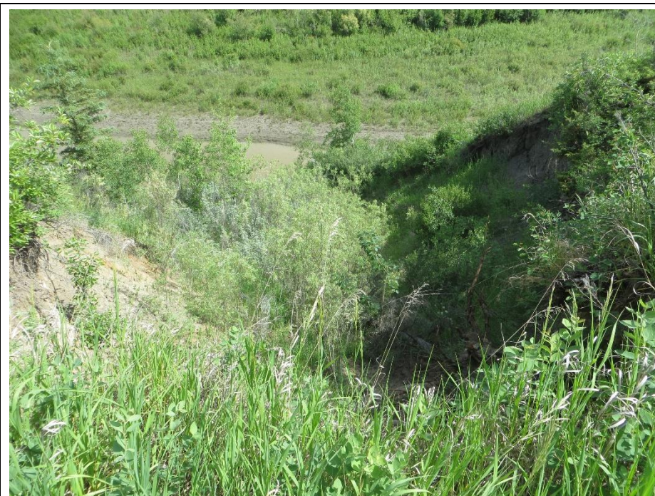
Photo 10. Looking east along the center of the backscarp of Slide 2. The backscarp is about 14 m wide along the crest of valley the slope.
