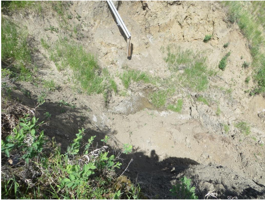
Photo 3. Looking northeast from the south side of Slide 1 down into the slide bowl. Some slow seepage and recent mud flow can be observed in the base of the bowl.
