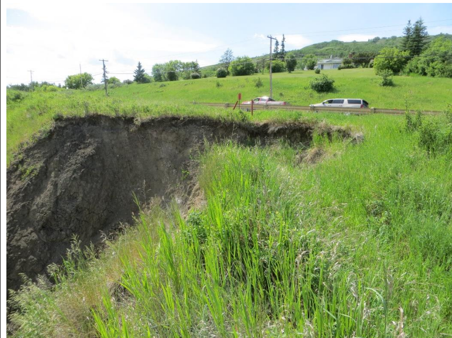
Photo 6. Looking southwest from the north side of Slide 1. The upper layer above the till surface is actively retrogressing towards Hwy 684:02.
