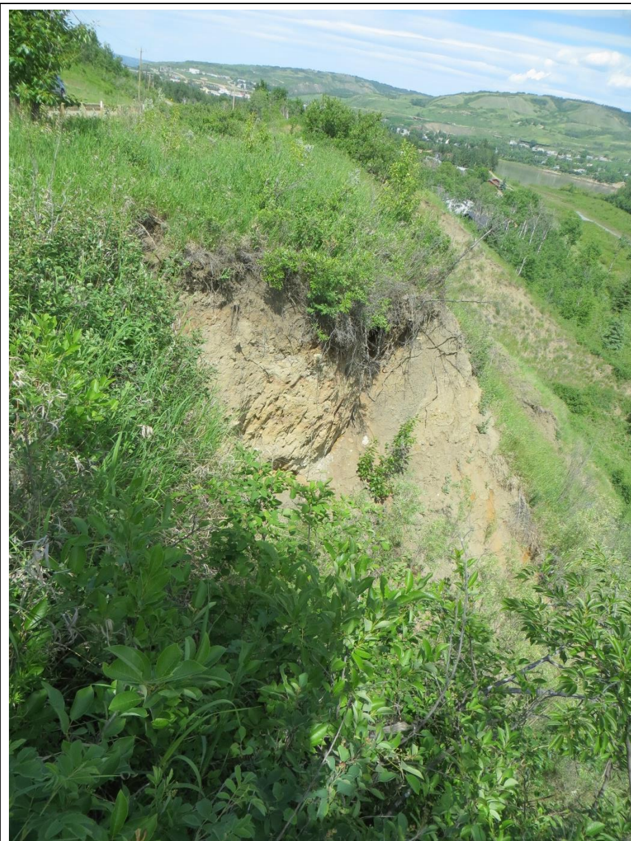
Photo 7. Looking northeast from the center of Slide 2.
