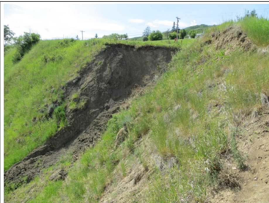
Photo 5. Looking southwest from the north side of Slide 1. The upper layer above the till surface is actively retrogressing.
