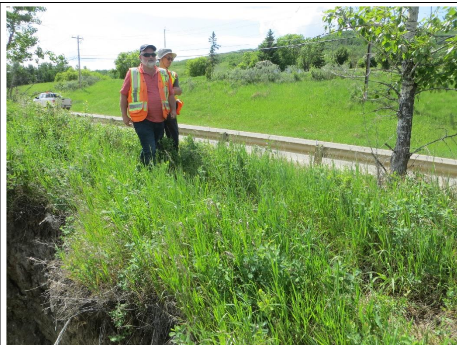
Photo 8. Looking southwest from the north side of Slide 2. The backscarp is currently at 7.5 m from the guardrail along Hwy 684:02.
