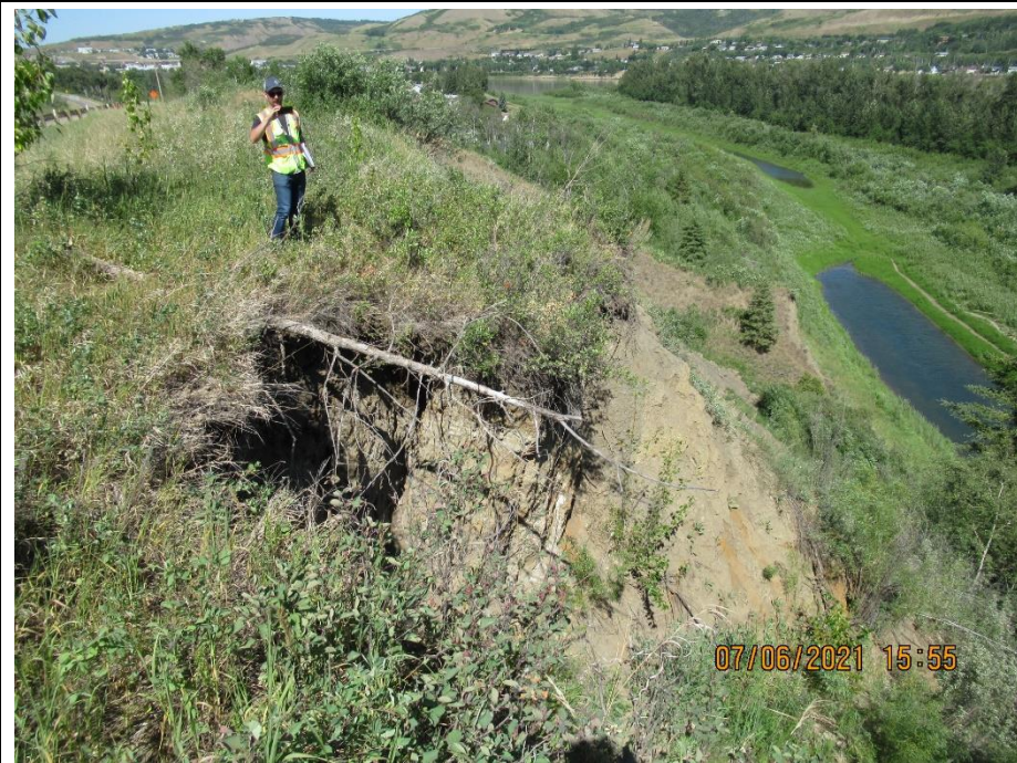
Photo 6. Looking northeast from the south flank of Slide 2.
