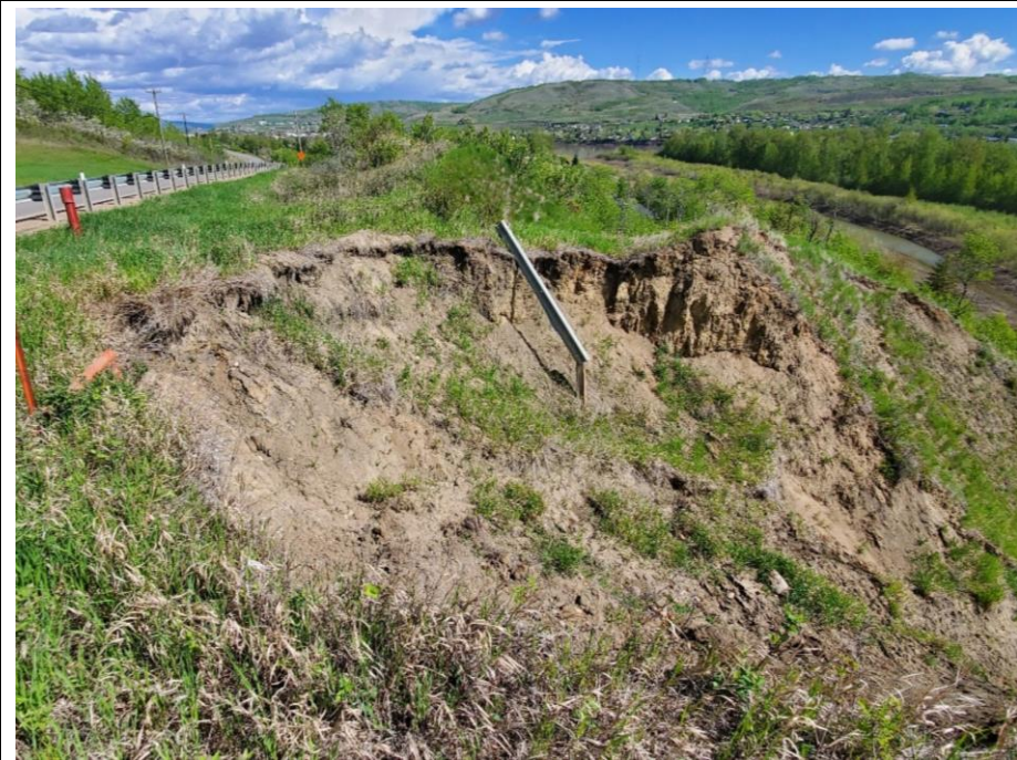
Photo 2. Looking northeast from the south side of the main scarp of Slide 1. No major retrogression was observed on the north flank relative to the 2021 condition.
