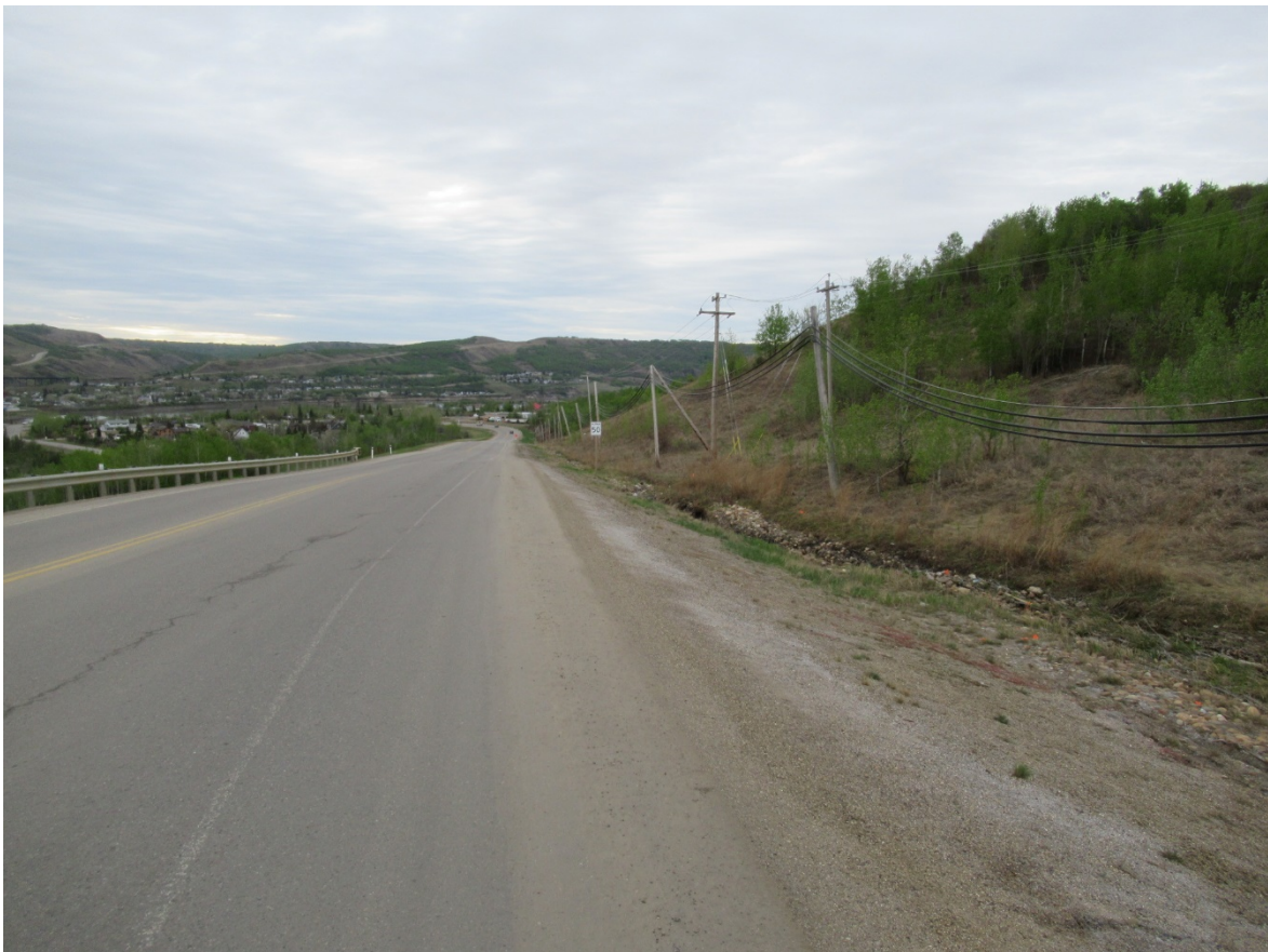
Photo 16: Looking southeast at continuation of crack from Photo 15.
