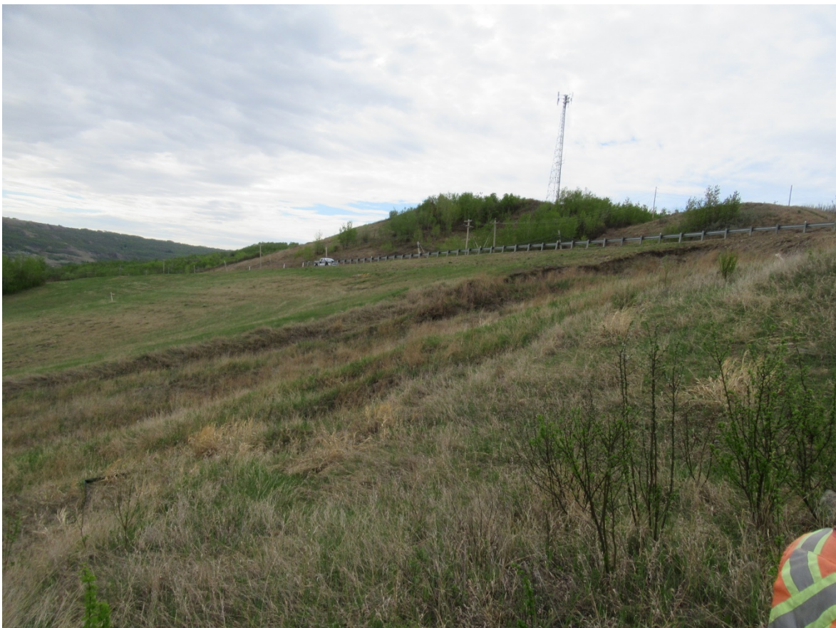
Photo 8: Looking south at backscarp of the Shop Slide below 99 Avenue intersection.
