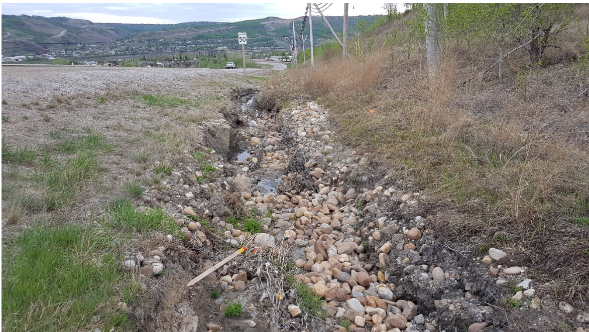
Photo 14: Looking southeast at the scour below gabion mattress in southeast ditch of Hwy 2 off-ramp.
