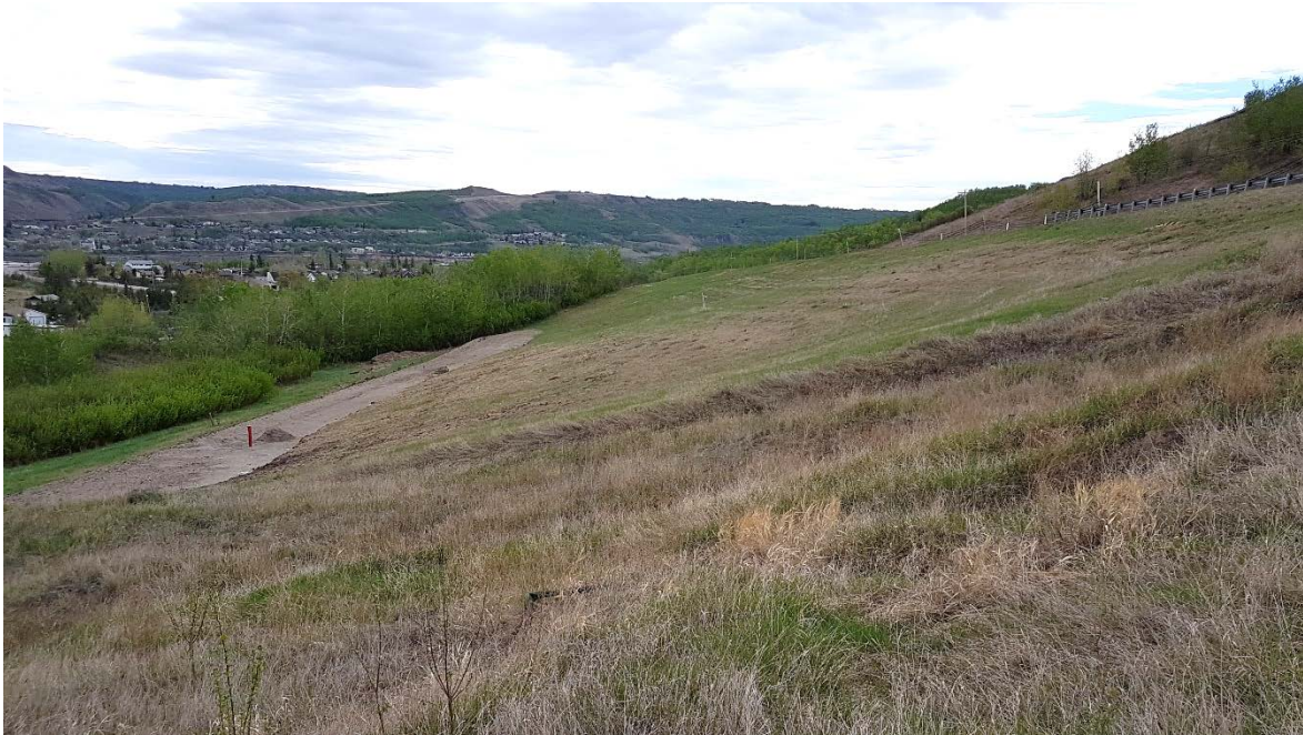
Photo 9: Looking southeast at the debris fan of the Shop Slide. New SI19-5 can be seen at left hand edge of photo on bench constructed for installation.
