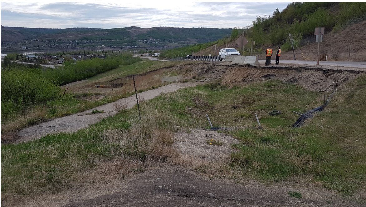
Photo 2: Looking southeast towards the backscarp along the east shoulder of the Hwy 2 off-ramp.
