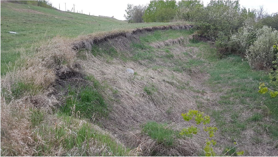
Photo 23: Looking northwest along the backscarp of the landslide downslope of the Hwy 2 off-ramp (below SP09-11).
