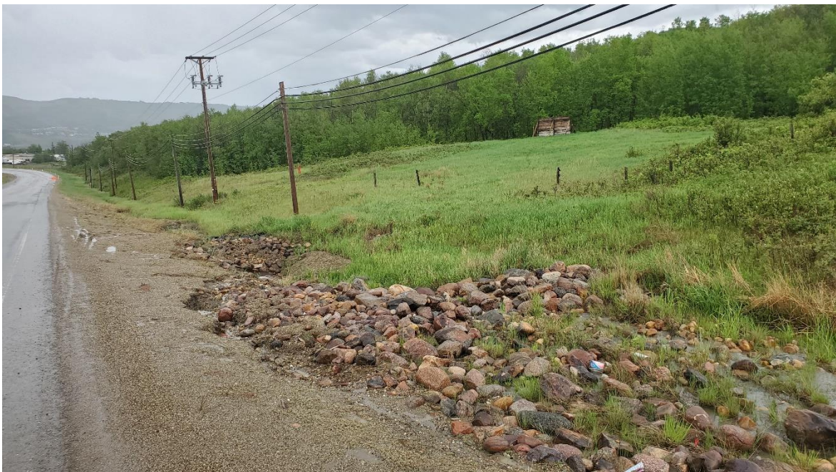
Photo 20: Looking south at riprap pile in ditch north of 500 mm SWSP centerline culvert inlet.
