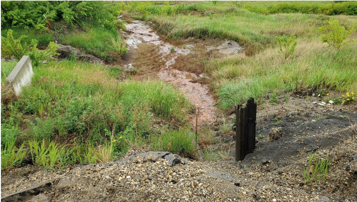
Photo 5: Looking east at seepage from gravel layer in the Hwy 2 off-ramp sideslope draining onto the geomembrane lining.
