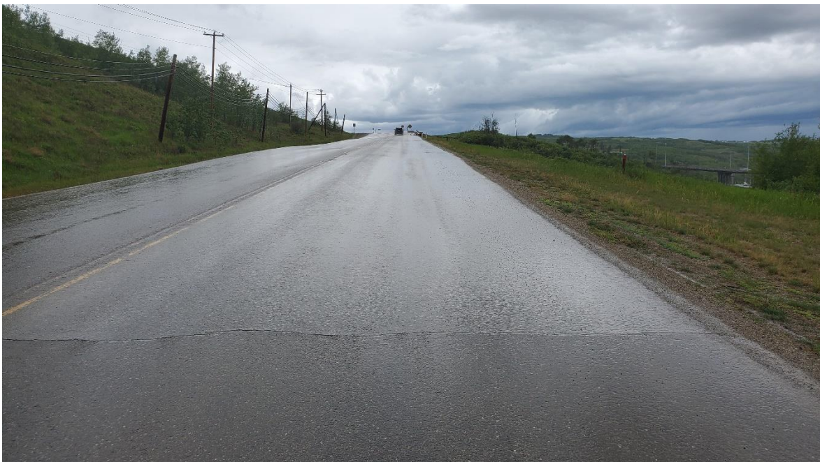
Photo 18: Looking northwest at previous scarp crack faintly visible in NBL through 2016 patch.
