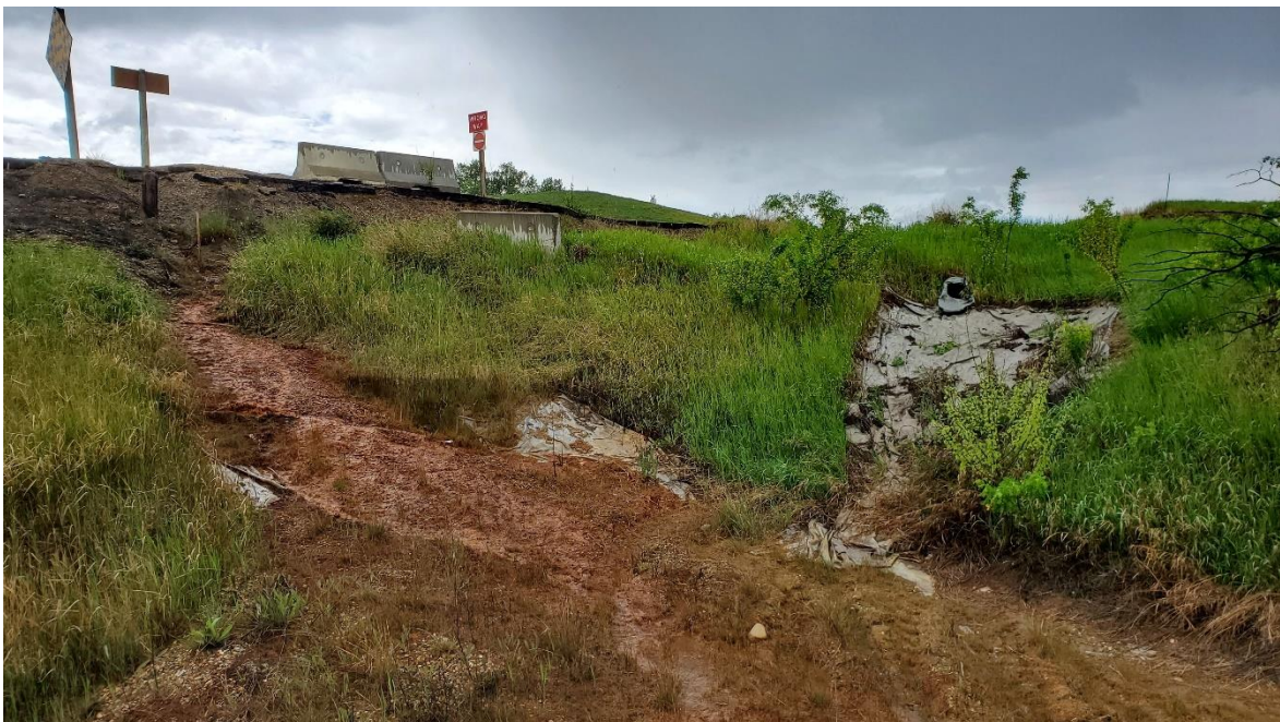
Photo 4: Looking west at springs flowing from the embankment below the Hwy 2 off-ramp at 99 Avenue.
