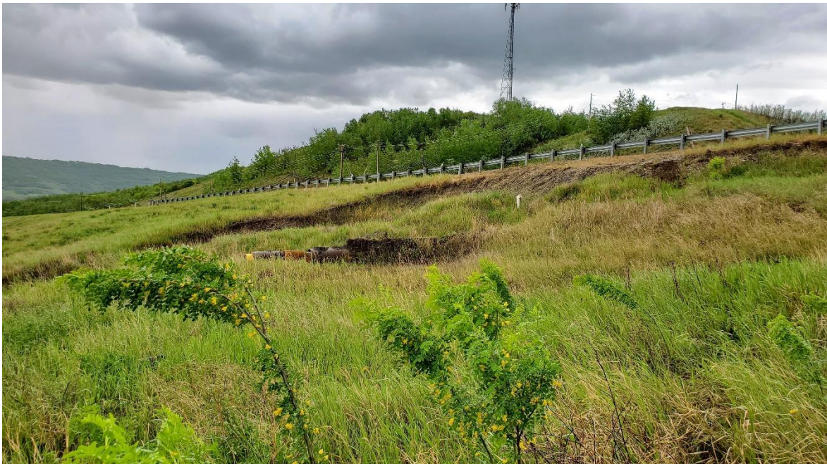
Photo 8: Looking south at backscarp of the Shop Slide below 99 Avenue intersection.
