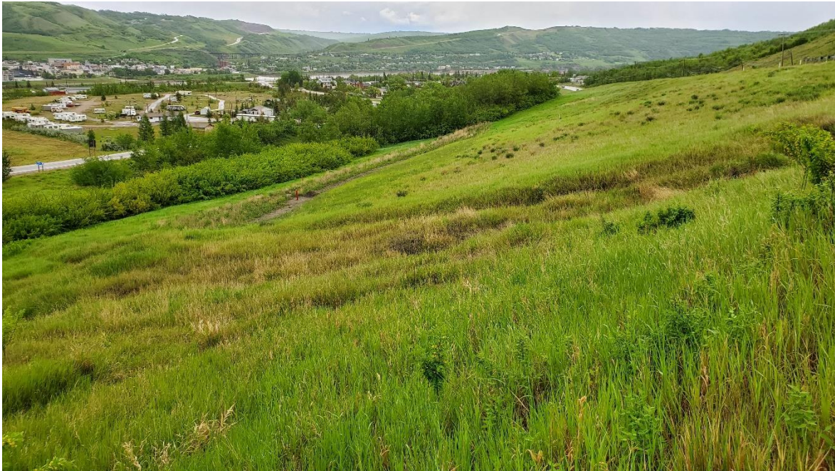
Photo 9: Looking southeast at the debris fan of the Shop Slide. New SI19-5 can be seen at left hand edge of photo on bench constructed for installation.
