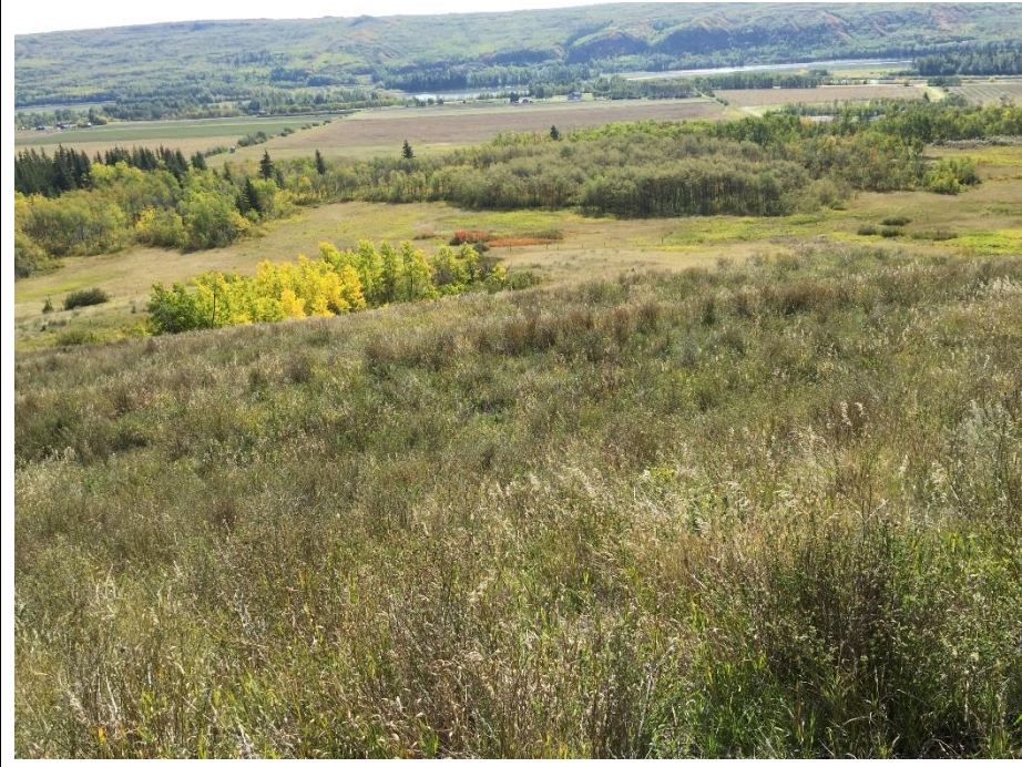
Photo 8. Looking SE from SBL ditch at toe berm constructed in 2004. No visible signs of movement or changes since last visit in June 2006.
