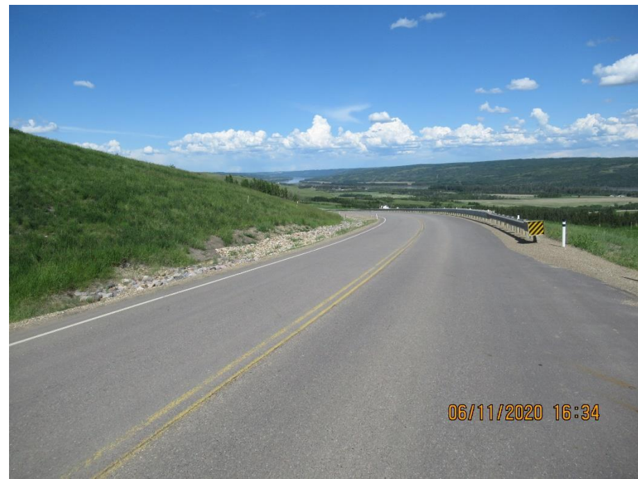
Photo 1. Looking northeast at repaired highway.
