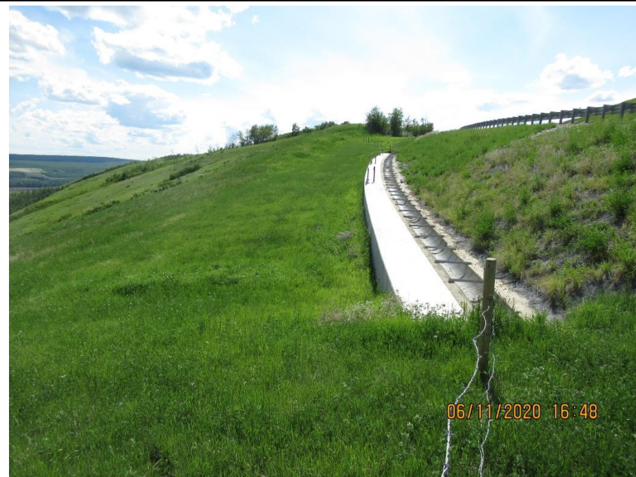
Photo 4. Looking southwest along the pile wall.
