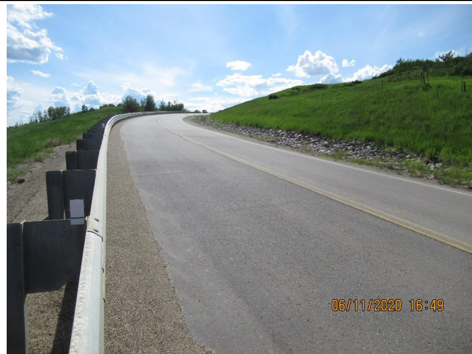
Photo 6. Looking southwest at the repaired highway.
