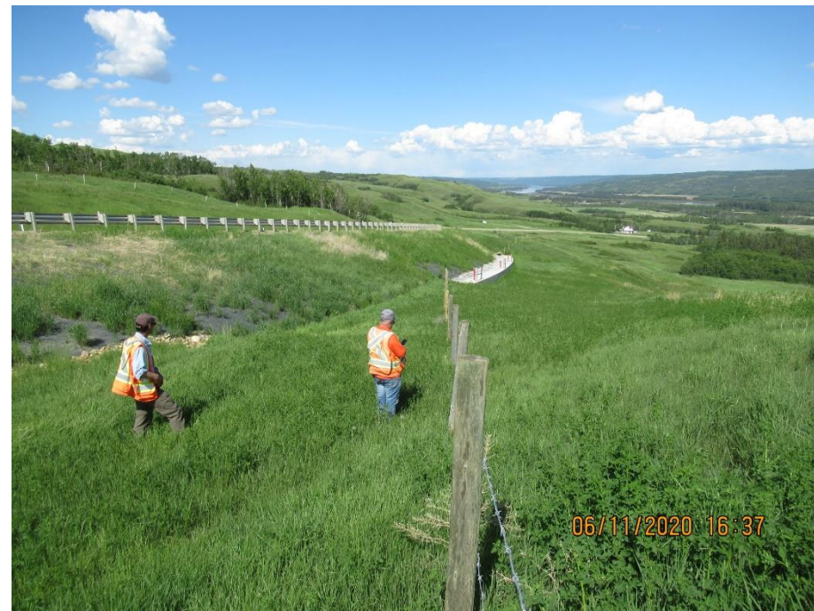
Photo 2. Looking northeast at reconstructed sideslope and pile wall.
