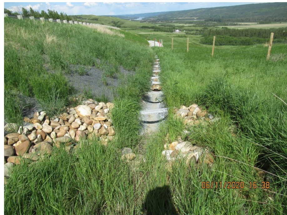
Photo 3. Looking northeast along the 1/2 culvert lined drainage south drainage ditch.
