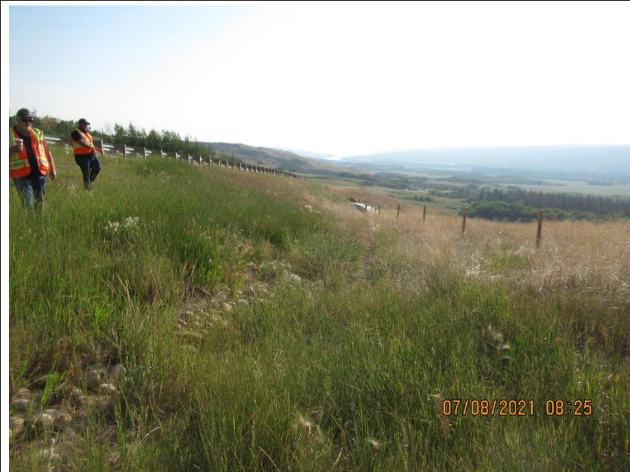
Photo 2. Looking east at landslide repair from inlet of drainage ditch
