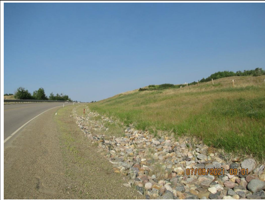
Photo 13. Looking west along upslope highway ditch
