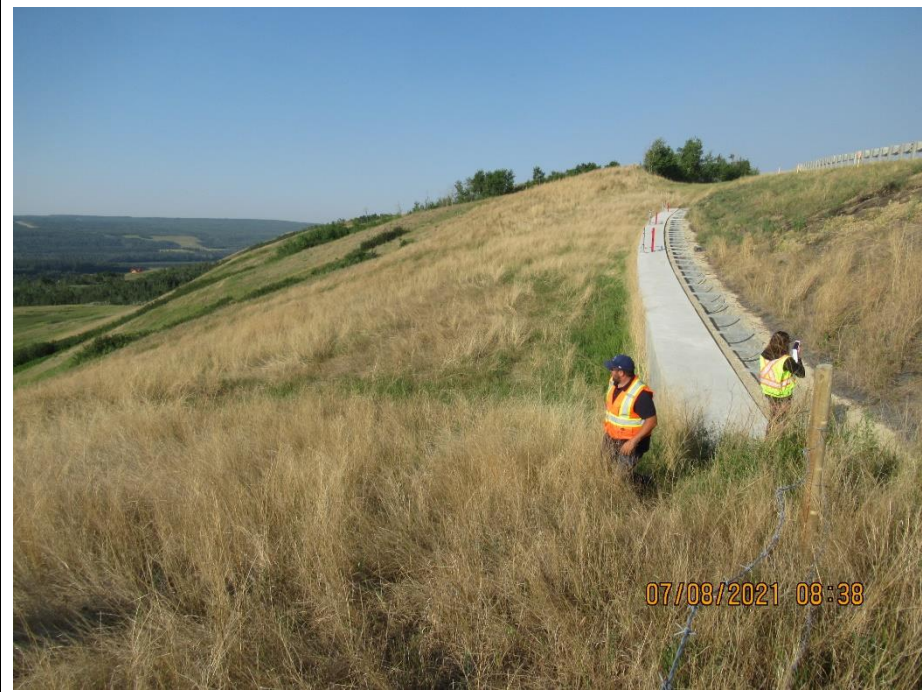
Photo 7. Looking west at slide repair fill
