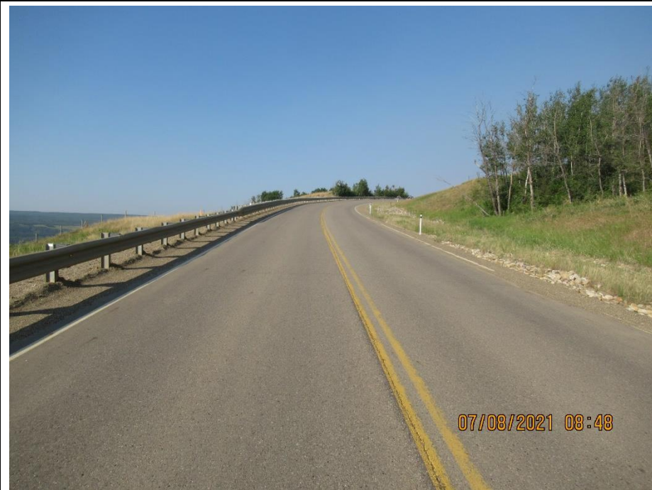
Photo 10. Looking west at slide repair along Hwy 684
