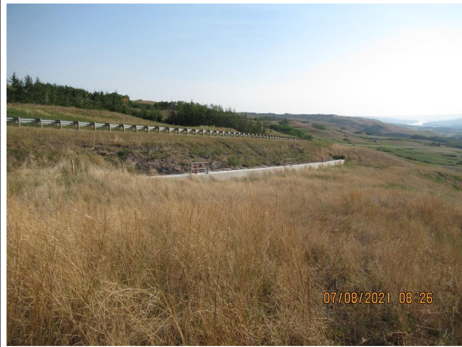
Photo 3. Looking northeast at the pile wall
