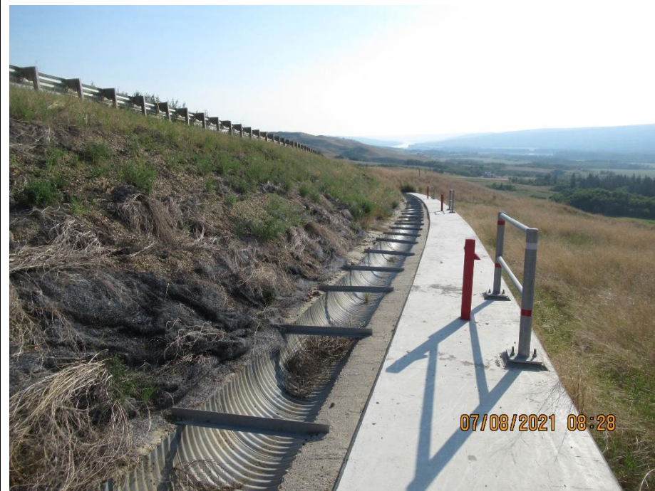
Photo 5. Looking east along the drainage trough and pile wall
