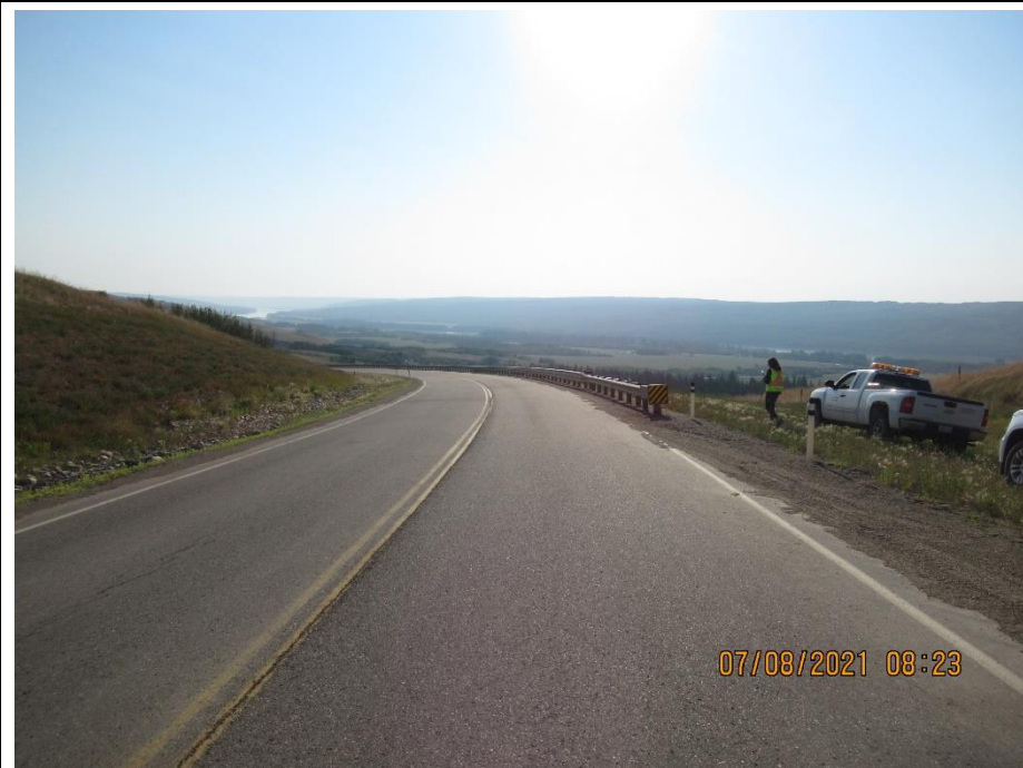
Photo 1. Looking east along Hwy 684 at landslide repair
