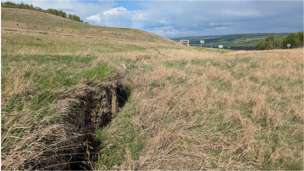
Photo 3: Looking southeast along the rest of the main tension crack at the highway sideslope.
