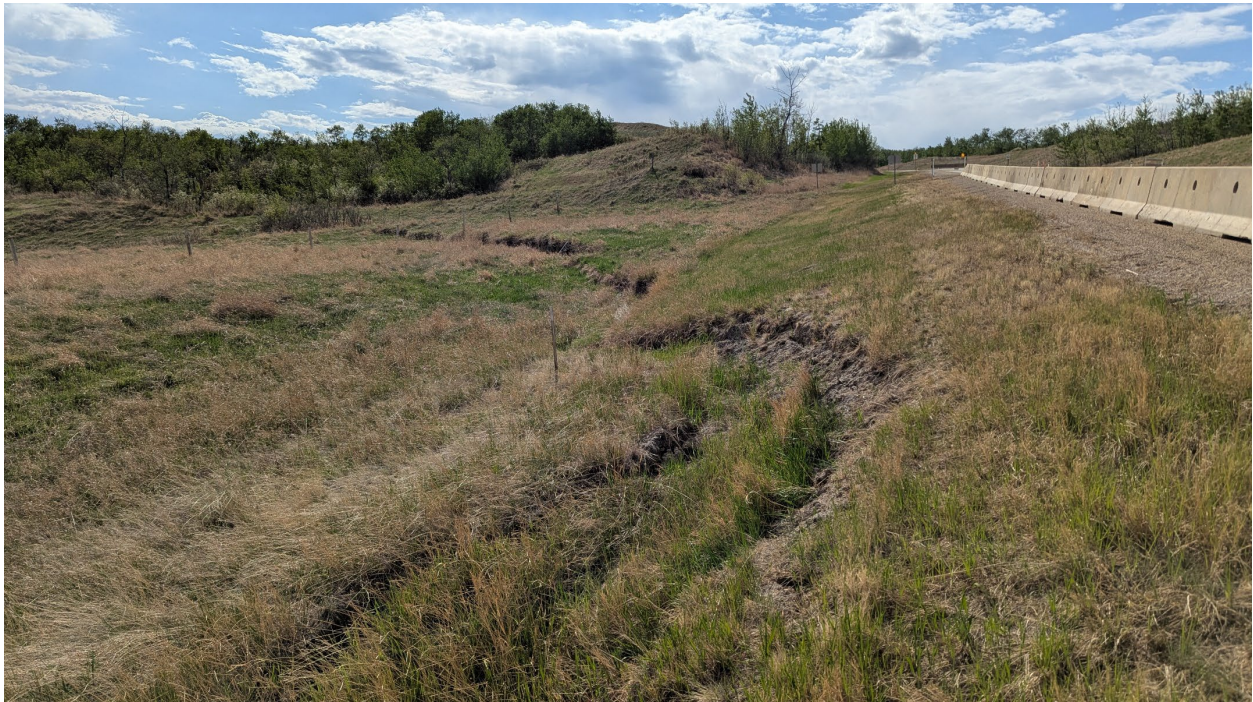
Photo 2: Looking southwest along main tension crack at the highway sideslope with measuring transect stakes in foreground.
