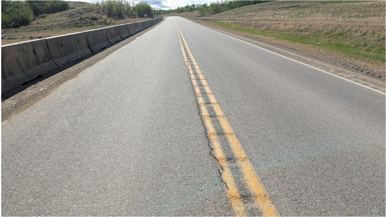
Photo 1: Looking west along as-yet uncracked highway surface. Centerline crack may be between mats from last paving/overlay.
