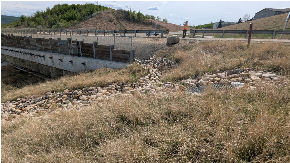
Photo 5: Looking south at NW end of wall just below SI11-01 which continues to move even after construction is completed.
