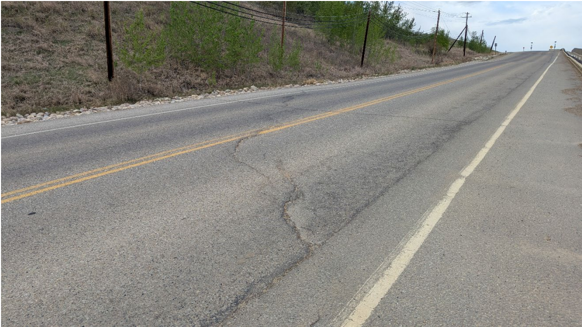
Photo 15: Looking west at the historical deep-seated crack location at the SE end of the pile wall. There was no significant change from 2024.
