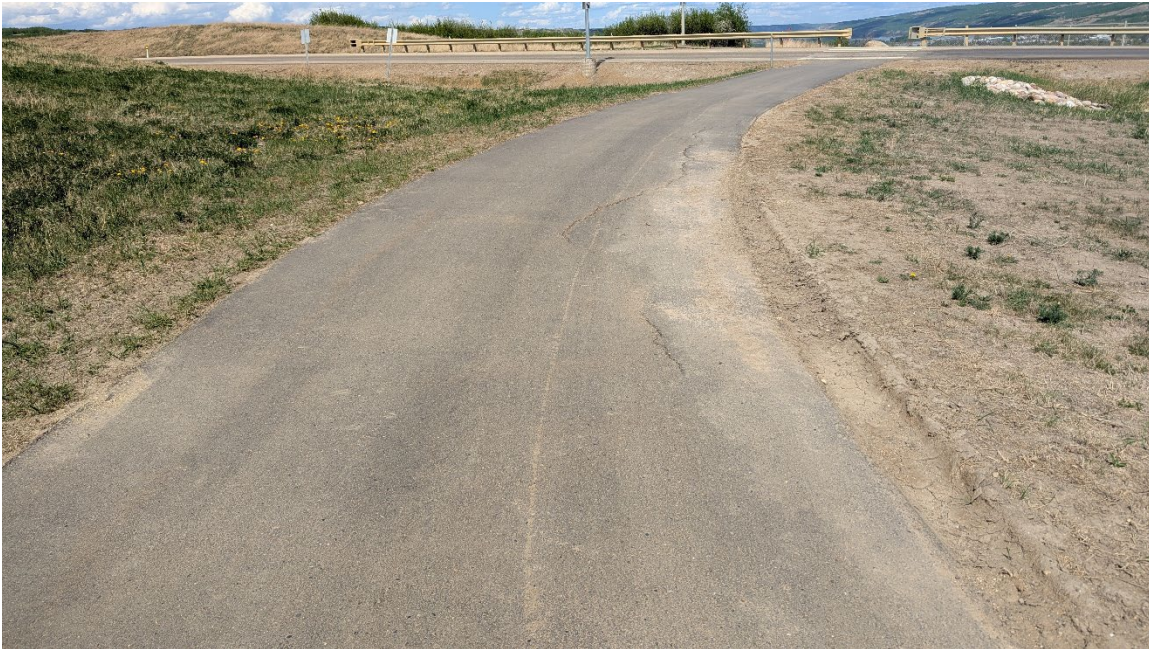
Photo 1B: Looking north at crack in new pedestrian pathway.
