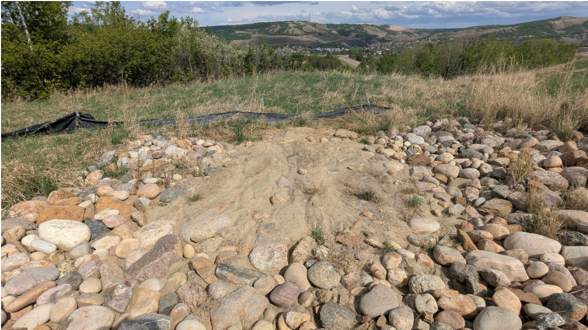
Photo 11: Looking southeast at accumulating sediment in the riprap dissipation bowl. The shallow gully forming beyond the silt fence has started to vegetate and stabilize.
