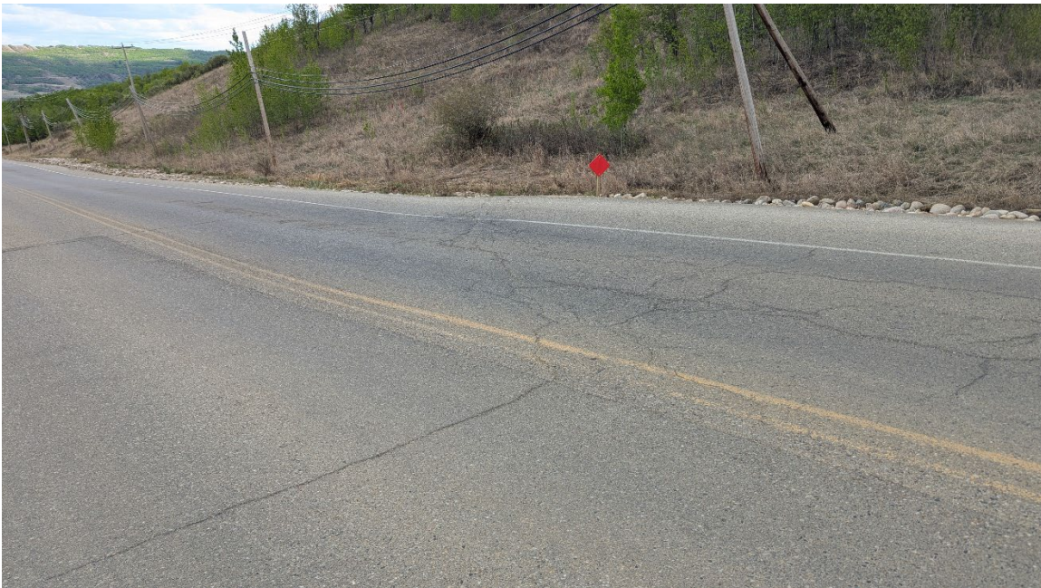
Photo 17: Looking south at the cracks coincident with the northwest flank of the deep-seated landslide.
