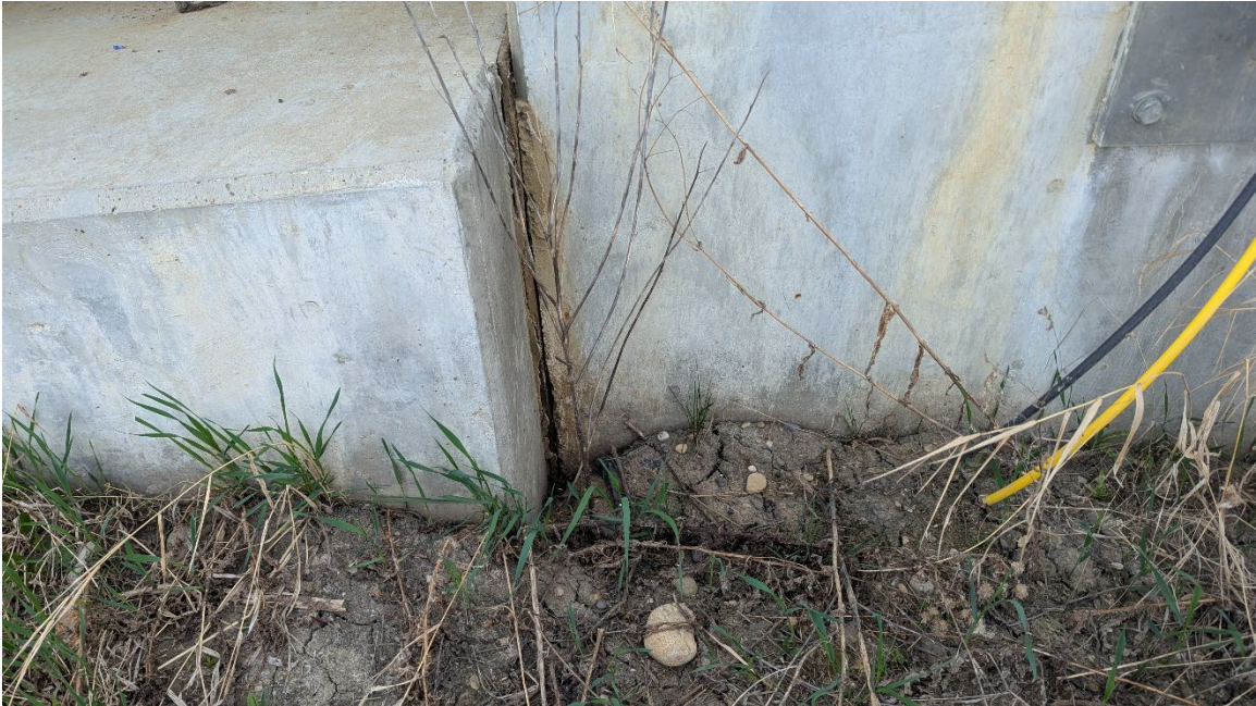
Photo 10: Small void or settlement at the junction between Wall Types 2 and 3. It hasn't gotten worse since 2024.
