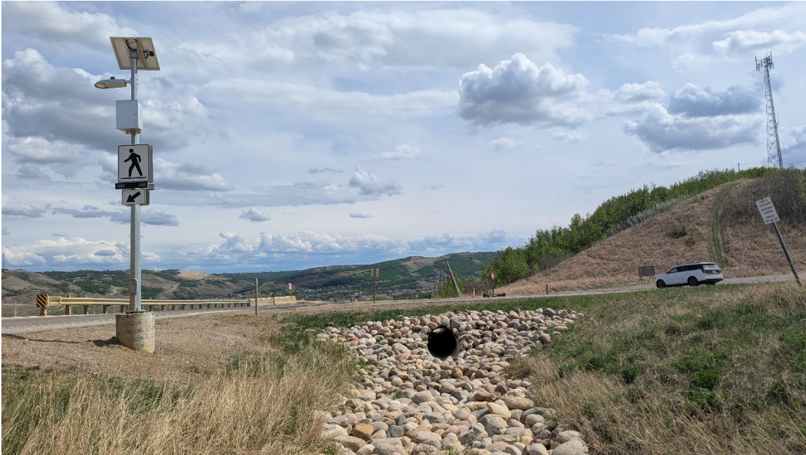
Photo 2: Looking southeast at new culvert and crossing lights installed by Town at pedestrian pathway.
