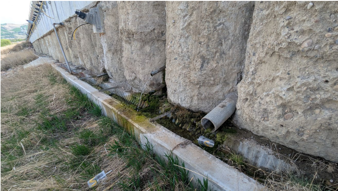
Photo 6: Accumulating sediment and moss growth around the active subdrains. Those on the far side of the apron are dry.
