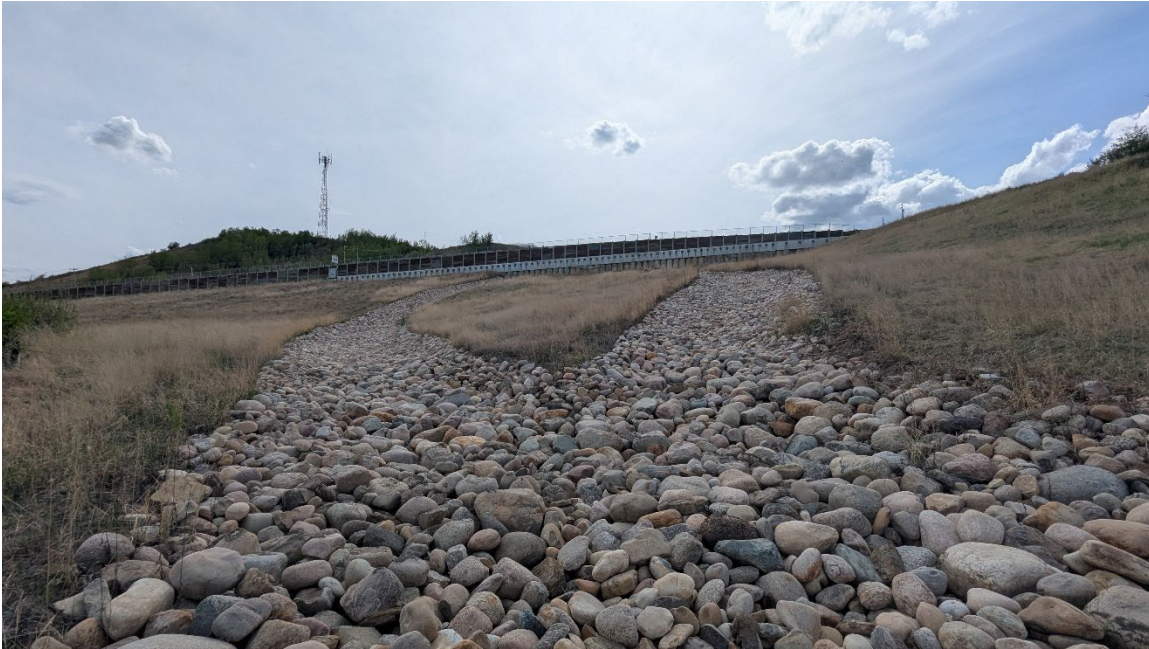
Photo 8: Looking southwest back up at the wall along the regraded slope and riprap drainage channels.
