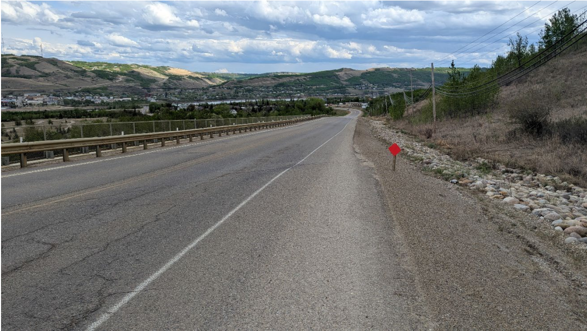
Photo 16: Looking southeast at the dips in the roadway surface and the shallow gully forming at the top of the riprap in the right ditch.
