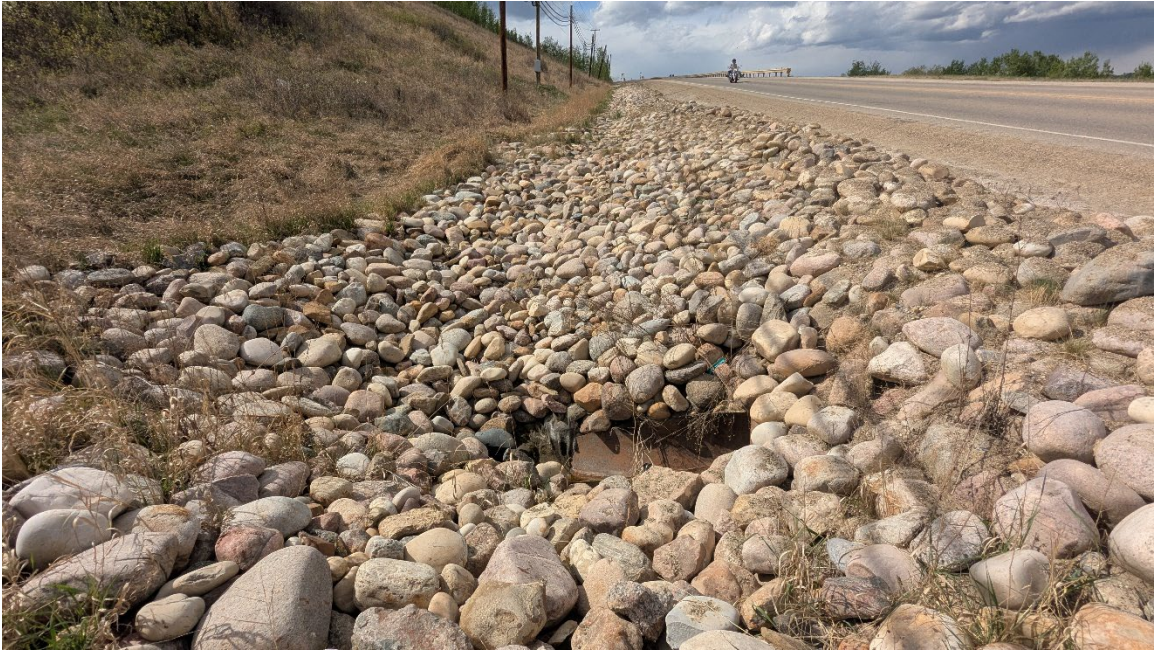
Photo 14: Looking northwest along the re-lined upslope ditch where 2024 construction activity had disturbed the riprap diverting flow out of the channel.
