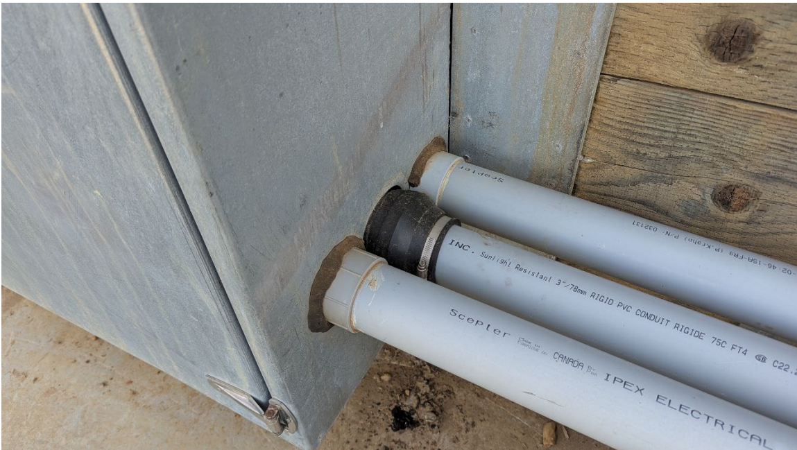
Photo 9: Thermal expansion/contraction had detached this conduit from the side of the data enclosure. It has been partially repaired with a rubber boot. More work is recommended to make this more weather-tight.
