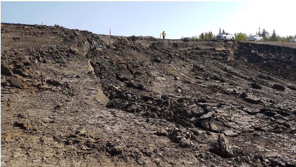
Photo 6: Looking southeast at west edge of slide.
