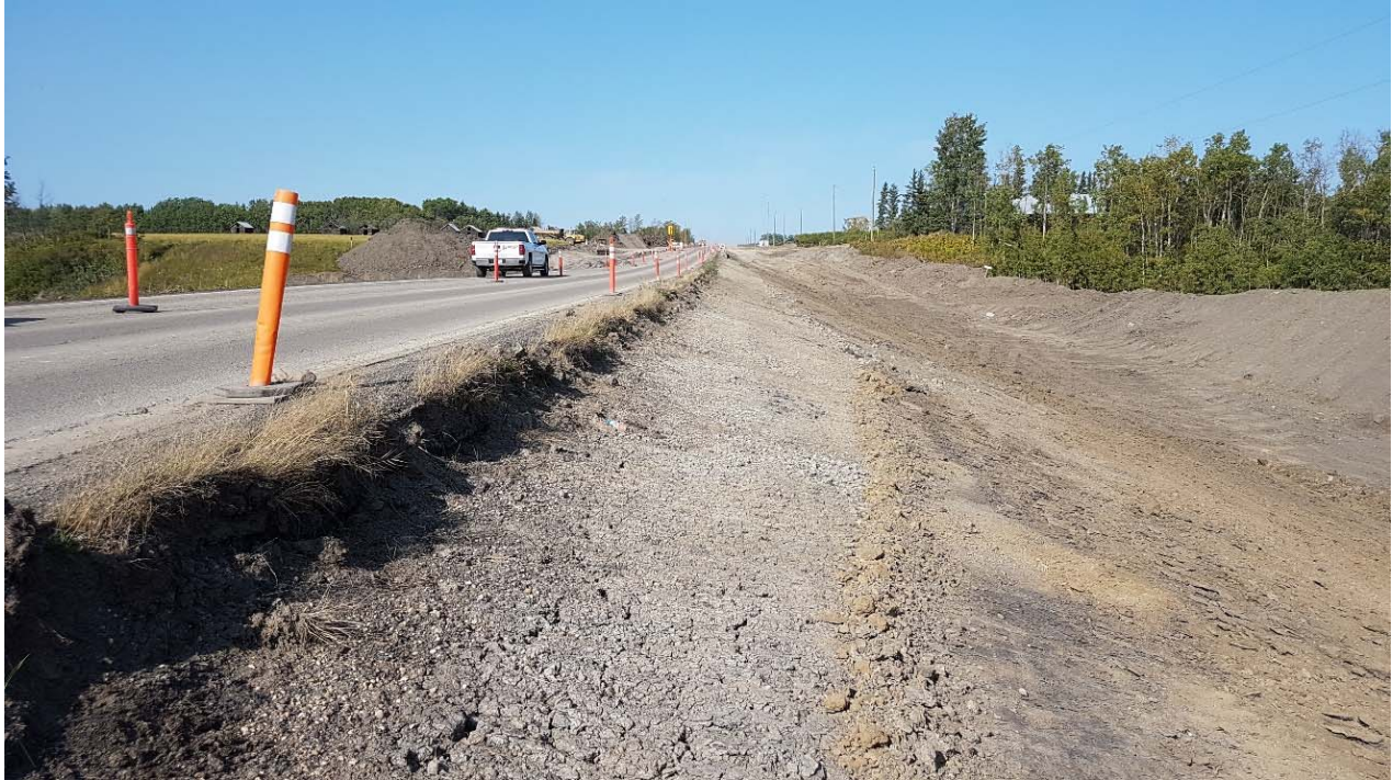
Photo 13: Looking north at stripped east sideslope above culvert extension excavation.
