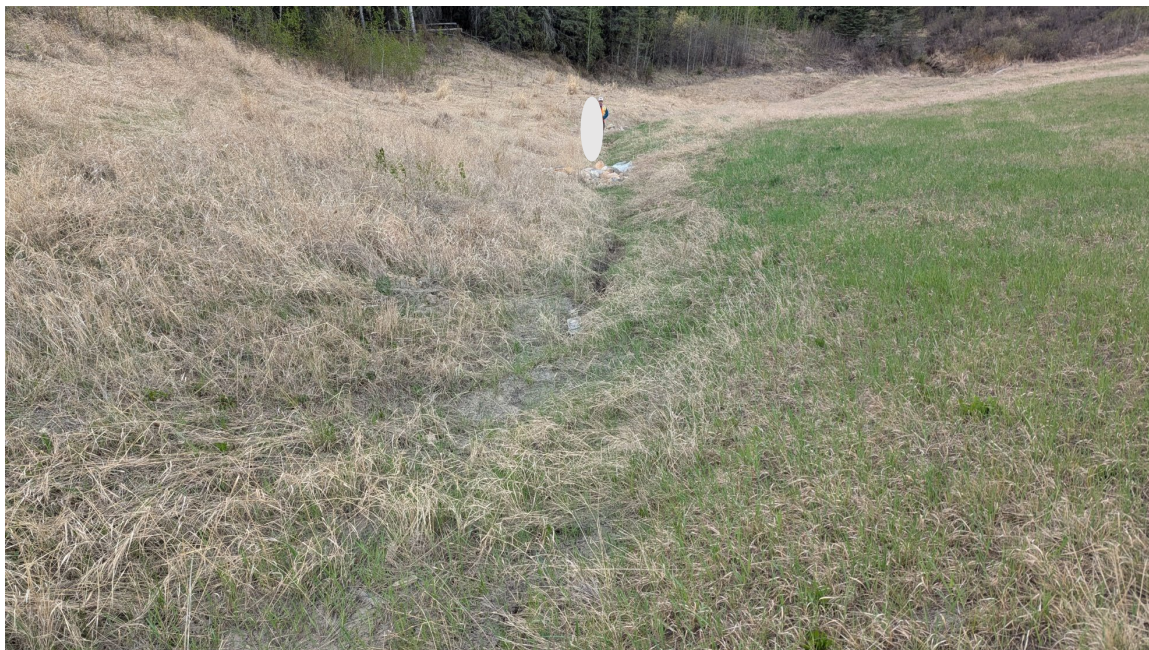
Photo 4 – Looking west at erosion gully forming in SW quadrant ditch.
