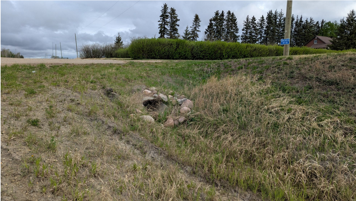
Photo 11 – Looking northeast at a gully starting to form below an approach culvert near Photo 9.
