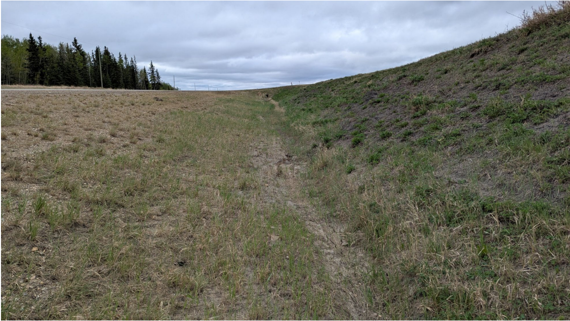
Photo 5 – Looking south at eroding west ditch. Vegetation growth has improved slightly since 2023.
