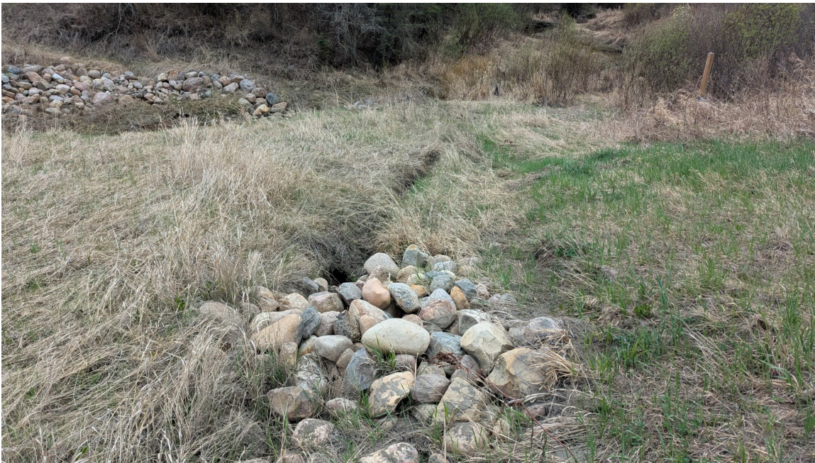
Photo 2 – Looking west at a riprap cluster and erosion gully in lower half of NW quadrant ditch.
