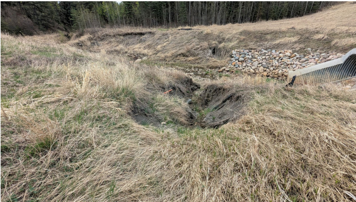
Photo 8 – Looking south at the north erosion gully (far side of Photo 6) and south erosion gully (far side of this photo) at the culvert inlet.
