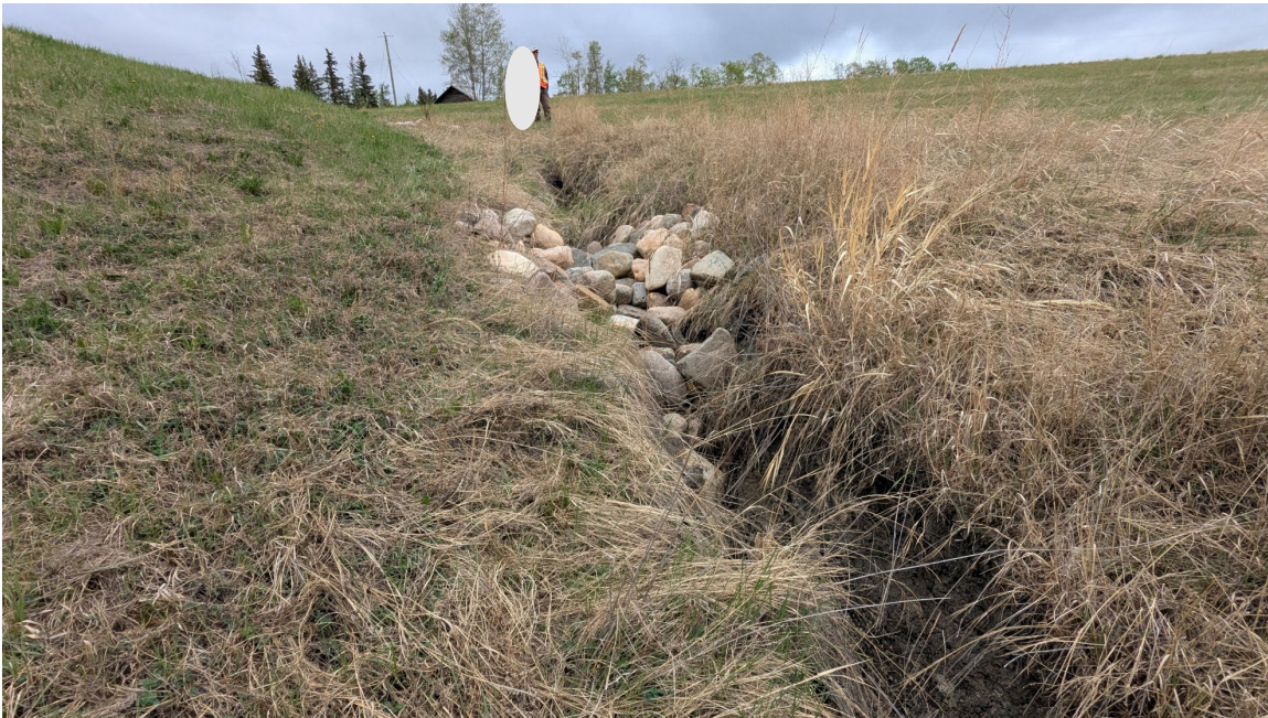
Photo 1 – Looking east at erosion at collapsed riprap clusters in NW quadrant ditch.
