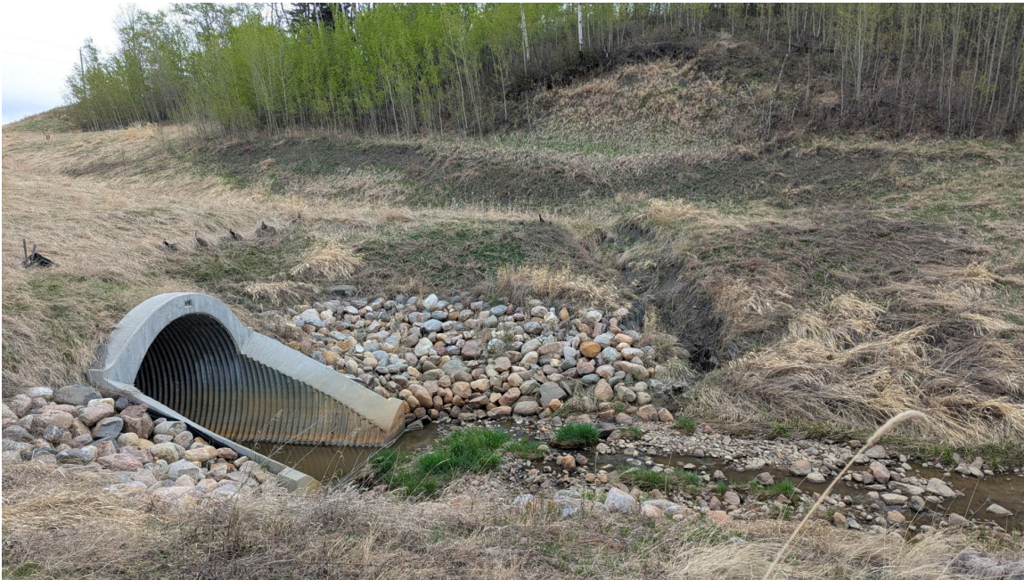
Photo 7 – Looking north at erosion gully on the north side of the culvert inlet which is starting to undermine the riprap apron.
