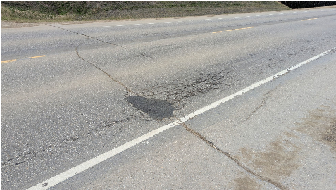
Photo 12 – Pothole and alligator cracking at north end near farm approach.
