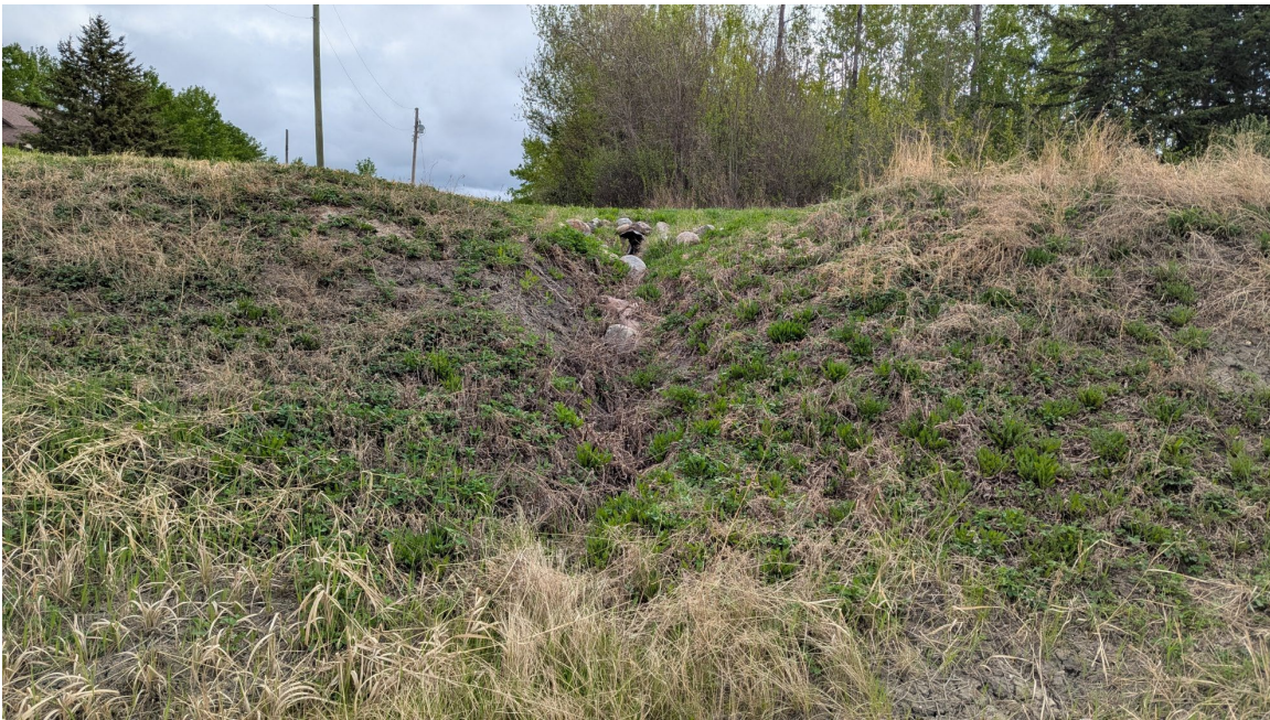
Photo 10 – Looking east at erosion gully forming below private landowner culvert on the east side of the ditch north of bridge culvert.
