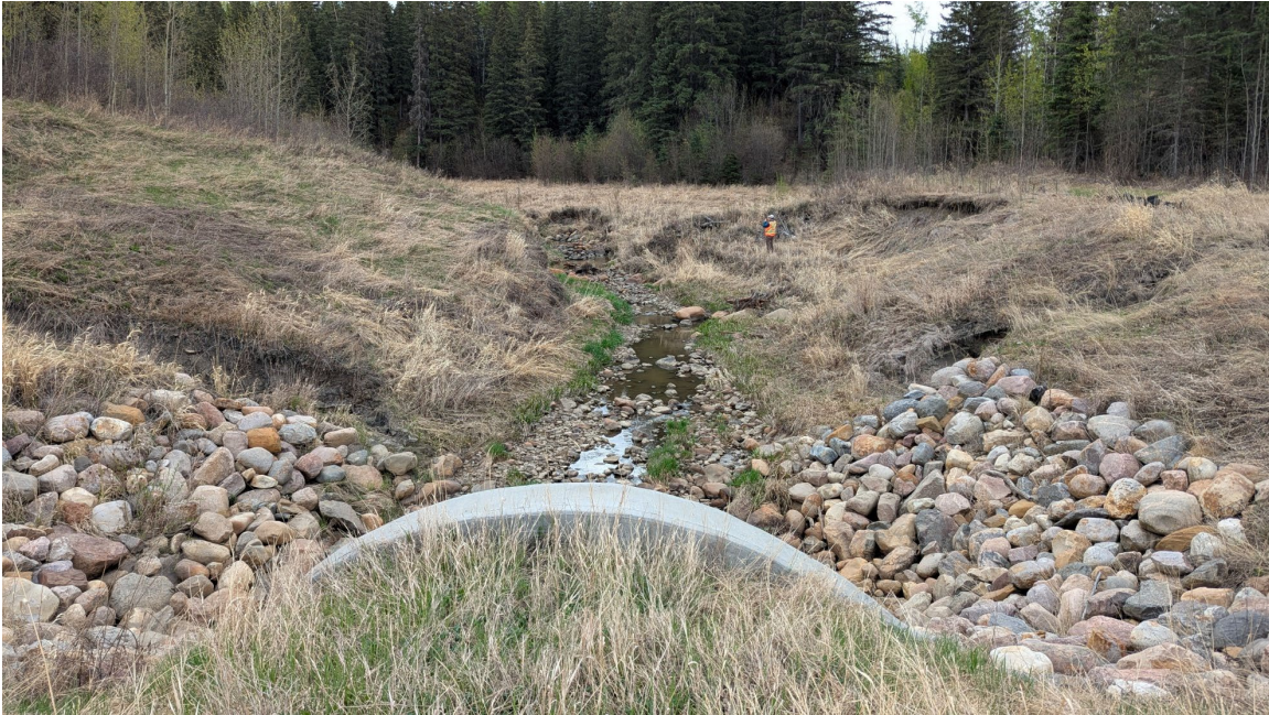
Photo 9 – Looking east at slumping forming upstream of the culvert inlet.
