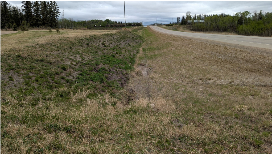
Photo 6 – Looking north at erosion gully forming below the outlet of an approach culvert in the west ditch south of the bridge culvert. Vegetation is becoming established. Also note dip in the highway over the bridge culvert.
