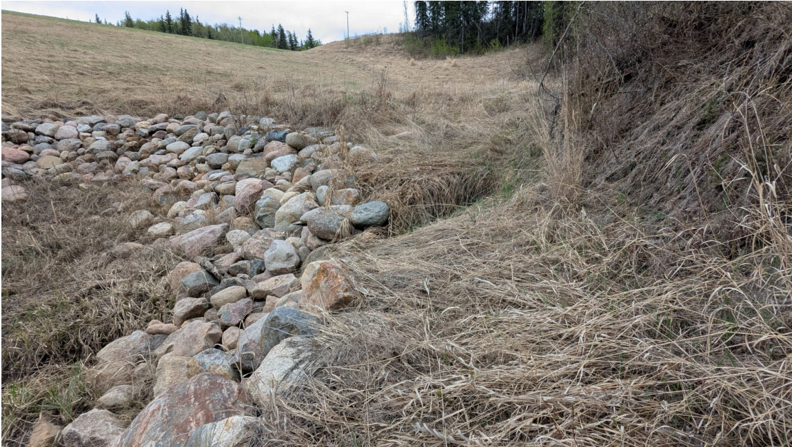
Photo 3 – Looking SE at new erosion gully cutting through the edge of the outlet riprap apron.
