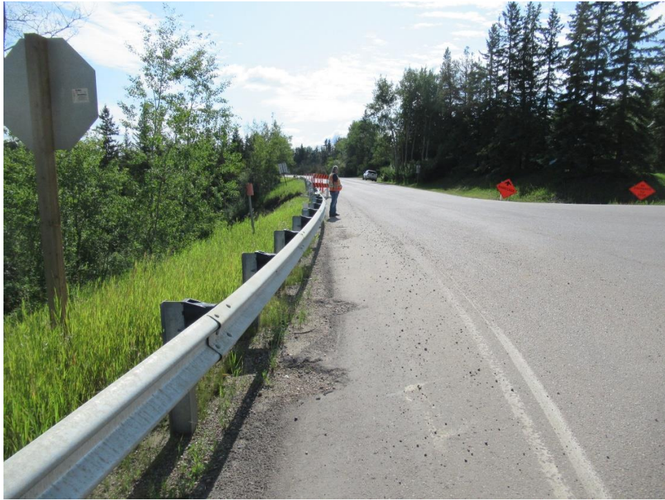
Photo 1, Looking East along Hwy. 691 toward the landslide.
