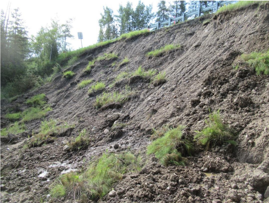
Photo 4, Seepage coming from the till in the backscarp at the slide mass.
