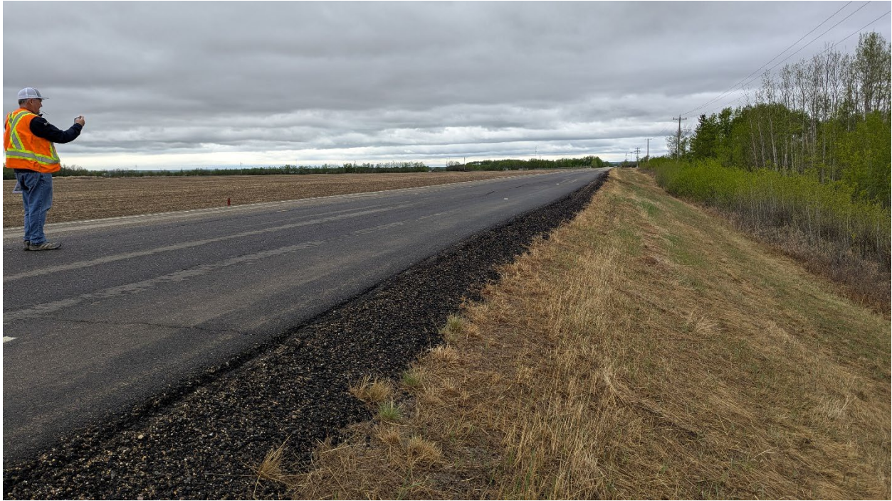
Photo 1 – Looking west over distressed area where dip is visible in the roadway surface. Note the increasing thickness of asphalt from repeated patching.
